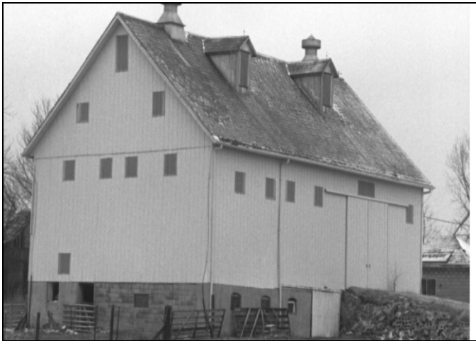
Grade C Bank Barn
