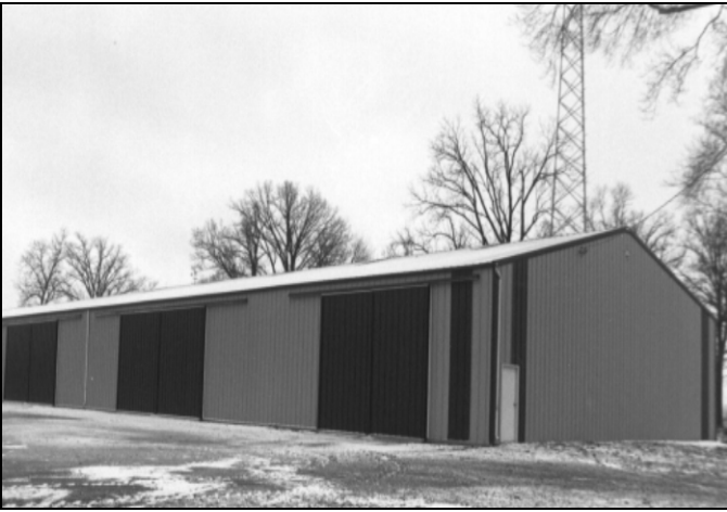
Grade C Pole Barn
