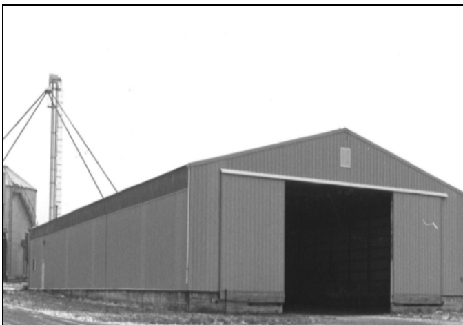
Grade C Pole Barn
