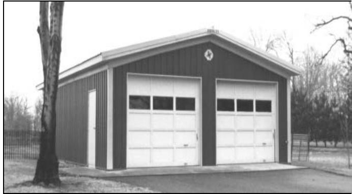
Grade C Detached Garage (Pole Type Construction)
