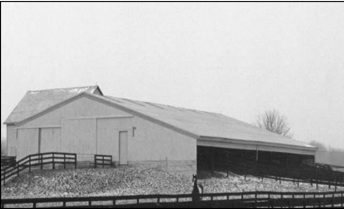
Grade C Pole Barn, One Side Open
