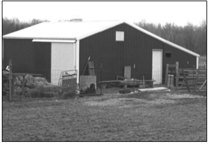
Grade C Pole Barn
