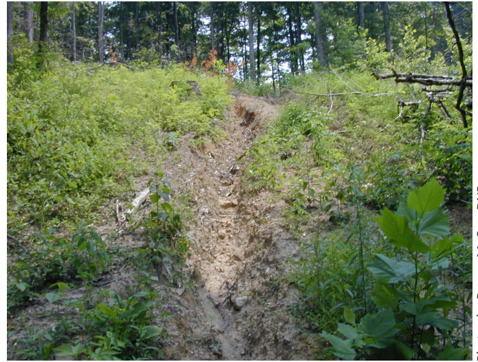
Vegetation alone is not enough to prevent erosion on skid trails with slopes. Adding water diversions to this skid trail could have prevented this gully erosion.
