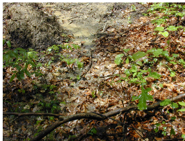
Water-bar outlet conveying runoff on to the stable forest floor.
