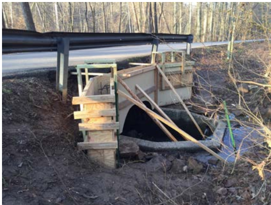
Culvert repair on the Ferdinand State Forest entrance Road
