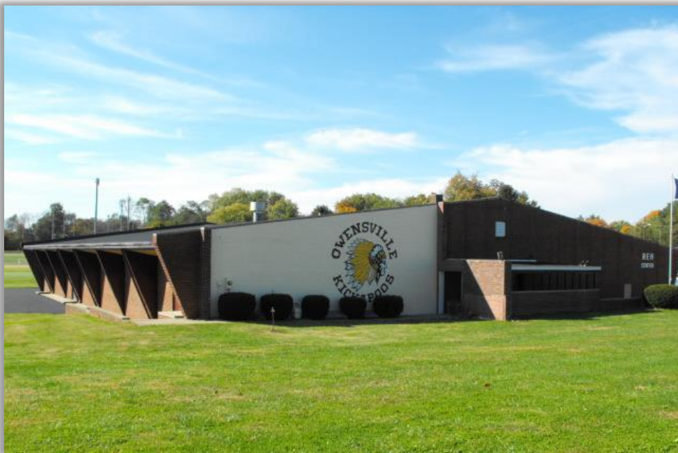
Montgomery Township Gymnasium, Owensville, the first of the sunken gyms constructed by Ralph Legeman in Indiana
