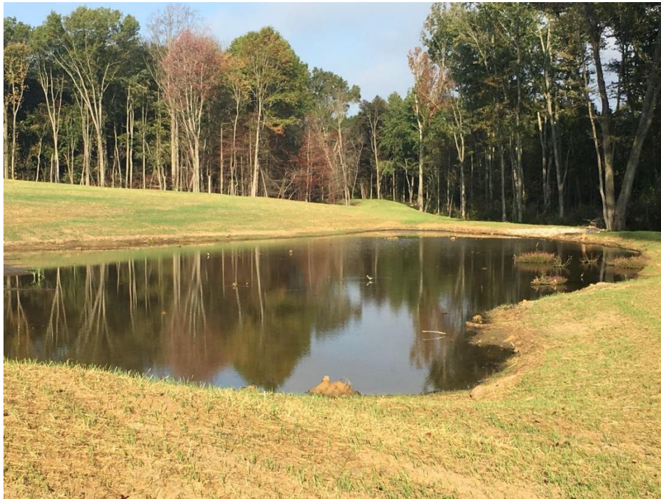
Completed reclamation of the Buttermilk Pit side of the project. The AMD-contaminated pits on this side of the project were replaced with water bodies of good water quality.
