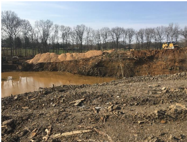
Buttermilk Pit highwall during construction.
