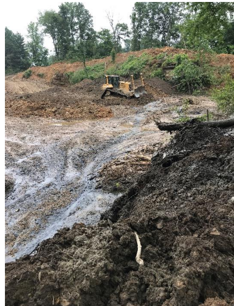
Whitney Pit highwall during construction.
