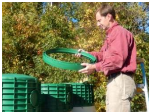
Figure 7G. Adjusting Riser Height
