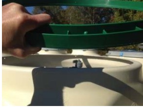
Figure 7E. Attaching Tuf-Tite 20-RTR Adaptor
