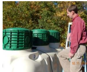
Figure 7H. Final Riser Adjustment
