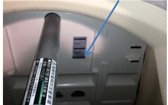
Low water line in sedimentation chamber
