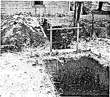
Figure 2—Tank-Hole ready for installation of wooden forms.
