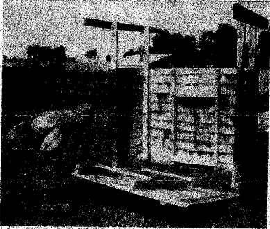
Figure 3—Assembling re-usable wooden tank forms.
