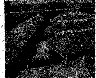
Figure 6—Effluent sewer trench and absorption trenches.
