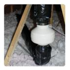
The **radon fan** is located in an unconditioned space, like an attic or outside, to prevent radon from leaking back into the home. The fan is plugged into an electrical junction box or hard wired.
