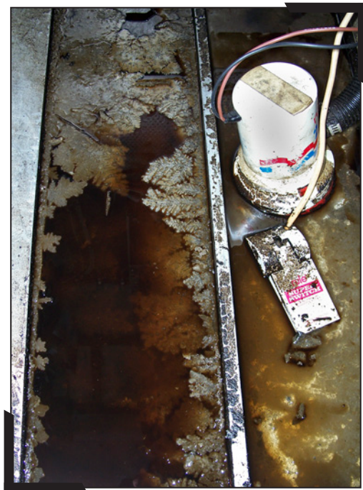
The use of a bilge sock would help prevent oil collected in the bottom of this bilge from being discharged to the lake (Photo by Joe Exl, IDNR).
