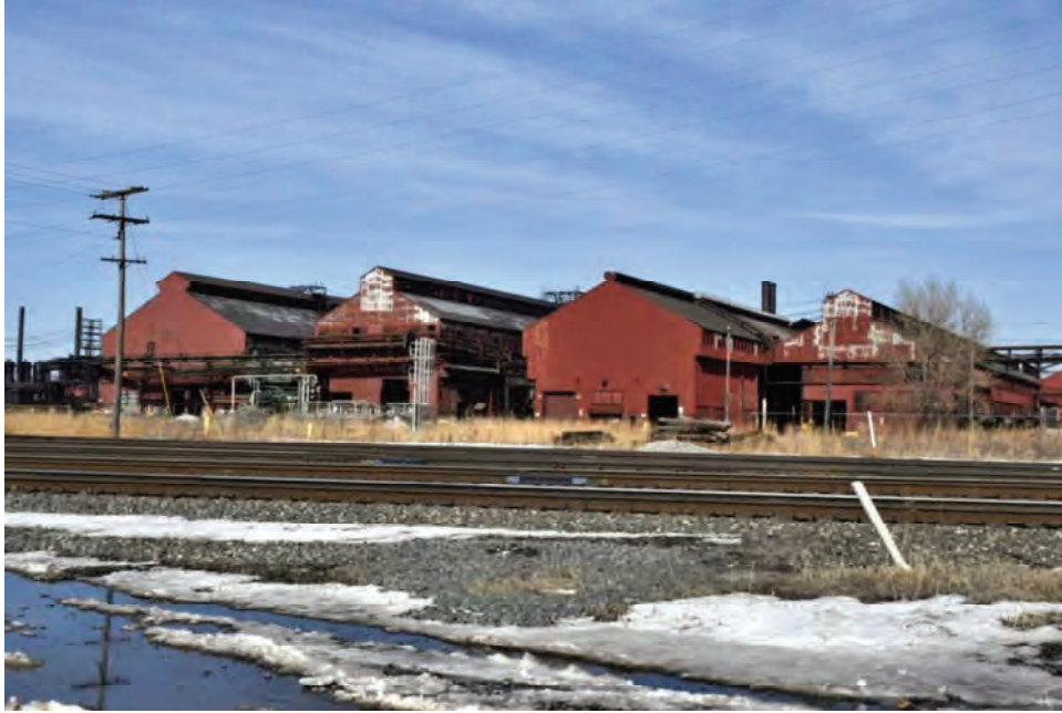
Photograph 7. Inland Steel/ArcelorMittal mill buildings. Photo taken looking north-northwest from the service road leading to the Pedestrian Bridge over the railroad.
