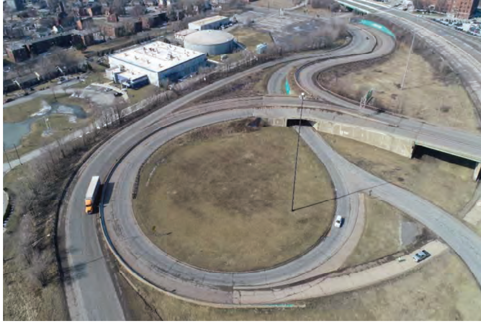
Photograph 1. Overview of the SR 912 and Michigan Avenue Interchange.
