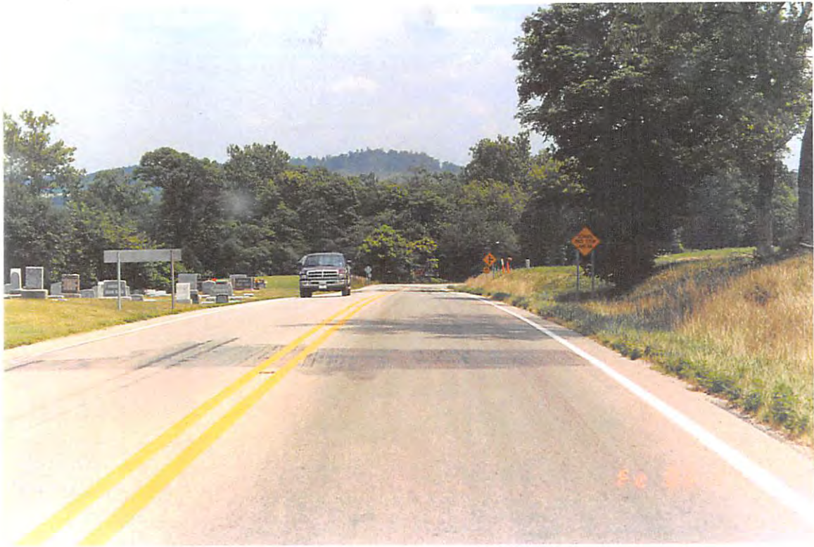
Looking east along US 150/SR 56 at location of new alignment
