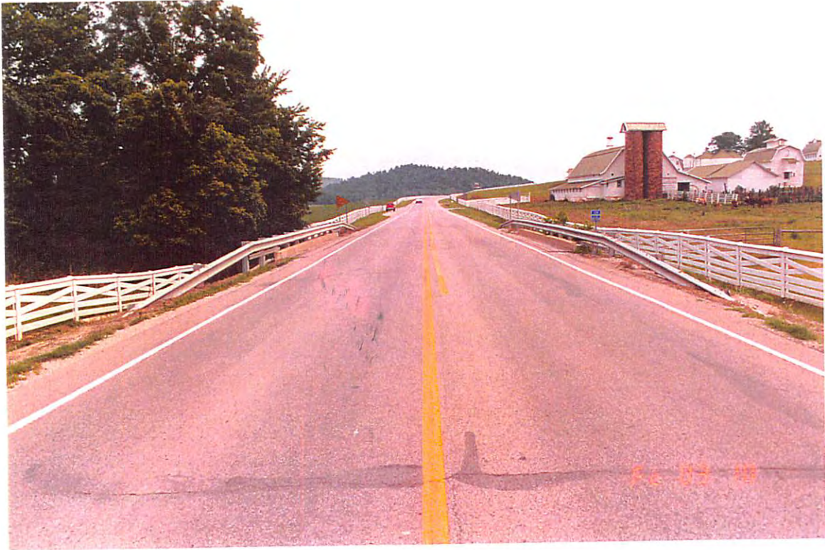
Looking east across Bridge Structure 150-59-0559
