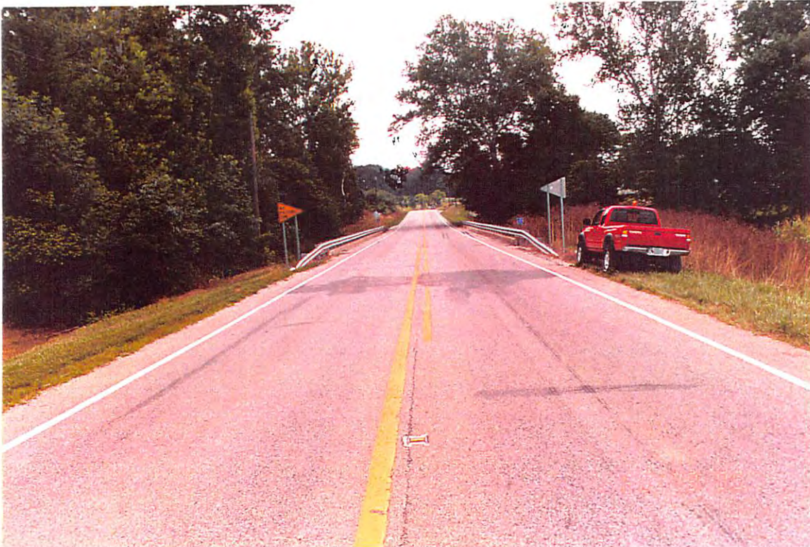
Looking east across Bridge Structure 150-59-0449 over Lick Creek
