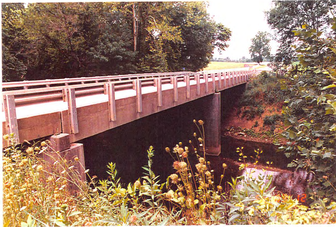
Looking southeast at Bridge Structure 150-59-5938A
