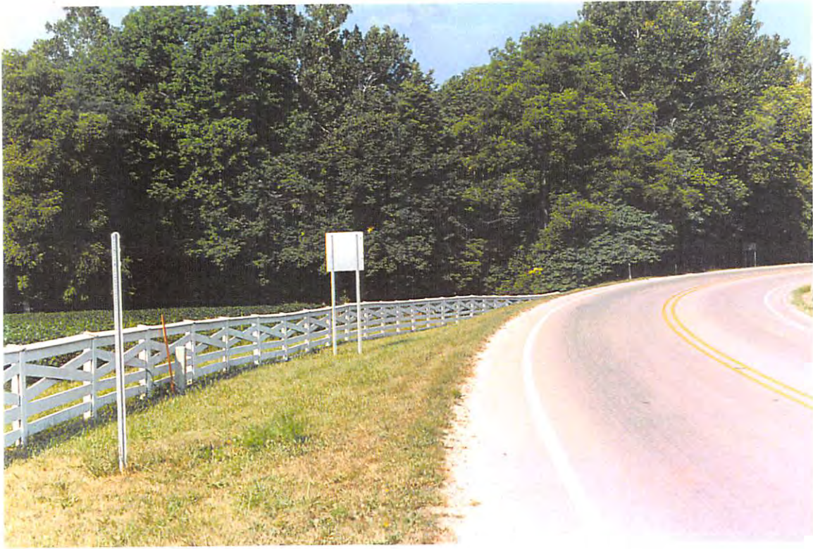
Looking west at location of where proposed alignment meets existing US 150/SR 56
