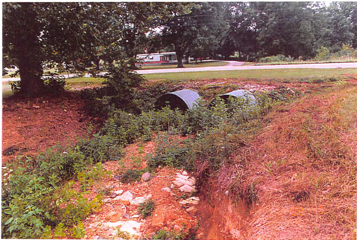
Looking south at Bridge Structure 150-59-6925
