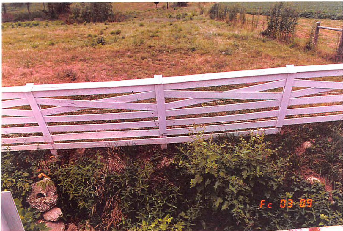
Looking downstream at branch of Lick Creek from Bridge Structure 150-59-0559
