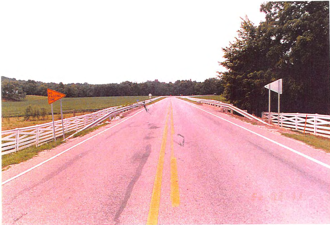
Looking west across Bridge Structure 150-59-0559
