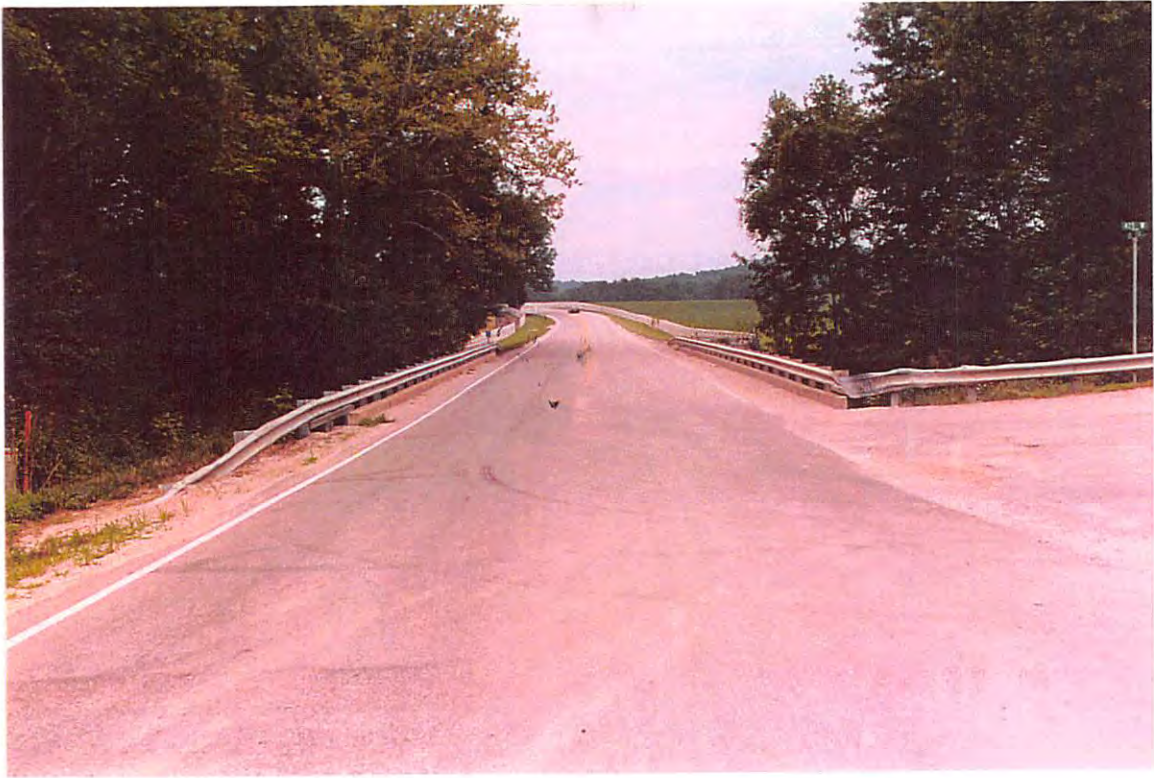
Looking west across Bridge Structure 150-59-5938A
