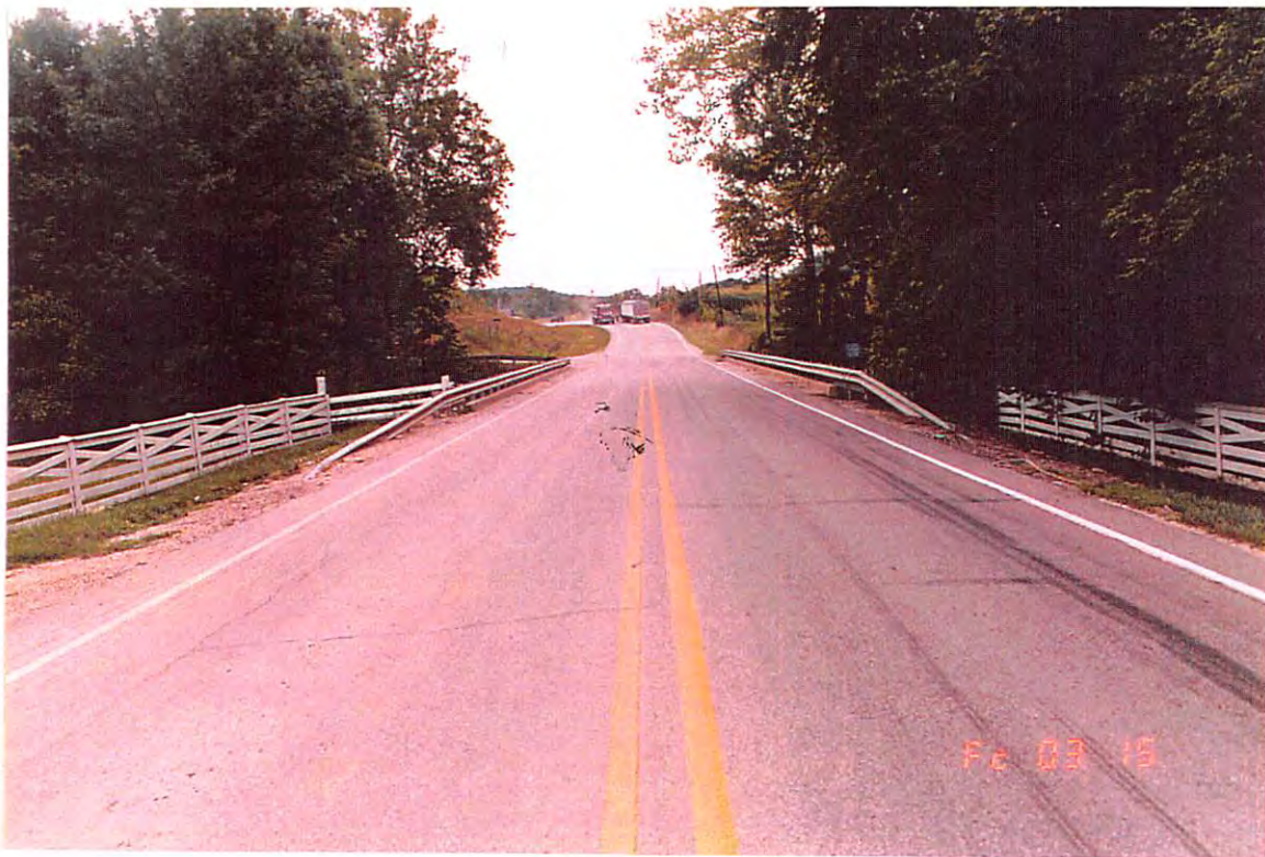
Looking east across Bridge Structure 150-59-5938A
