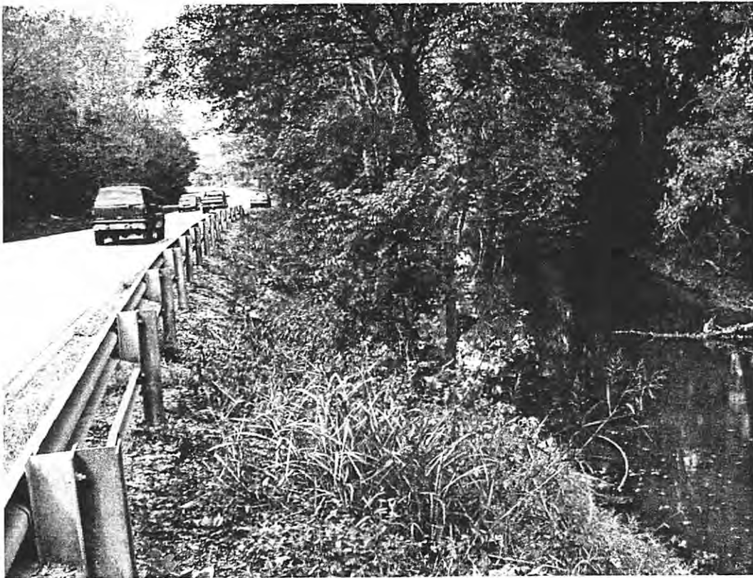
Photo 2. Highway curve near Lick Creek east of Ames Chapel
