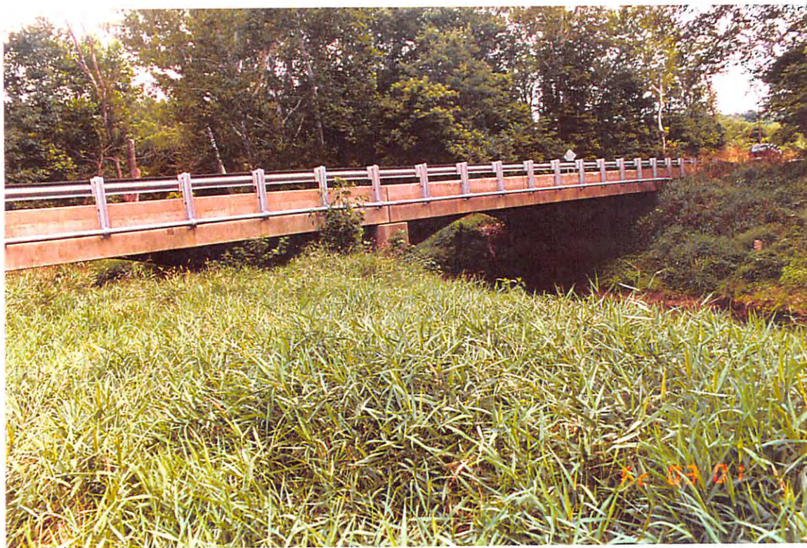
Looking northeast at Bridge Structure 150-59-5937A
