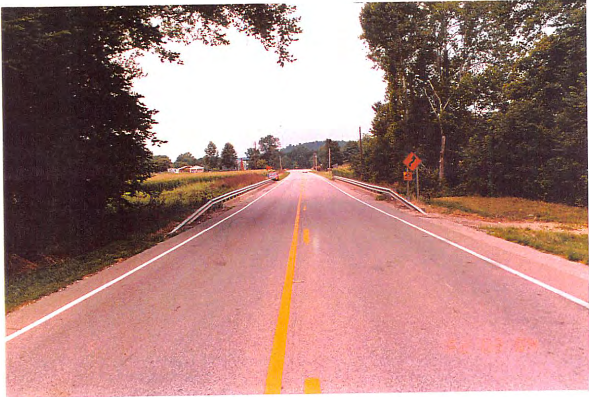
Looking west across Bridge Structure 150-59-0449 over Lick Creek
