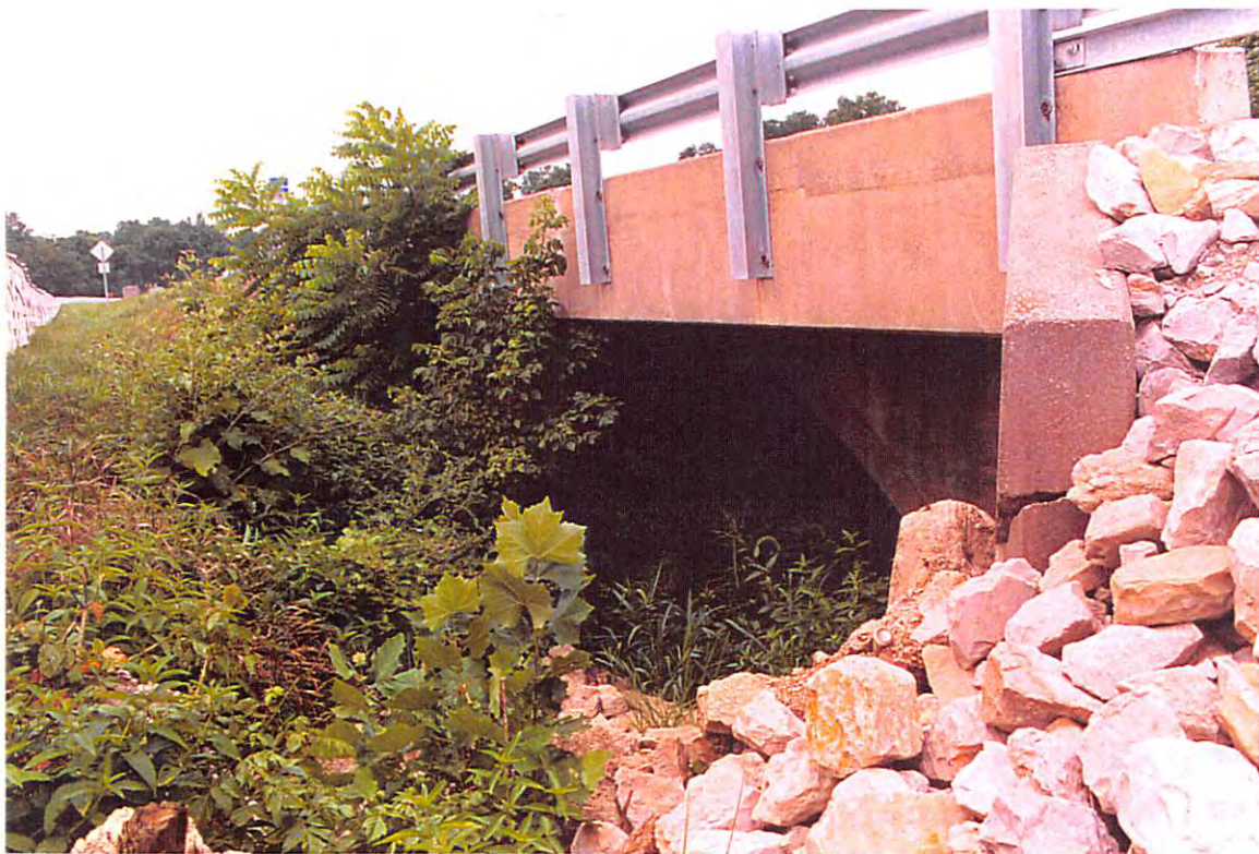
Looking northwest at Bridge Structure 150-59-0559 branch of Lick Creek
