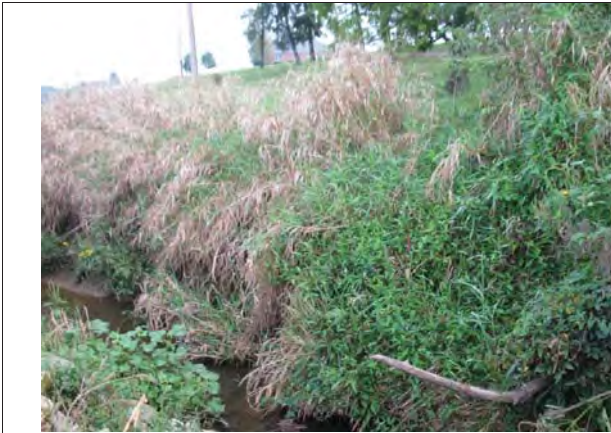
5. Looking at north bank on east side of the bridge.
