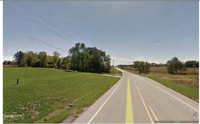
28. Looking southeast at drain inlet to underground culvert draining RSD 1 (Google Earth, Image Date: 09/2012).
