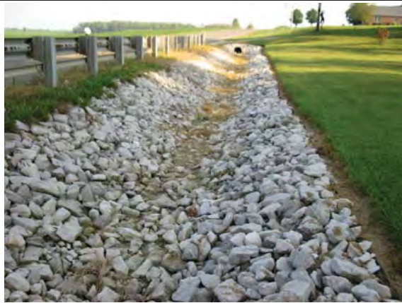
10. Looking north in roadside ditch (RSD) 1, riprap portion.
