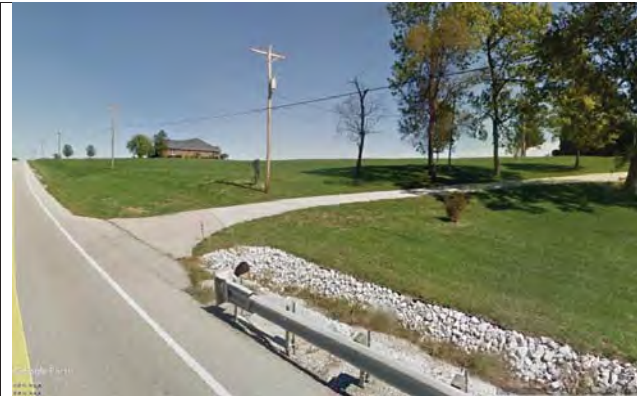
29. Looking northeast at outlet from underground culvert draining RSD 1 (Google Earth, Image Date: 09/2012).
