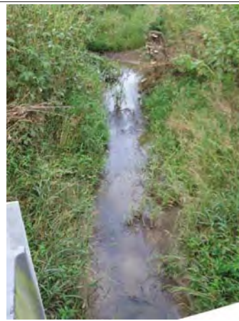
2. Looking northwest from bridge towards downstream of Wells Ditch.
