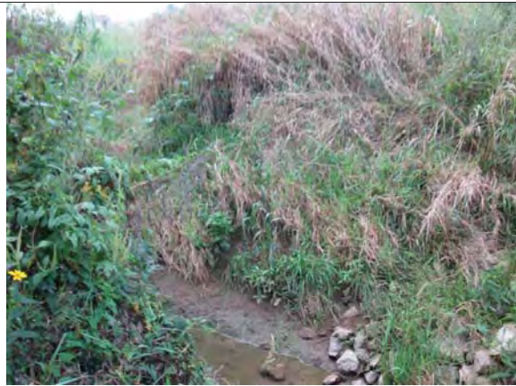
6. Looking at south bank on east side of the bridge.
