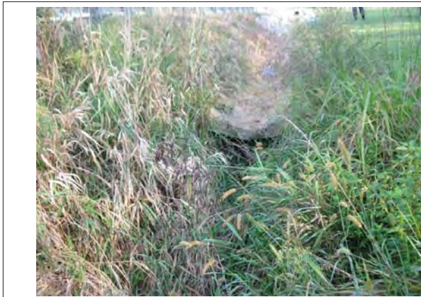
13. Looking north at concrete lined ditch in RSD 1.
