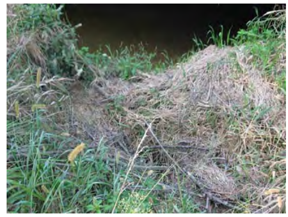
12. Looking at outfall point of RSD 1 into Wells Ditch.
