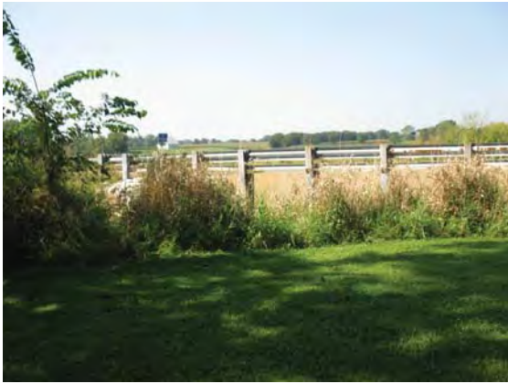
23. Looking southwest in the northeast quadrant of the investigated area.
