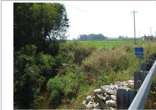
25. Looking southeast towards the southeast quadrant of the investigated area. RSD 3 in background.
