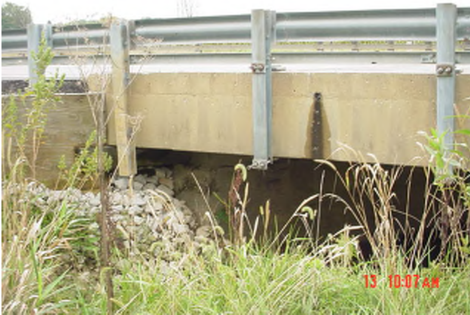
Looking at upstream side of bridge over Tilley Ditch.
