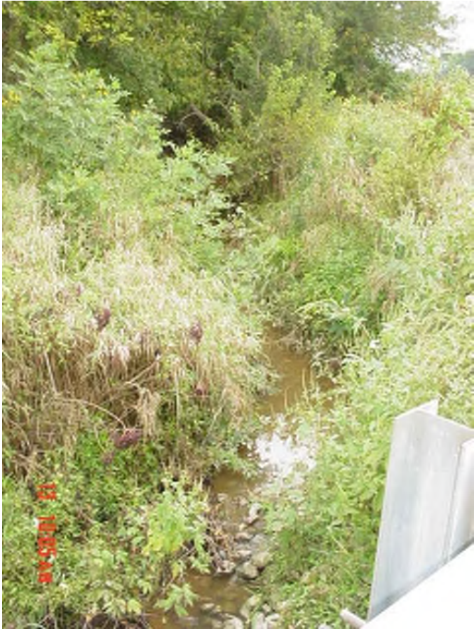
Looking upstream of bridge to be replaced.
