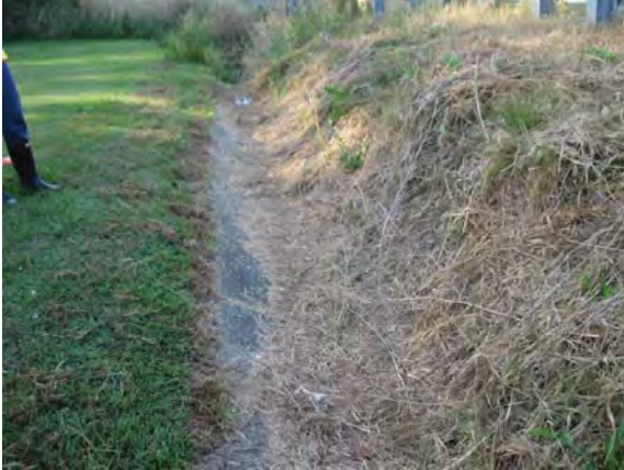
11. Looking south in RSD 1, concrete lined portion.
