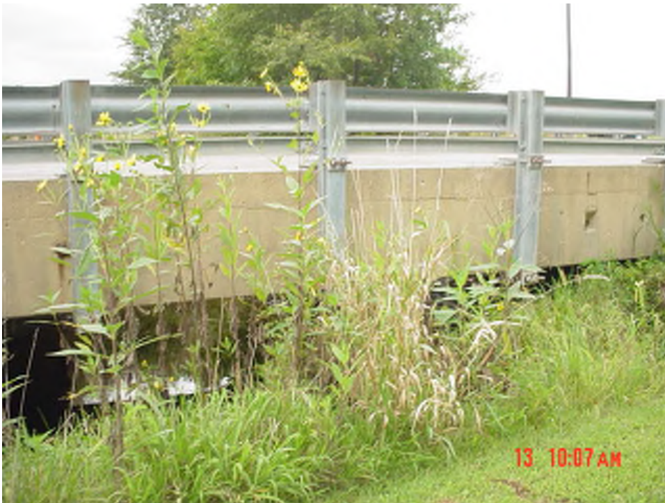
Looking at upstream side of bridge over Tilley Ditch.
