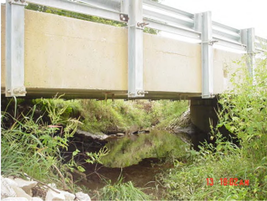
Looking at downstream section of bridge over Tilley Ditch.
