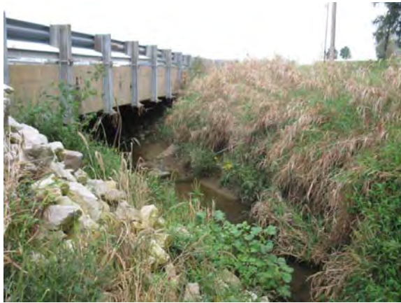
3. Wells Ditch on east side of bridge.
