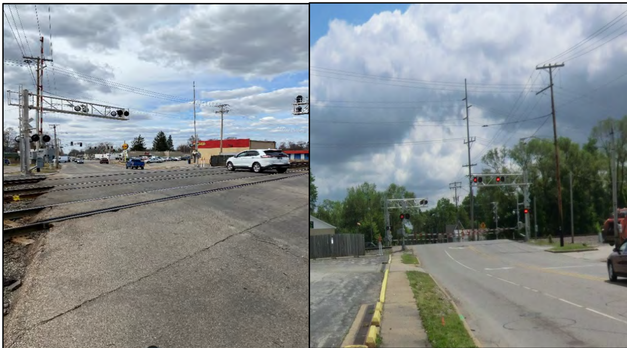
Figure 16. Hively Avenue and Norfolk Southern Railroad At-grade Crossing (Baker 2020)
