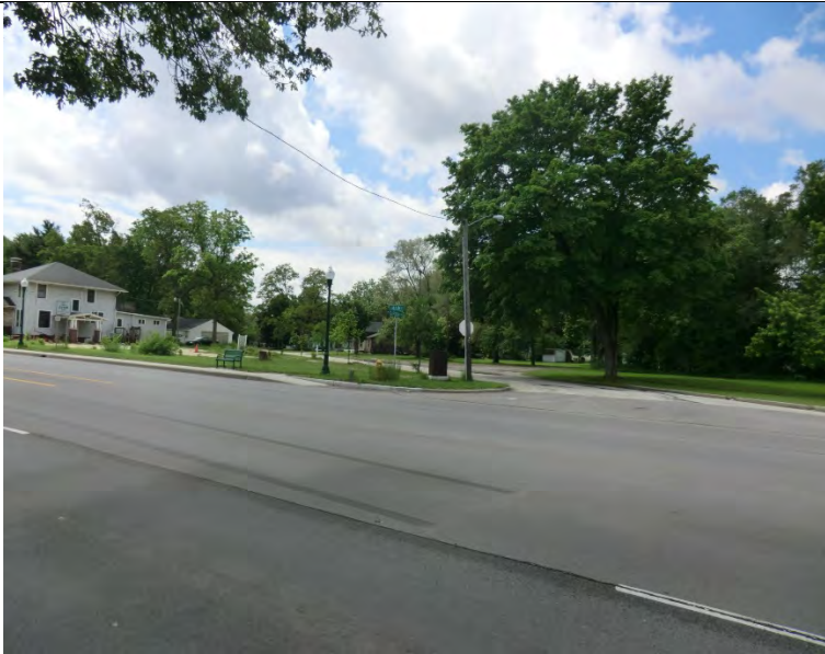
Photo 23: Facing south at South Main Street and Garden Boulevard
