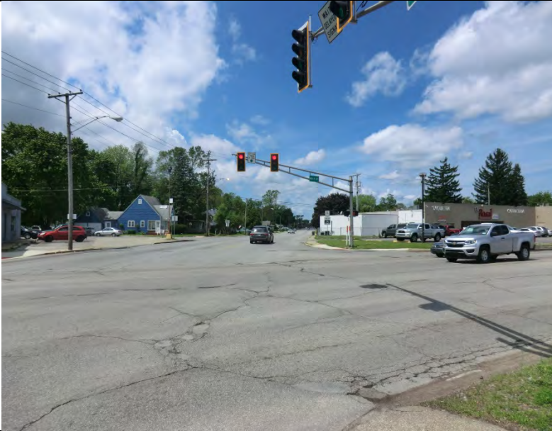
Photo 17: Facing west at Hively Avenue and South Main Street
