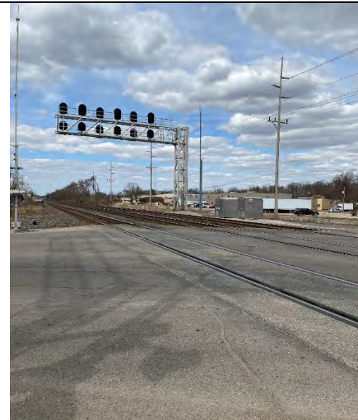
Photo 26: Facing northeast at Norfolk Southern RR Crossing
