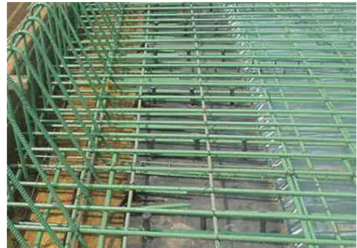
Figure 5-10 Shear Connectors
