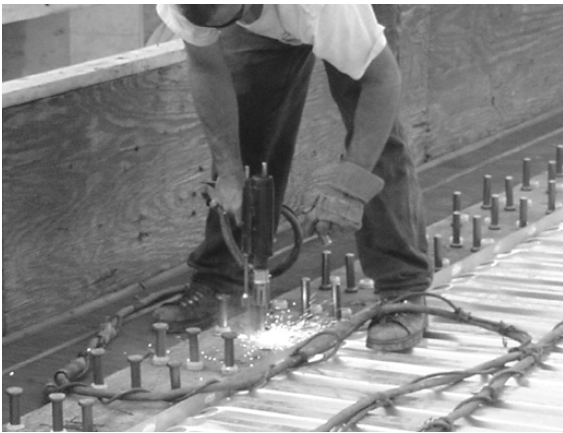
Figure 6-6 Shear Connector Studs
