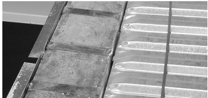
Figure 6-5 Deck Form Installation
