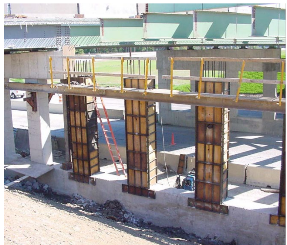
Figure 3-1 Bent Column Forms
