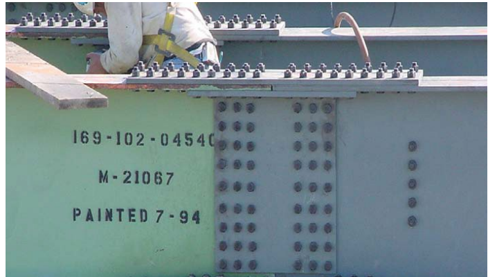
Figure 5-14 Splice Plate Bolts
