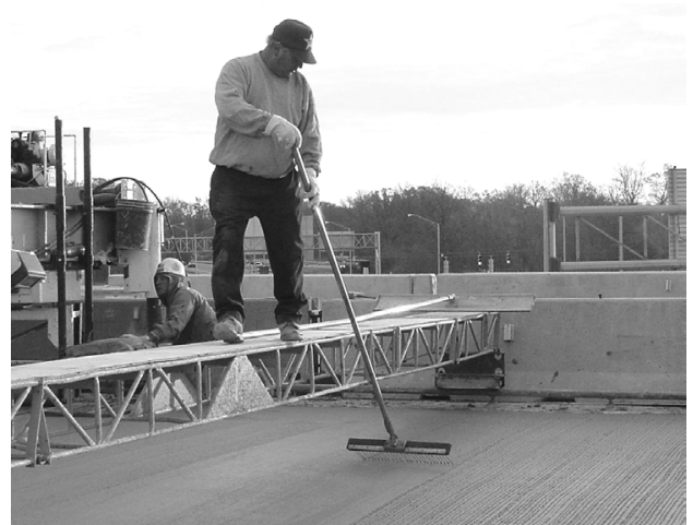
Figure 6-11 Concrete Finishing
