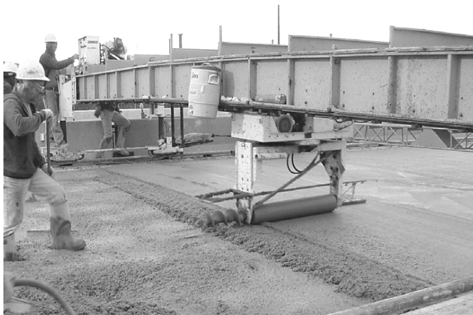
Figure 6-10 Concrete Vibrating and Striking Off
