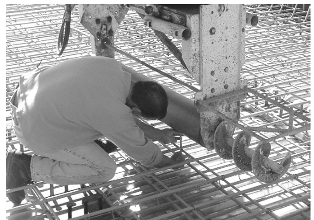
Figure 6-7 Checking Reinforcing Bar Clearance
