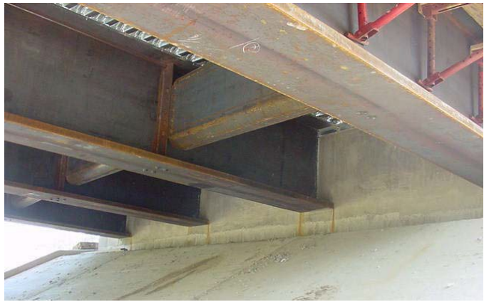
Figure 5-2 Integral End Bents
