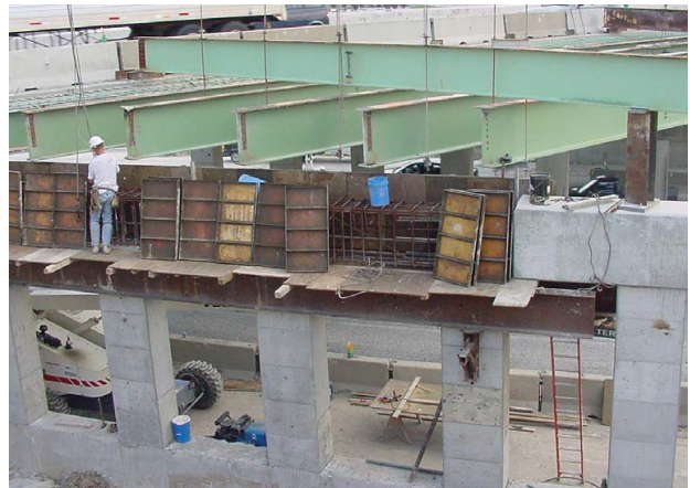
Figure 3-7 Formwork
