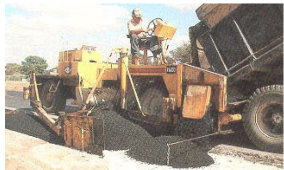
Figure 7-1 HMA Widening
