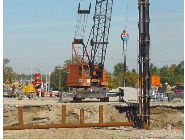
Figure 2-3 Foundation Piles
