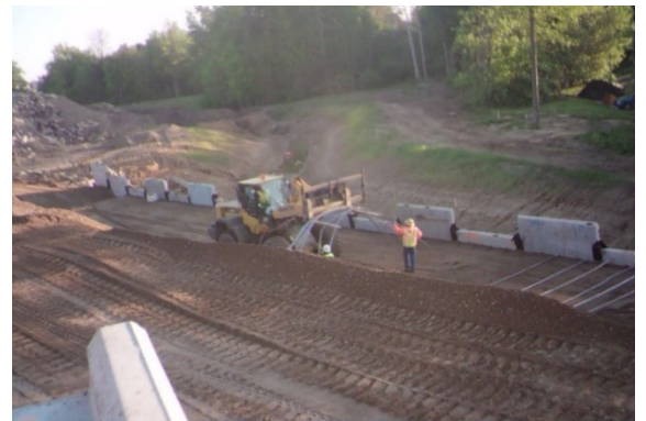
Figure 10-8 Reinforcement Strap Installation
