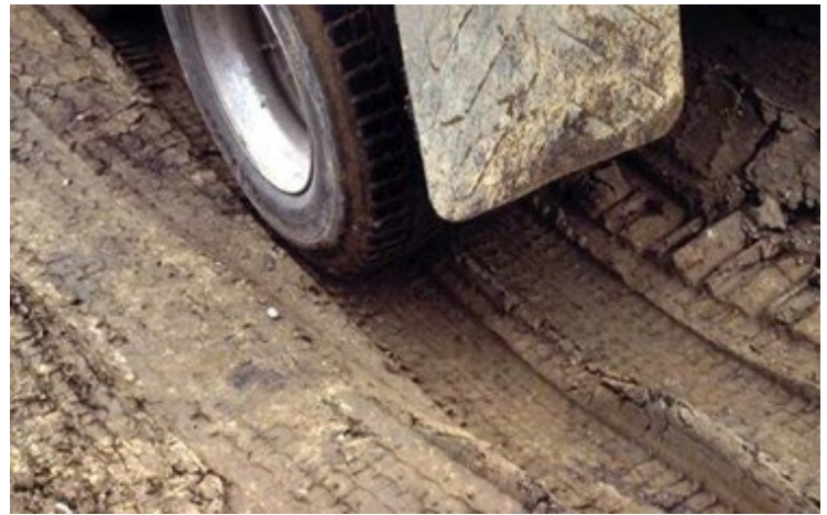
Figure 10-2 Unacceptable Compaction
