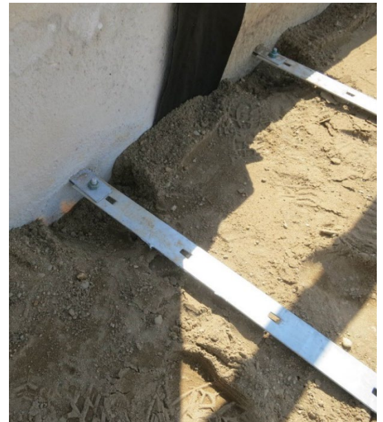
Figure 10-7 Proper Strap Attachment
