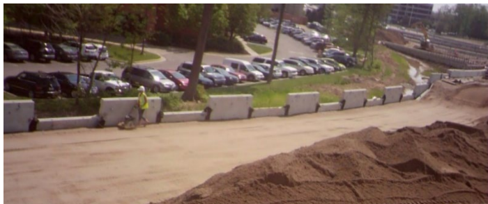
Figure 10-4 Five Passes of Plate Compactor within 3' of Wall
