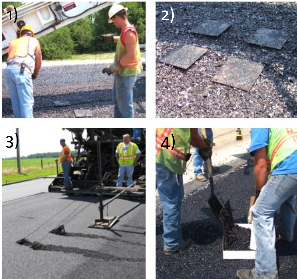
Figure 7-6 Plate Sampling: 1) Setting plates; 2) Final plate arrangement; 3) Locating plates after paving; 4) Collecting loose HMA material for testing
