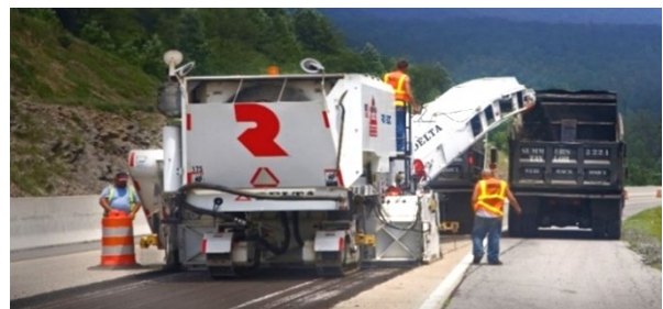
Figure 4-2 Milling Machine
