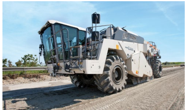
Figure 4-1 Chemically Modifying Soil
