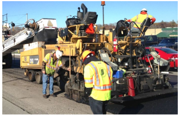
Figure 3-2 HMA Paver
