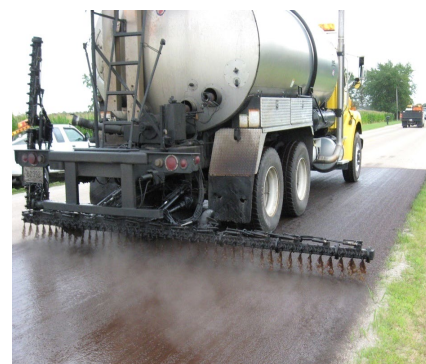
Figure 4-7 Tack Coat Application
