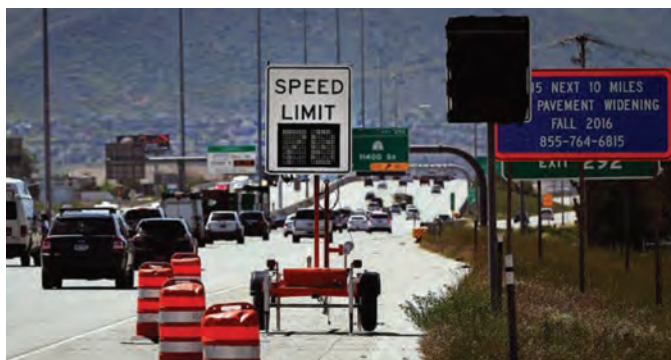
Figure 2.5. Regulatory PVSLS trailer at a Utah work zone (Credit: Street Smart Rental).
