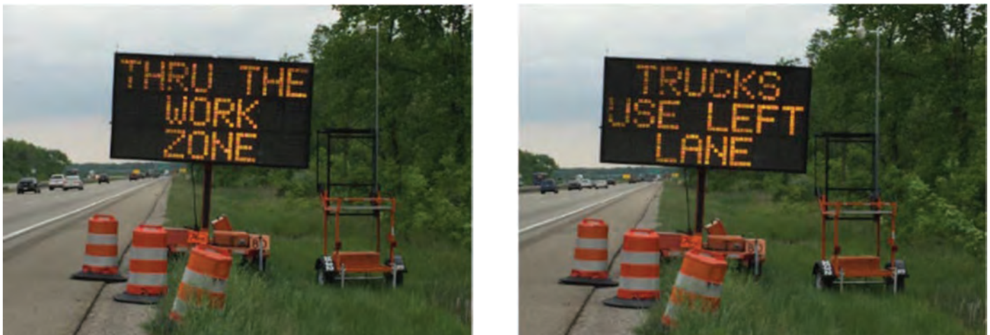
Figure 3.12. Work zone truck-lane restriction (Credit: KLS Engineering).
