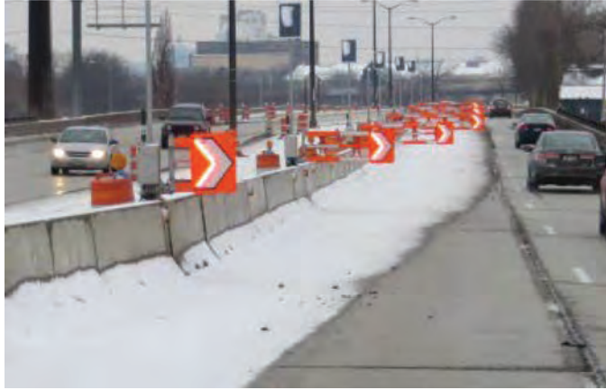
Figure 3.10. Reversible lane operations using moveable barrier and swift gate (Credit: WisDOT).
