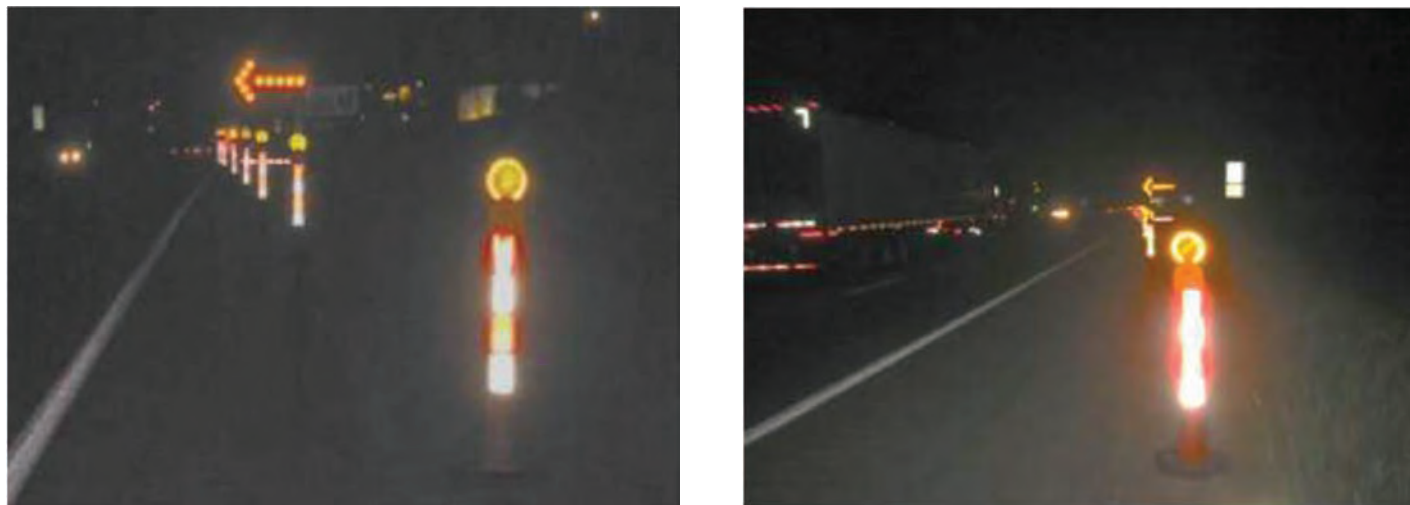
Figure 2.11. Sequential warning lights (Credit: University of Missouri).
