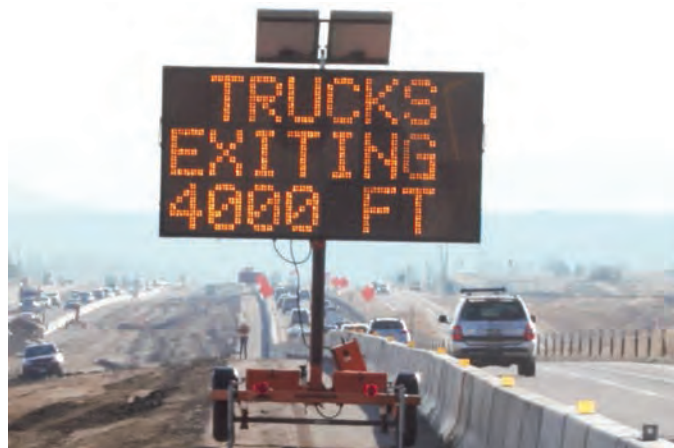
Figure 10.3. I-25 Construction truck warning system (Credit: CDOT).
