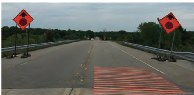
Figure 2.10. Orange polymer rumble strips with adhesive (Credit: MDOT).
