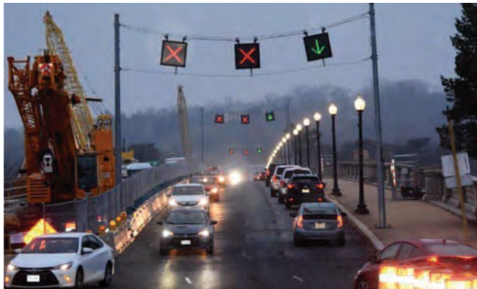
Figure 3.7. Reversible lane operations on Arlington Memorial Bridge using lane-use control signals (Credit: Dave Dildine/WTOP).
