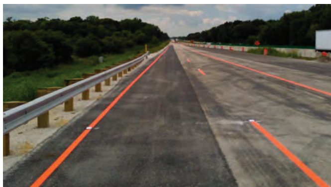
Figure 12.13. WisDOT use of orange pavement markings (Credit: John Shaw/University of Wisconsin–Madison).
