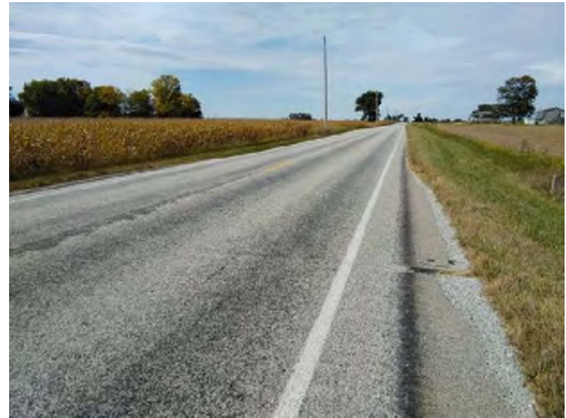
PP-48; Looking west at the east end of the project area (9-30-2020).
