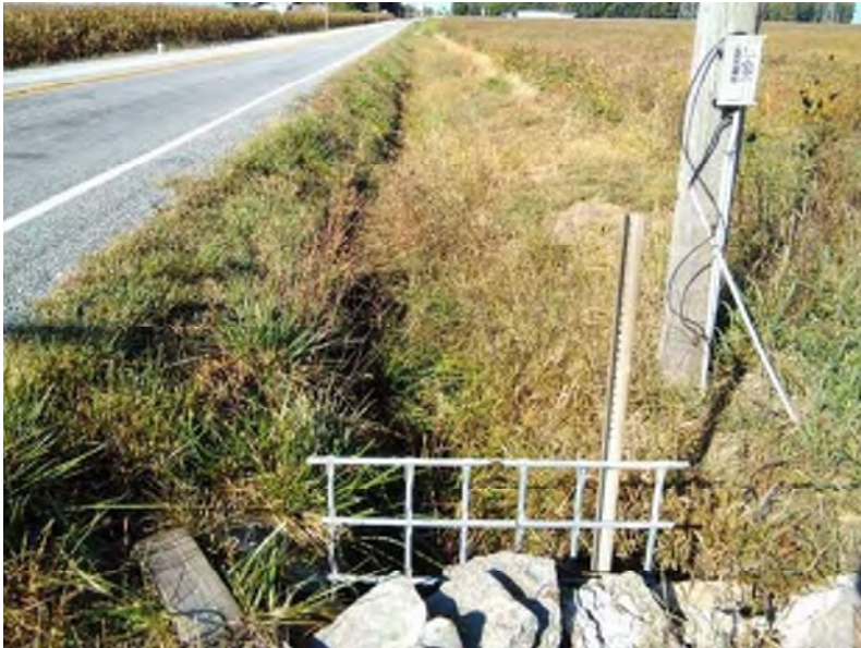
PP-7; Looking west at non-jurisdictional RSD 1 (9-29-2020).
