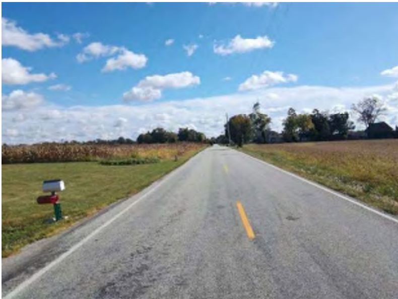
PP-23 Looking east along SR 244 showing typical mowed ROW and farm fields along the project area (9-29-2020).
