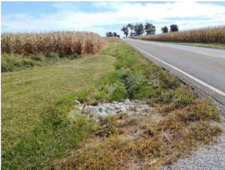
PP-47; Looking east at non-jurisdictional RSD 3 (9-30-2020).
