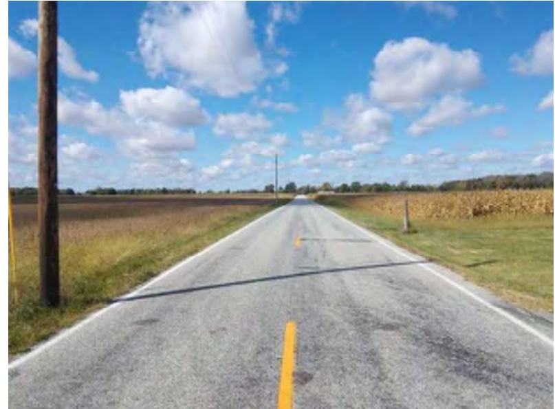
PP-22; Looking west along SR 244 showing typical mowed ROW and farm fields along the project area (9-29-2020).
