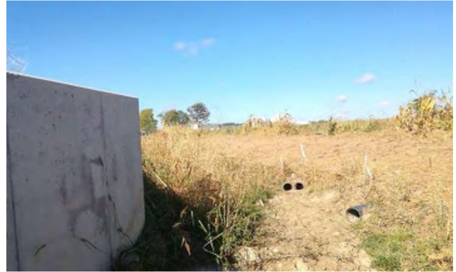
PP-10; Looking west at tile outlets that feed UNT 2 (9-29-2020).
