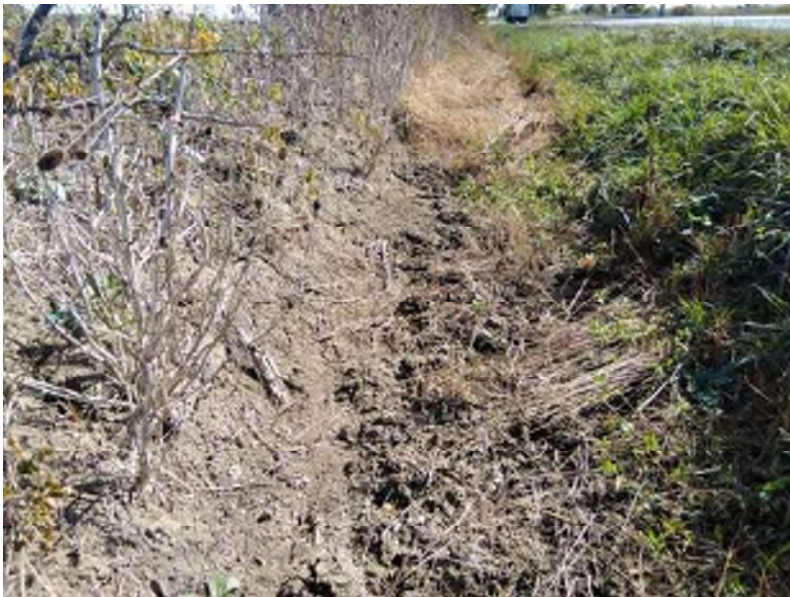
PP-19; Looking east at RSD 2 (9-29-2020).
