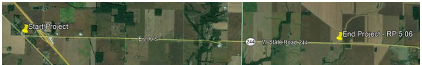
Figure 1: SR 244 Existing Aerial
