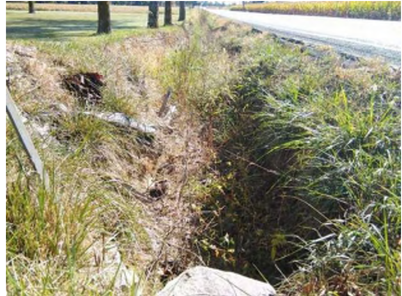
PP-8; Looking east non-jurisdictional RSD 1 (9-29-2020).
