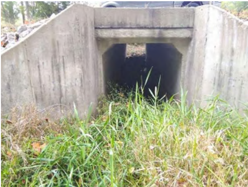
PP-36; Looking north at the culvert that conveys UNT 4 under SR 244 (9-29-2020).
