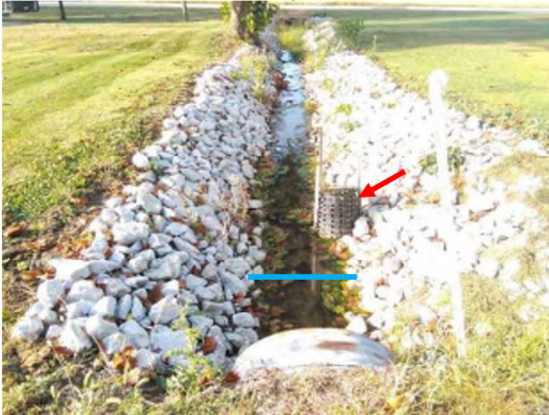
PP-1; Looking southwest, downstream at UNT 1 (9-29-2020). OHWM 39.497141, -85.699807 and overflow drain
