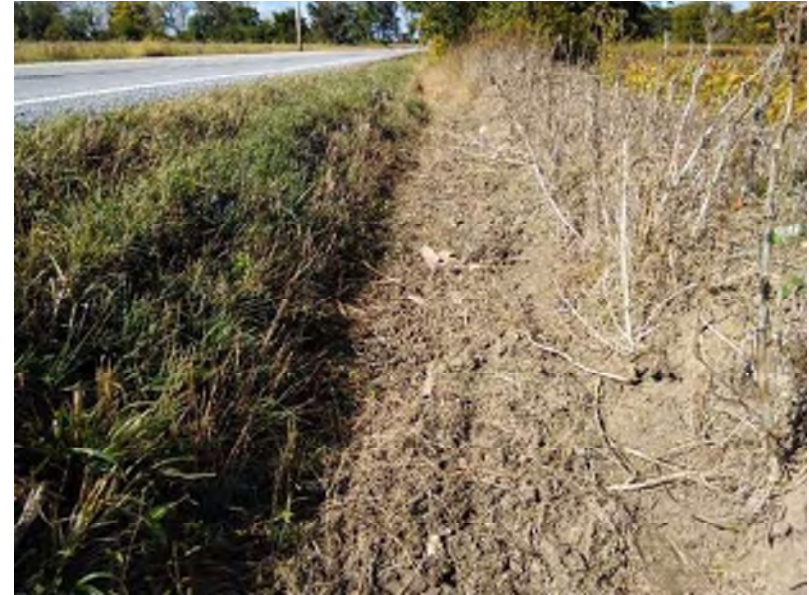
PP-18; Looking west at RSD 2 along the north side of SR 244 (9-29-2020).
