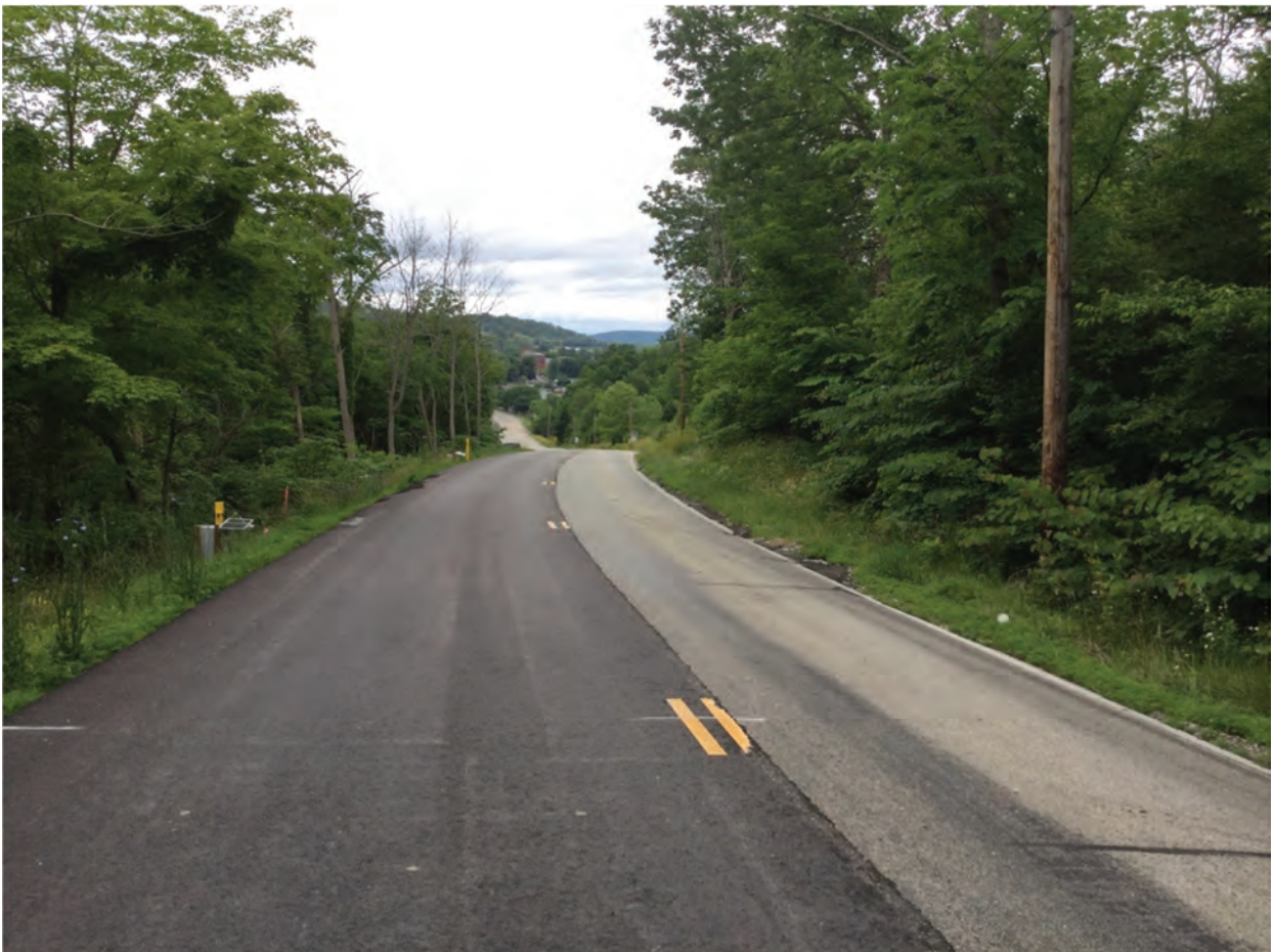
8. Looking west along SR 252
