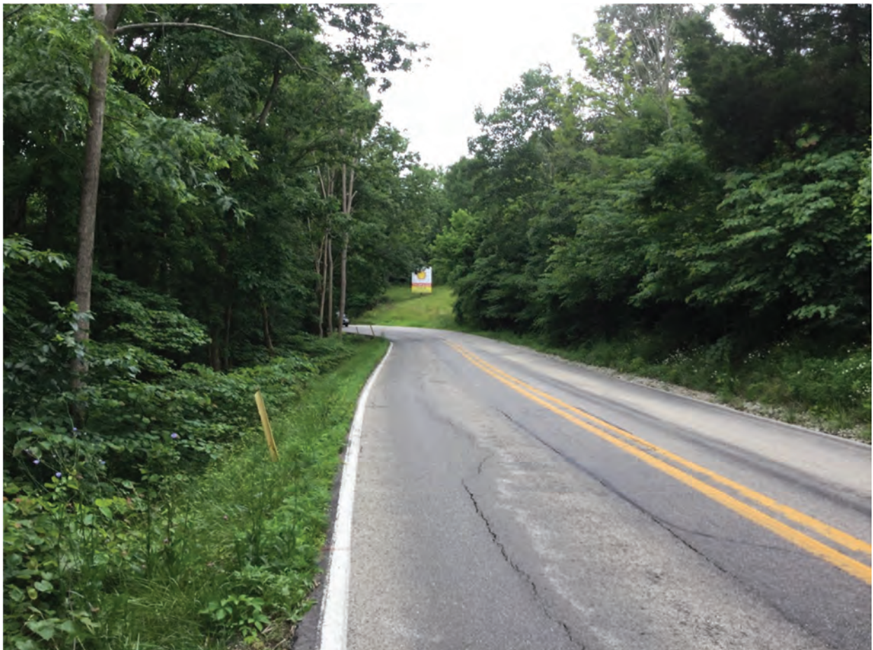
18. Looking west along SR 252
