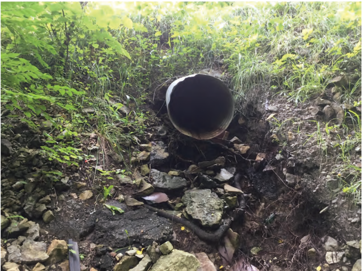
14. Looking north at culvert conveying UNT 2 to East Fork Whitewater River
