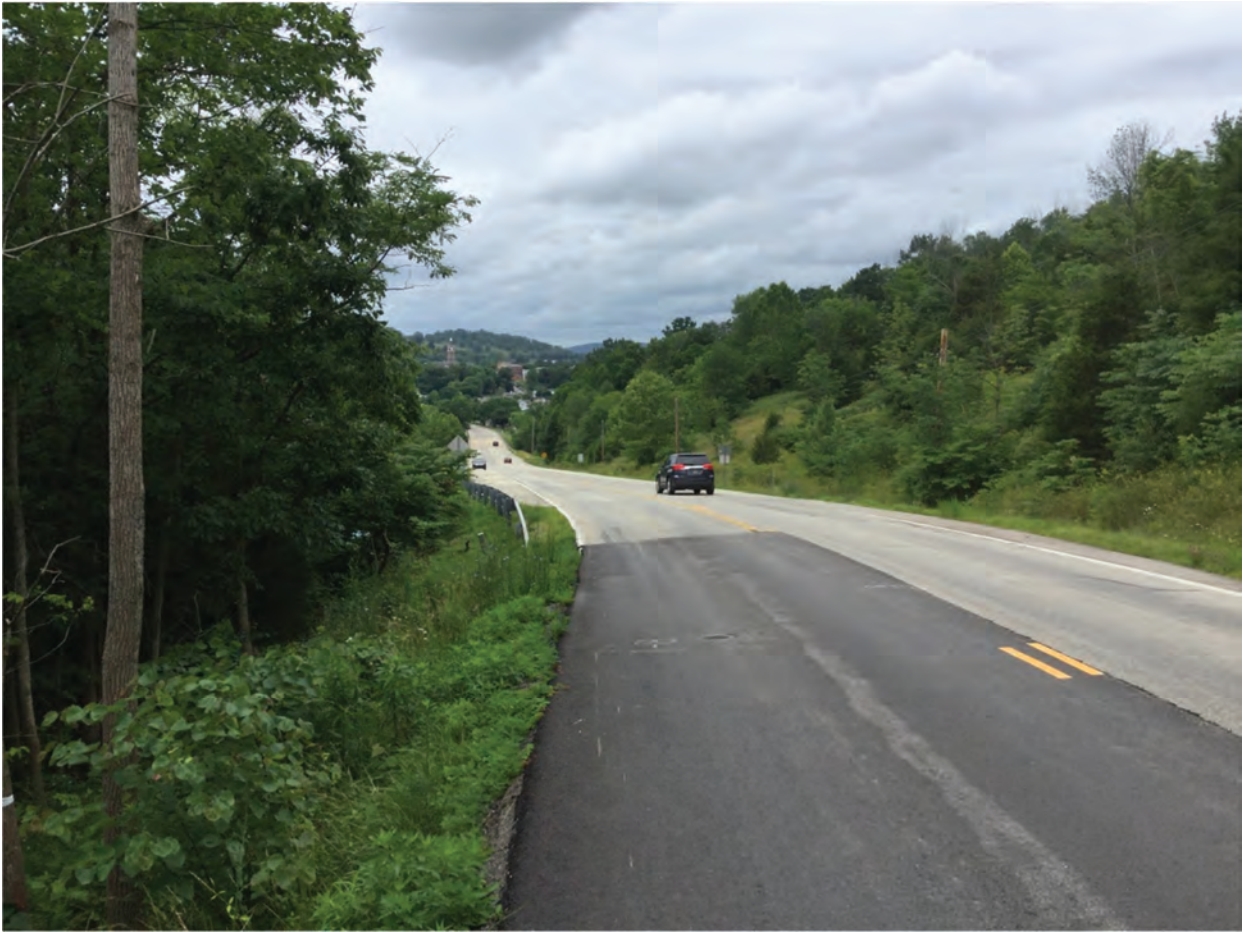
5. Looking west along SR 252
