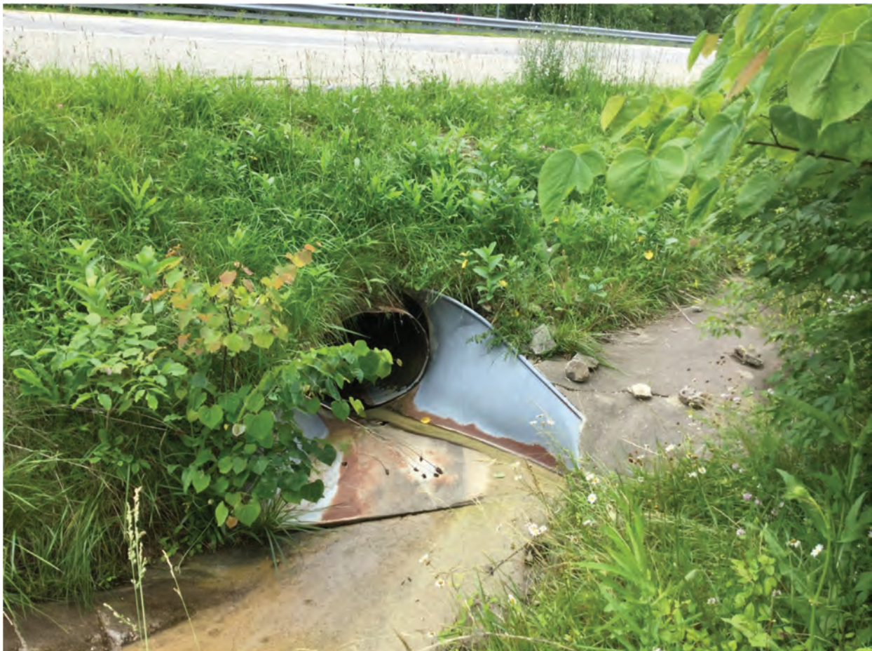
4. Looking south at culvert under SR 252
