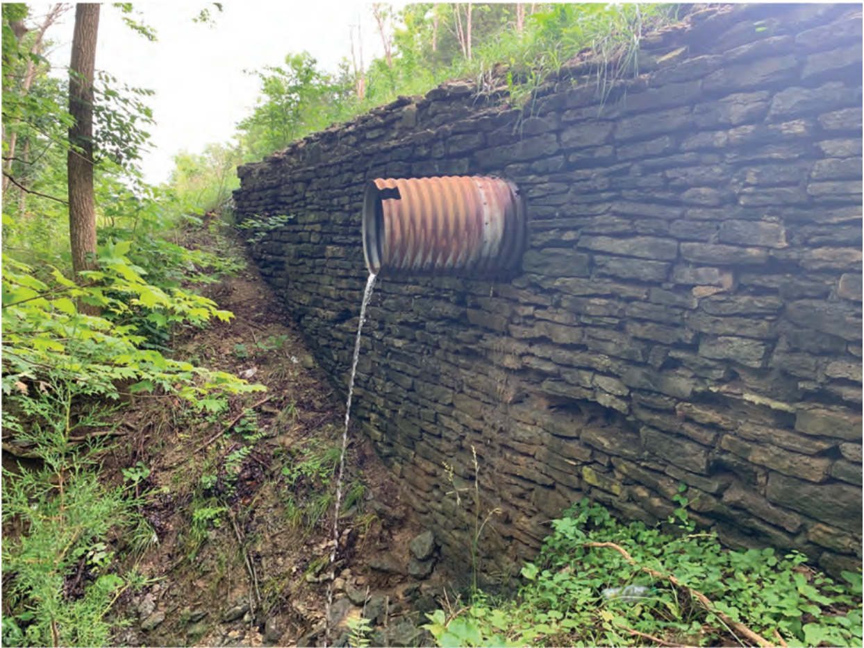
11. Looking northwest at culvert conveying UNT 3 to East Fork Whitewater River
