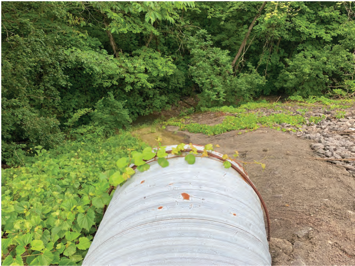
3. Looking southwest at culvert from SR 252
