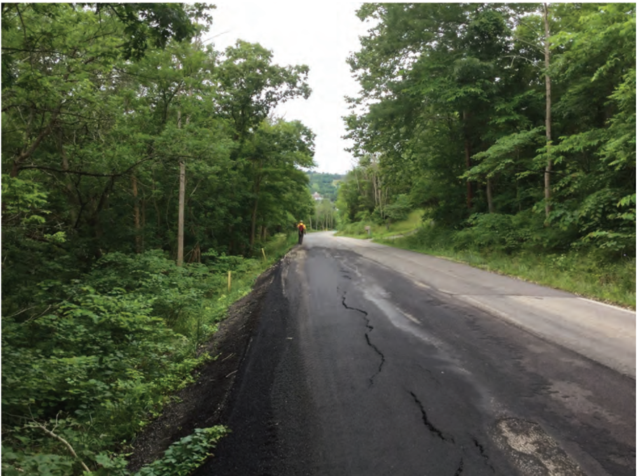
12. Looking west along SR 252
