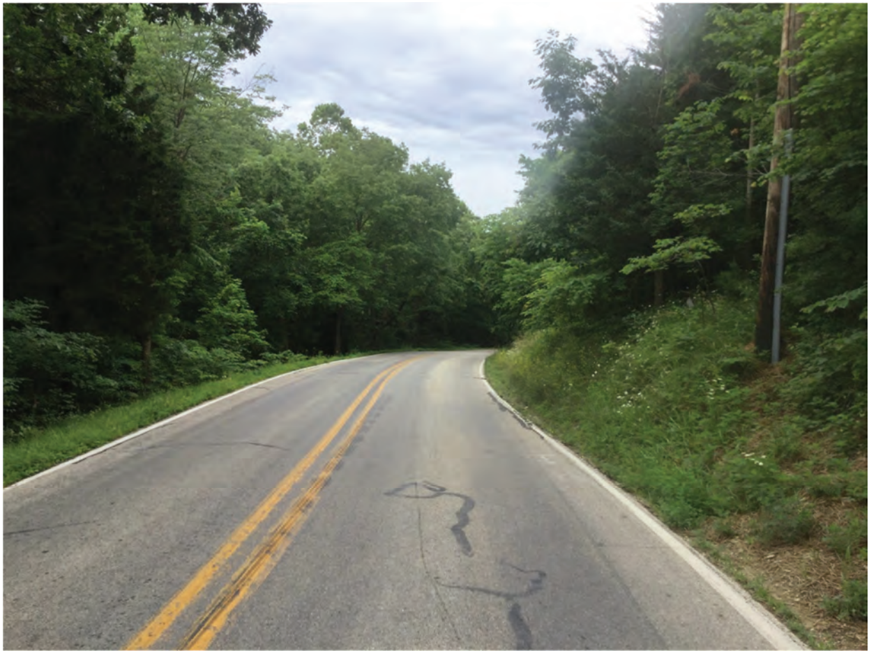
19. Looking west along SR 252
