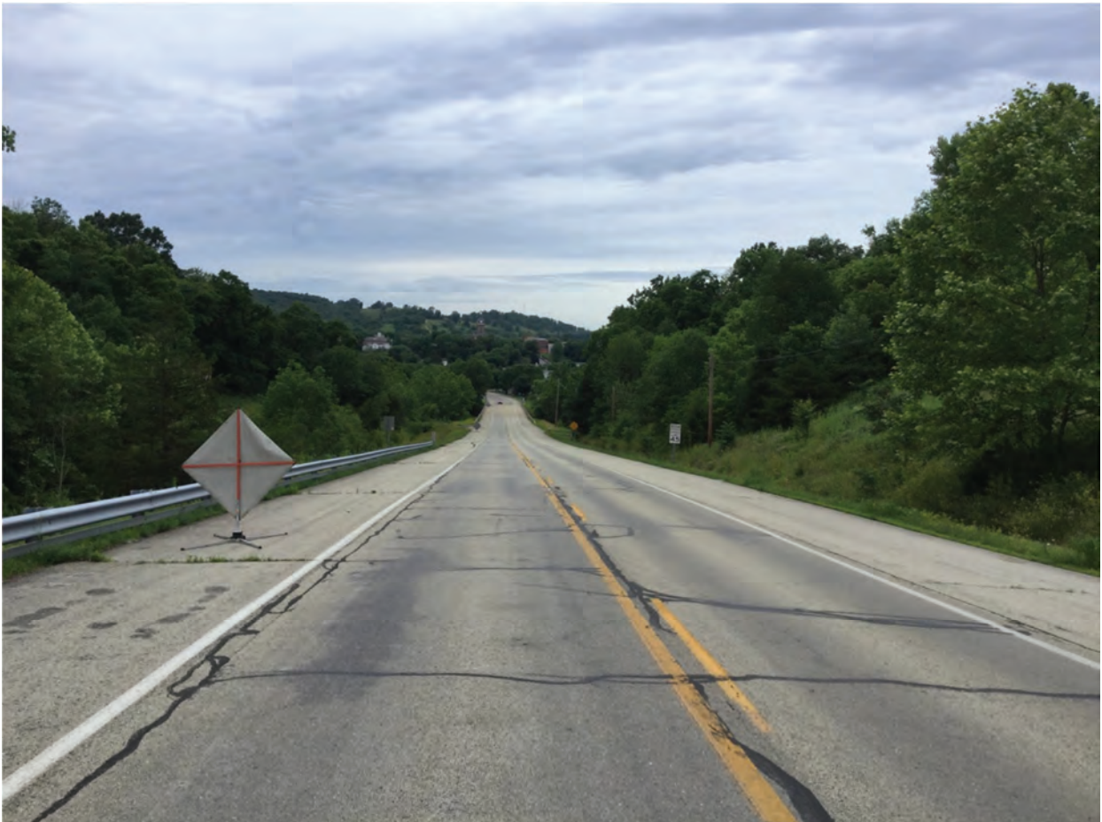
2. Looking west along SR 252
