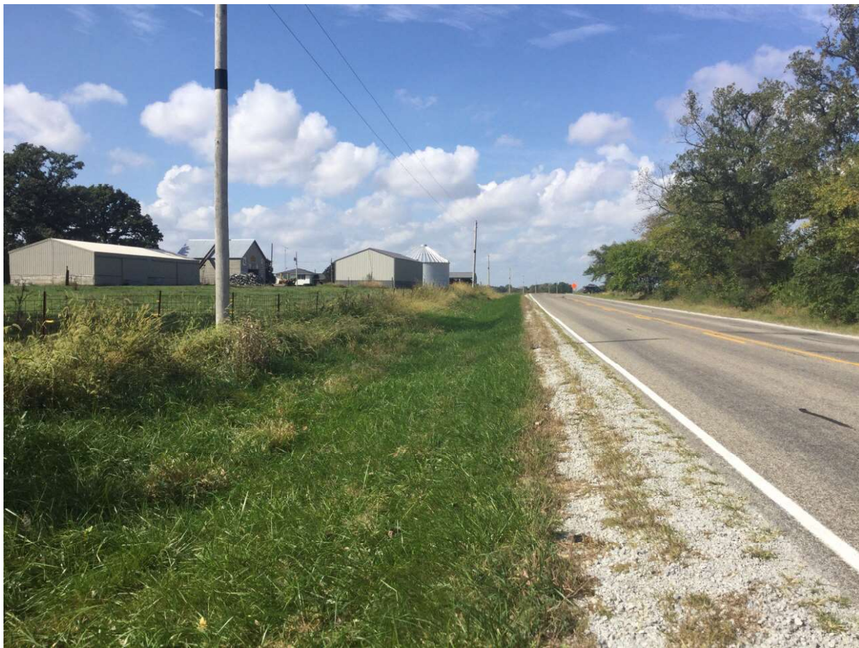
1. Looking west along SR 14.
