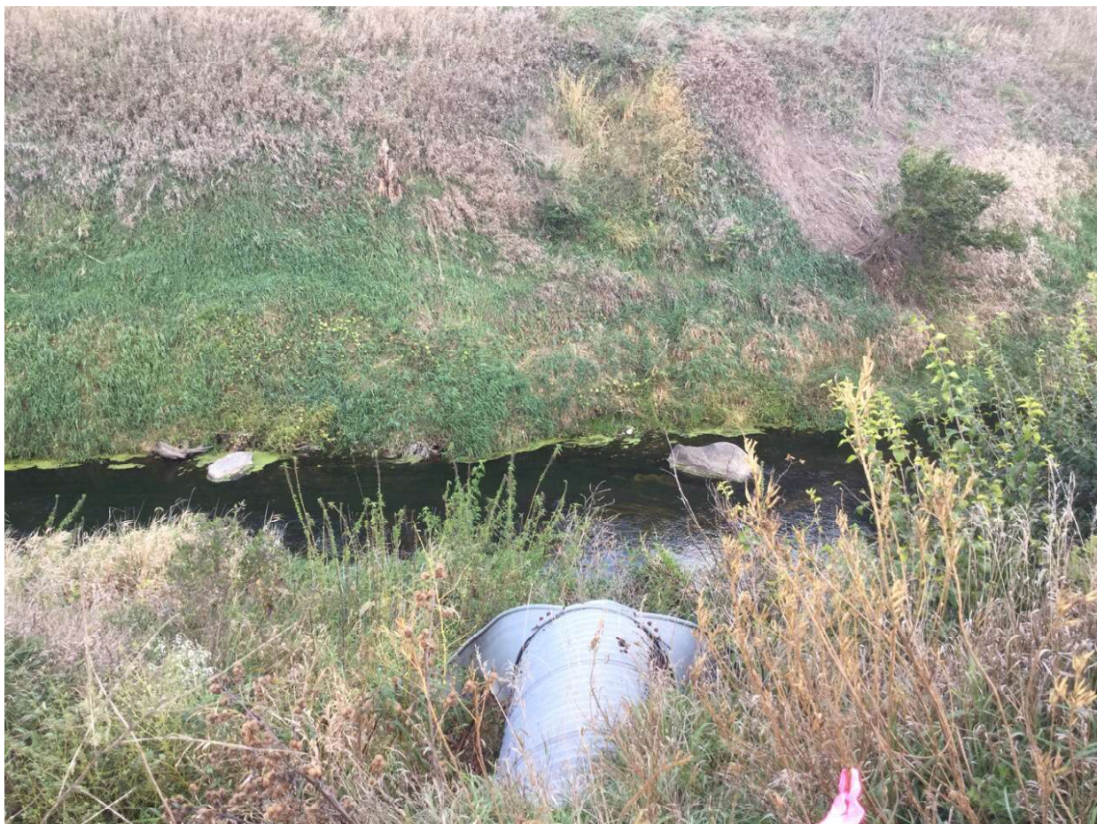
10. Looking north from culvert outlet towards Oliver Ditch.
