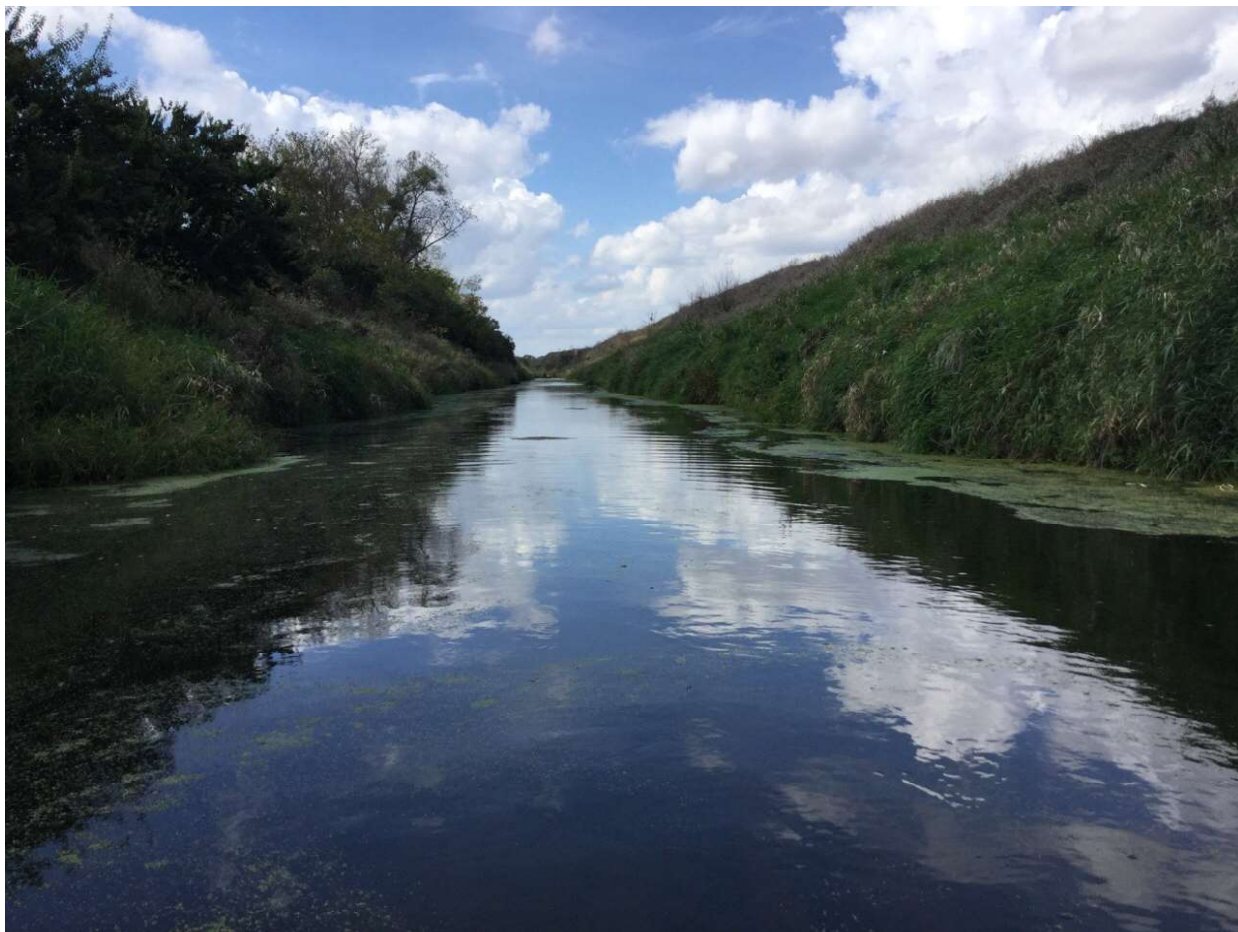
7. Looking west downstream Oliver Ditch.
