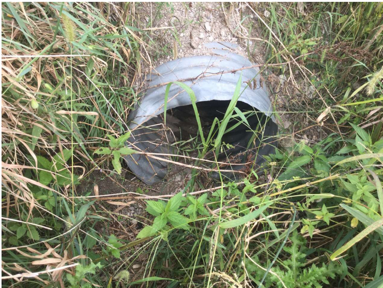
9. Looking north toward structure on south side of SR 14.
