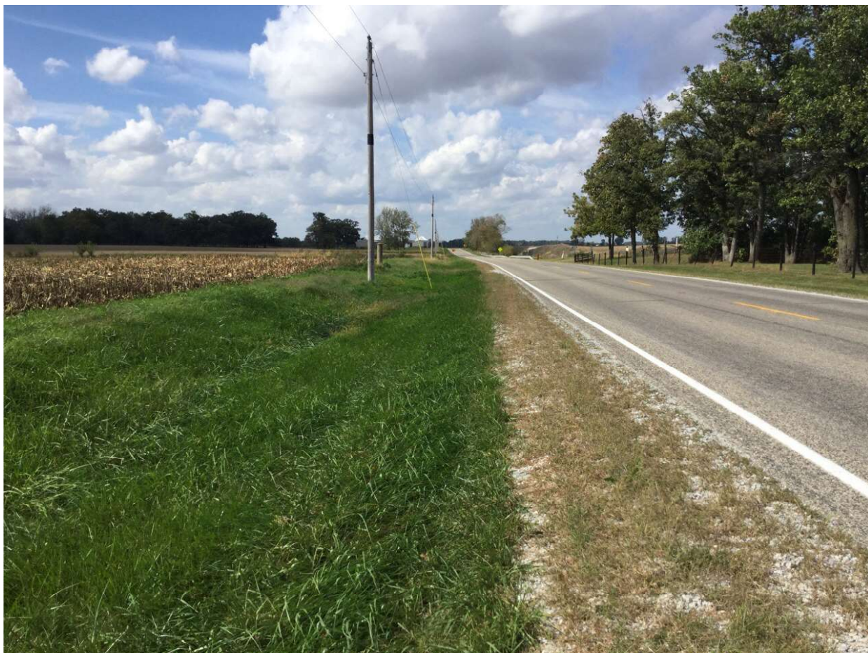
12. Looking west along SR 14.
