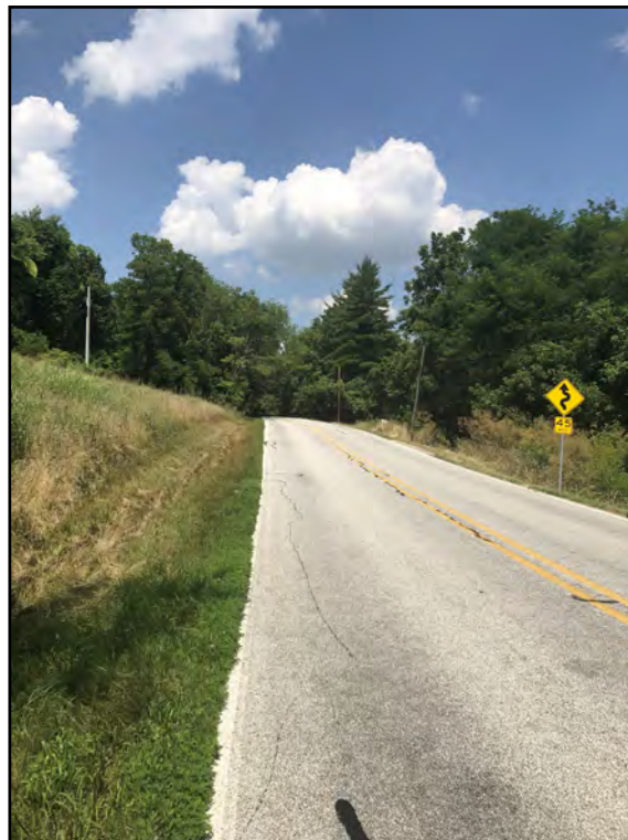
Photo 2: Looking northeast at SR 56 from the culvert.
