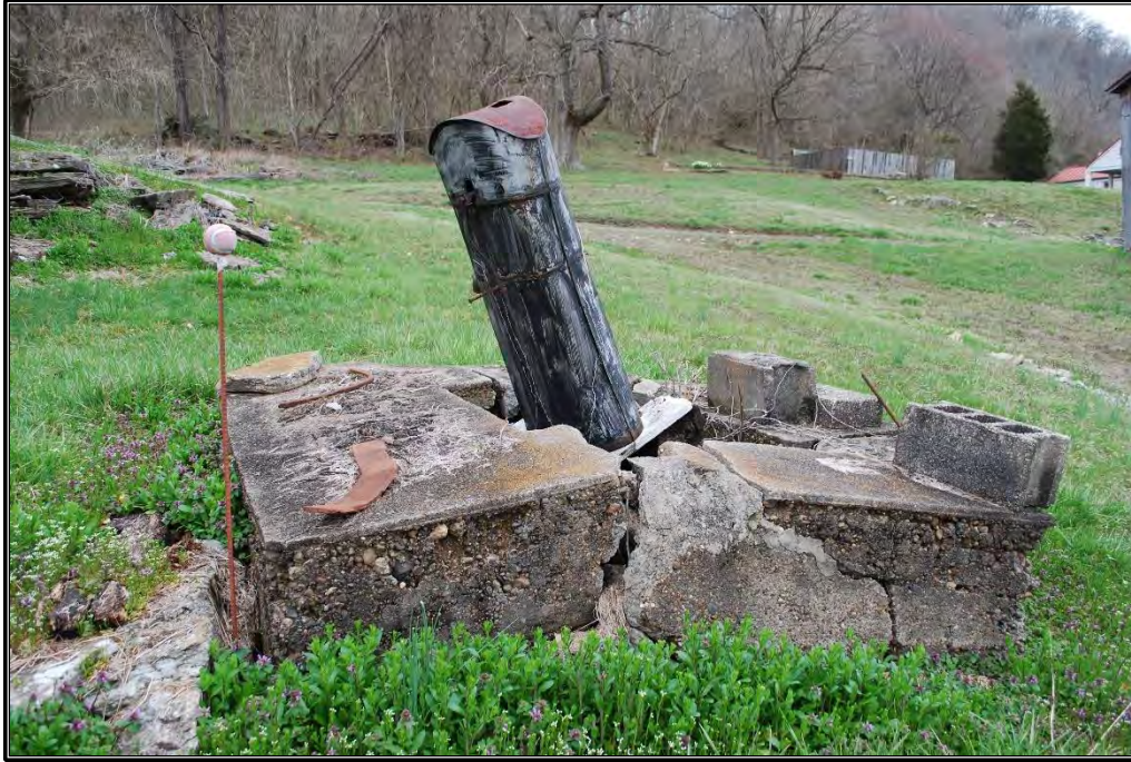
Figure B-24. Well (Resource L), facing north.
