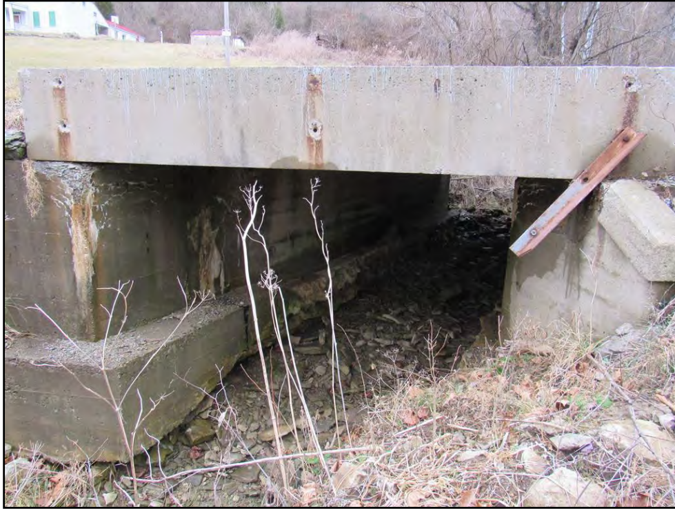
Photo 11: South side of culvert. Taken from engineering report photos.
