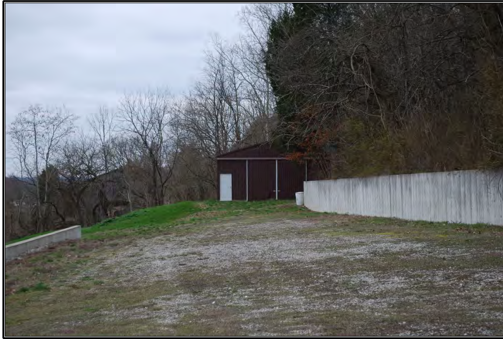
Figure B-26. East elevation of pole barn (Resource N), facing southwest.
