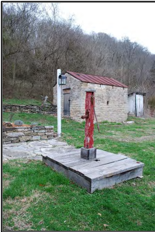
Figure B-23. Well with pump (Resource K), facing north.
