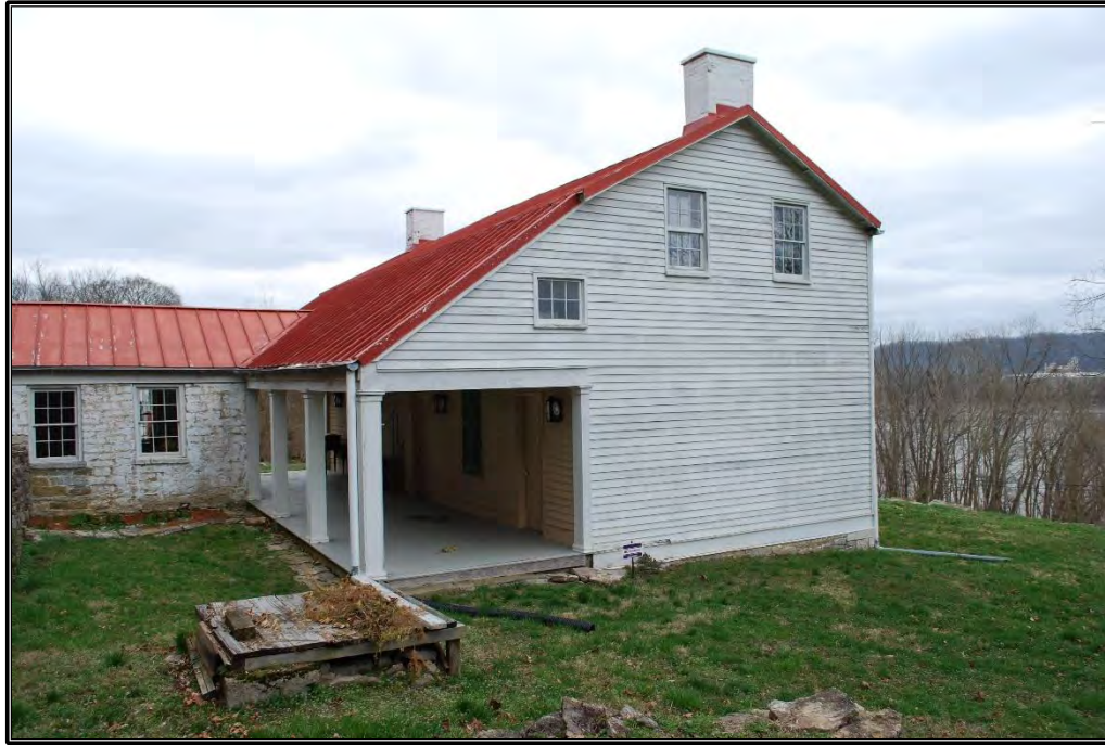
Figure B-4. Rear (north) and west elevations, facing east.
