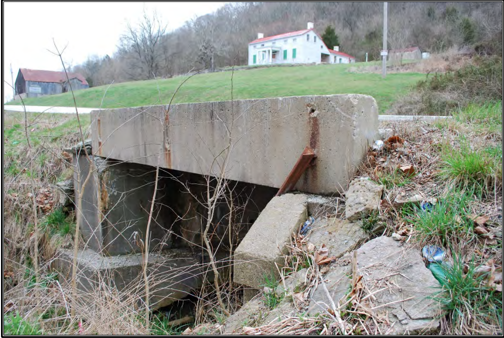
Figure 3. View of culvert (CV 056-078-158.30), south elevation and APE, facing northwest
