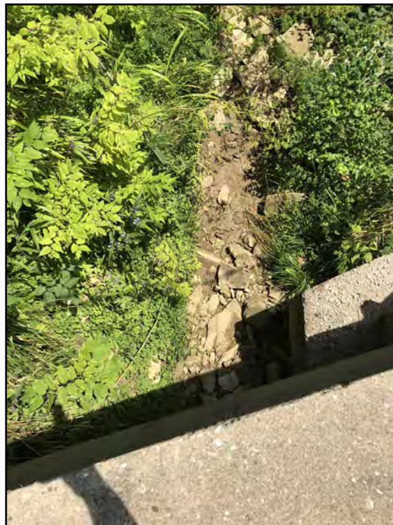
Photo 10: View of the bank of the southeast side of the culvert. Channel is saturated but no surface water is present.
