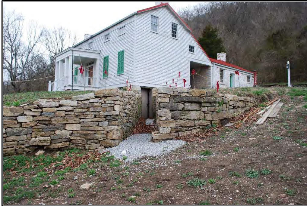
Figure B-6. New basement access, east elevation, facing west.
