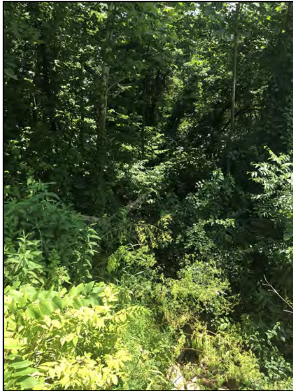
Photo 7: Looking over the southeast side of the culvert from road level.
