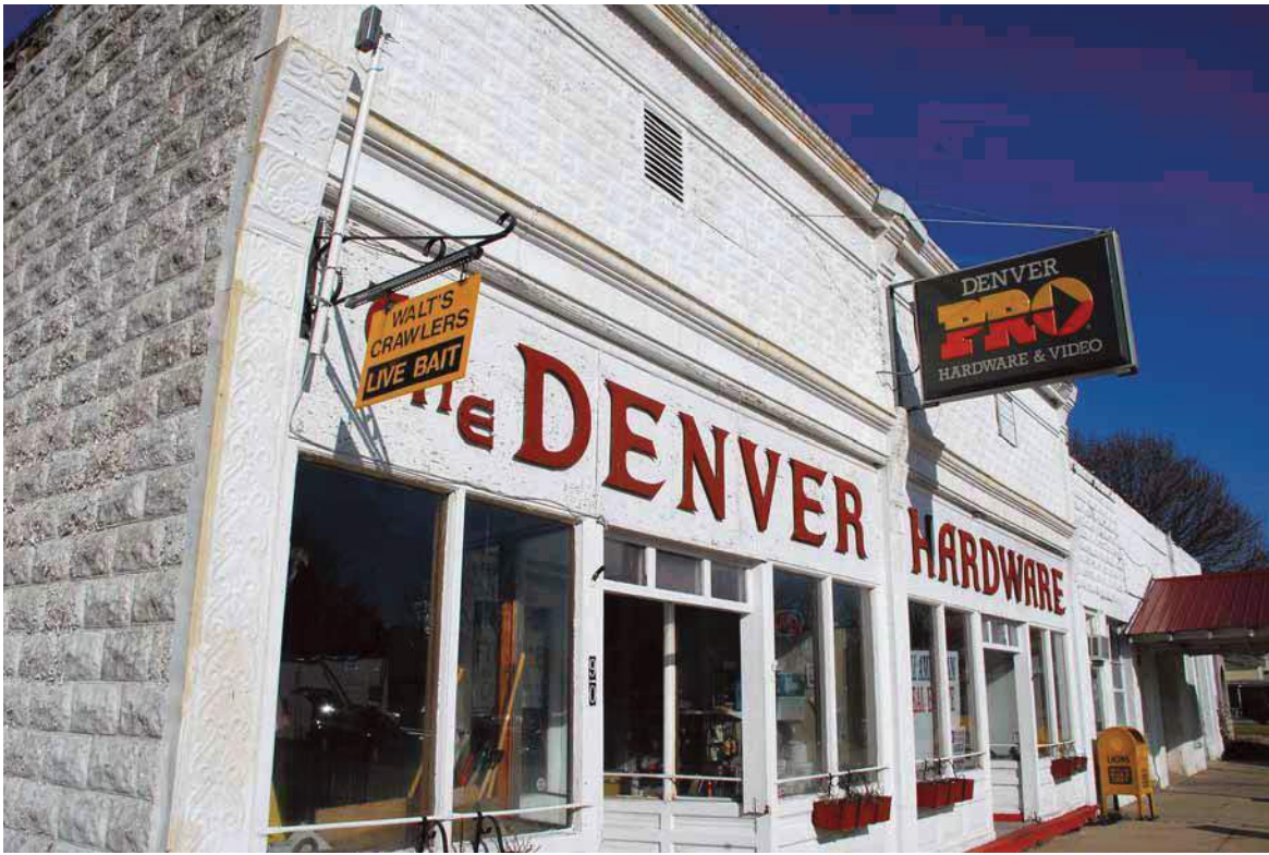
7. The facade of the Denver Hardware building (103-507-21019) at 90 W Harrison St
