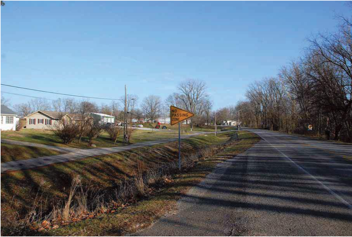
1. View looking east from west end of APE
