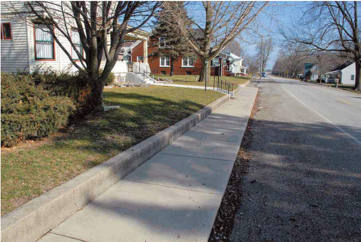
16. View of the wall in front of 224 E Harrison (103-507-21016)
