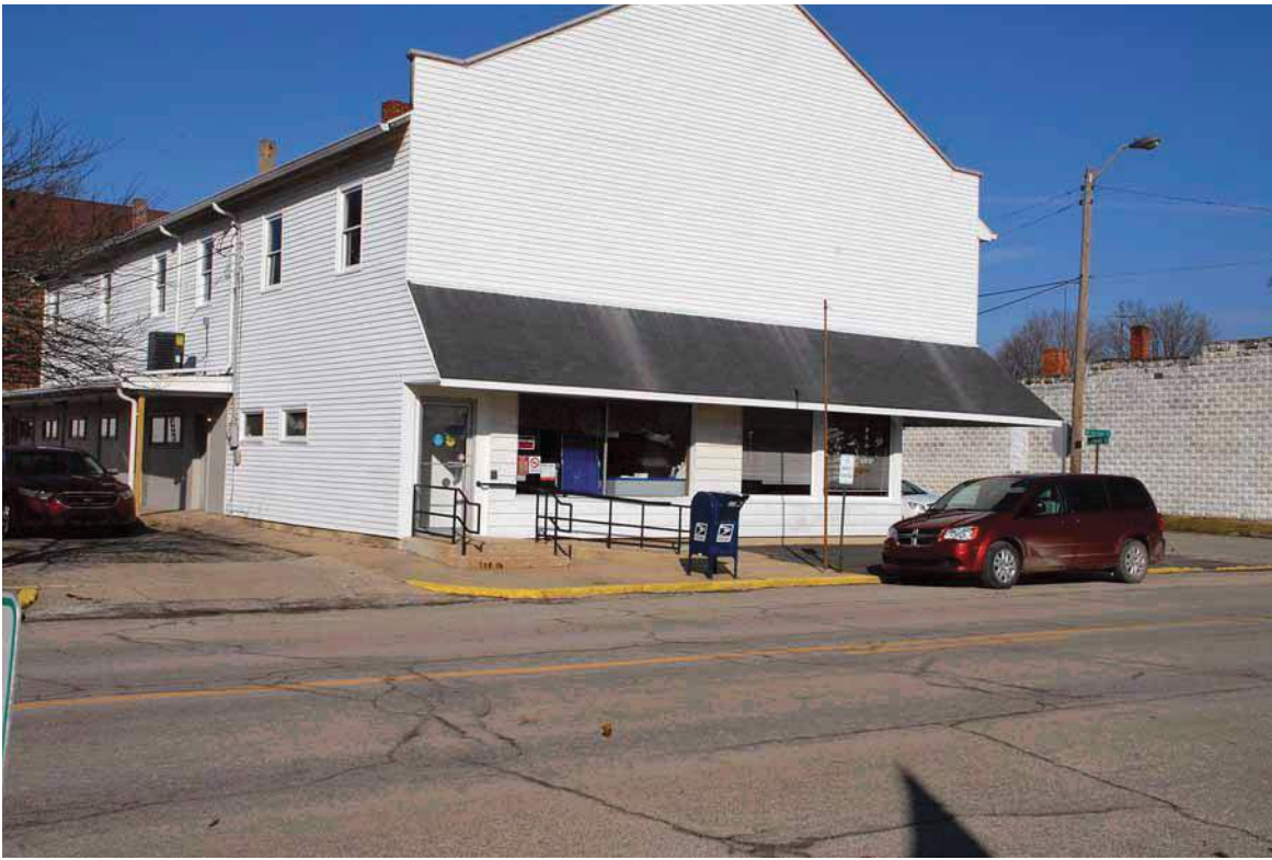
5. Commercial Building at 106 W Harrison (WA3)
