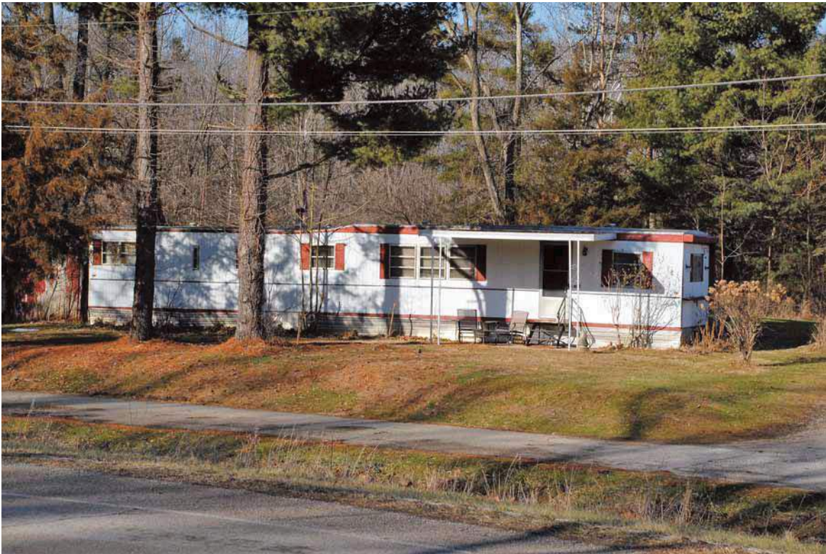
2. Non-contributing mobile home at 466 Harrison St
