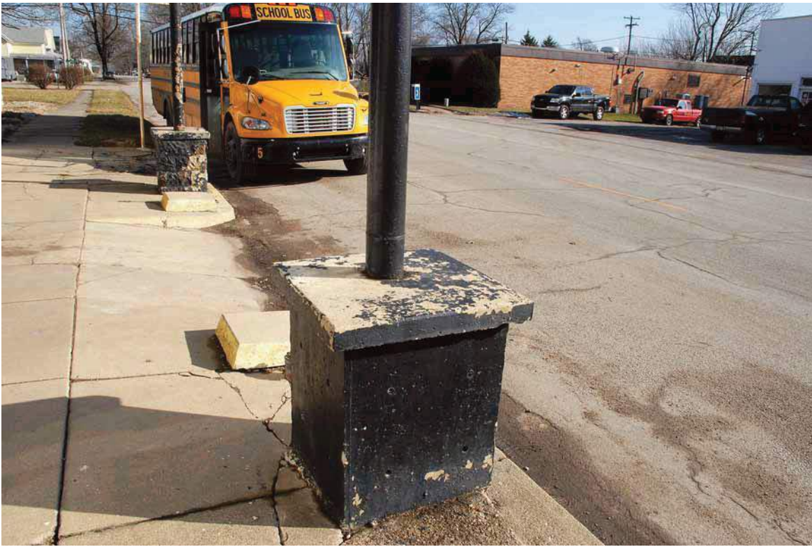
9. View of roof columns at 76 W Harrison St (WA4)
