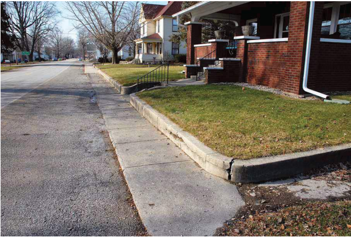
19. View of retaining wall in front of 246 E Harrison St (103-507-21015)
