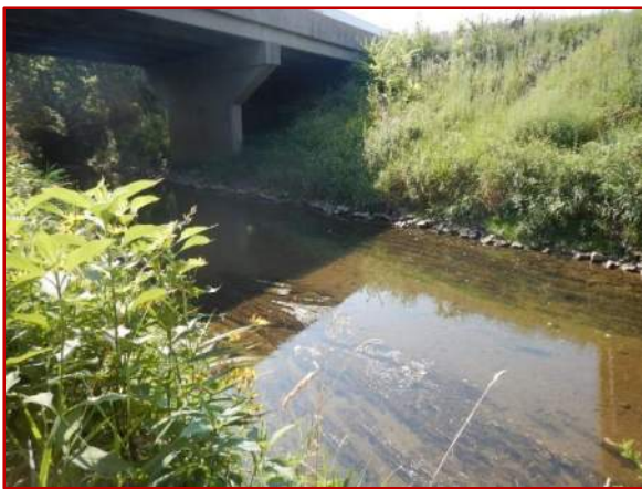
Photo 11: Looking northwest, within the I-65 median.
