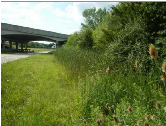
Photo 5: Looking northwest, east of I-65 northbound and north of the Lafayette Avenue exit ramp.
