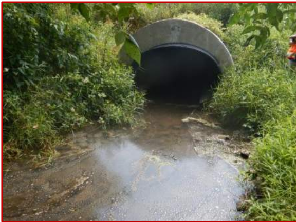
Photo 31: Looking east, west of I-65 southbound.
