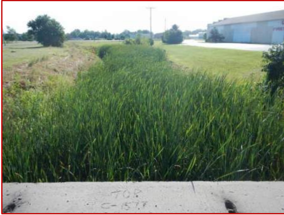
Photo 1: Looking east, east of I-65 northbound.
