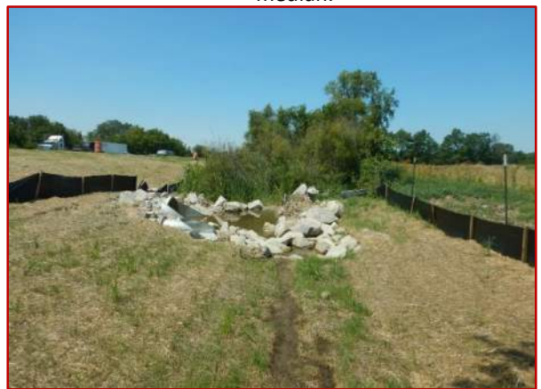
Photo 16: Looking northwest, east of I-65 northbound.
