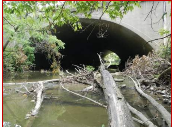
Photo 40: Looking northeast along Prairie Creek, west of I-65 southbound.
