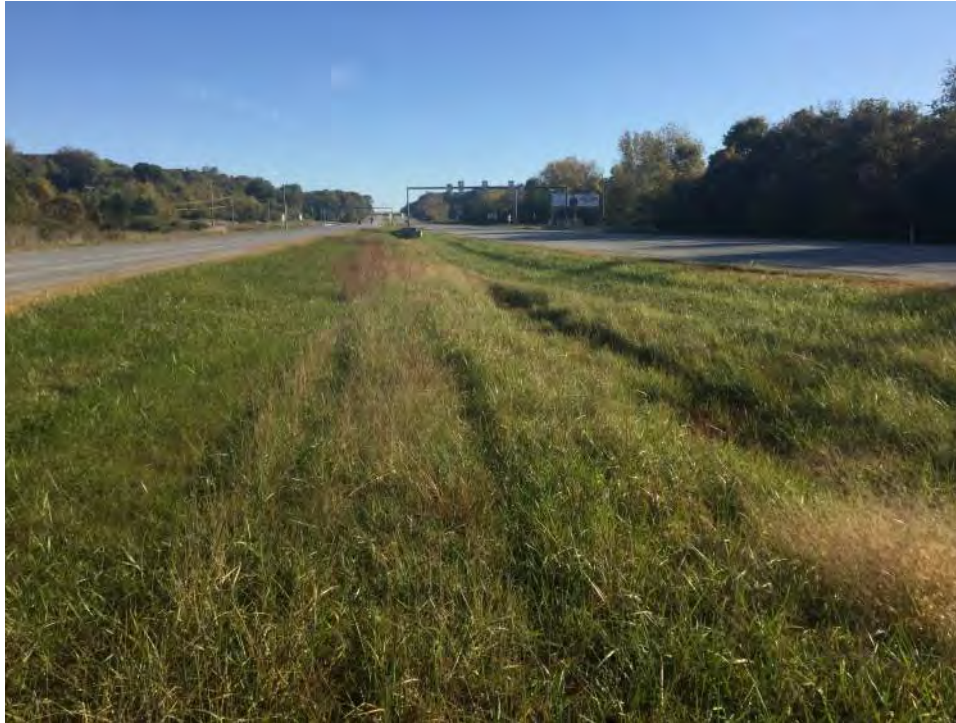
Photo 4: Facing northeast—view of RSD-6 within the US 24 median.
