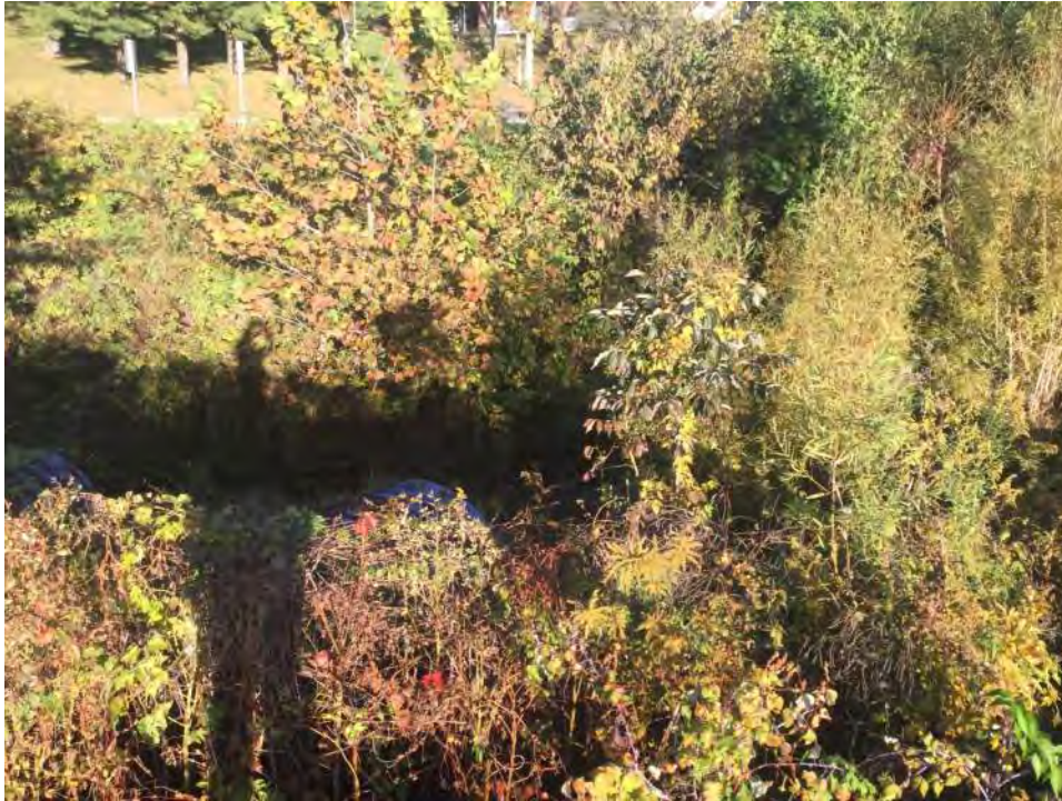
Photo 14: Facing northwest—view of upstream end of structures carrying Prairie Ditch beneath US 24.
