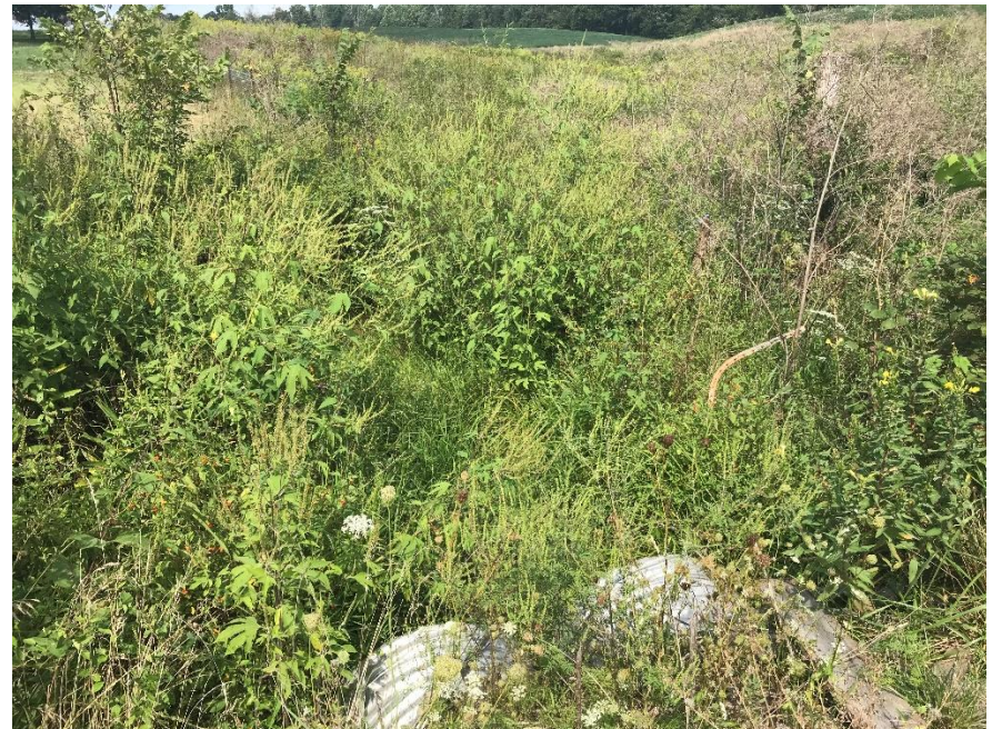
Photo 4. Project culvert outlet, facing north (9.3.2020).
