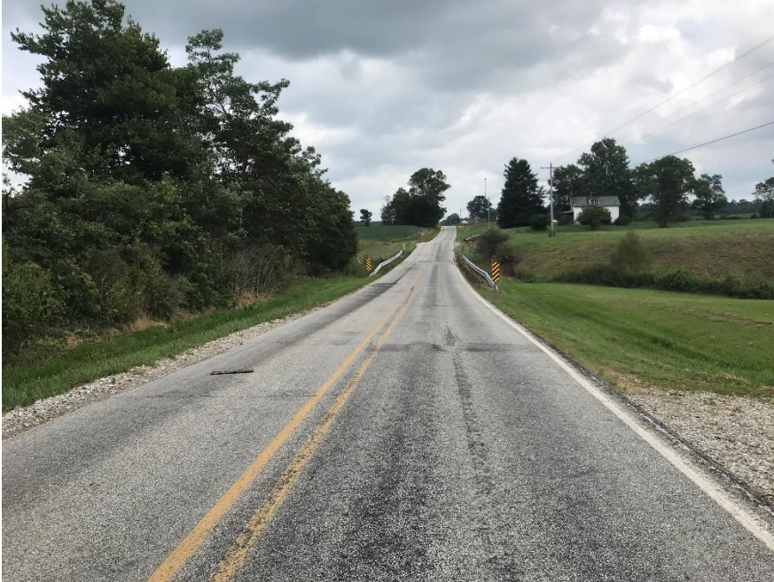
Photo 1. SR 250 approach roadway, facing east (9.3.2020).
