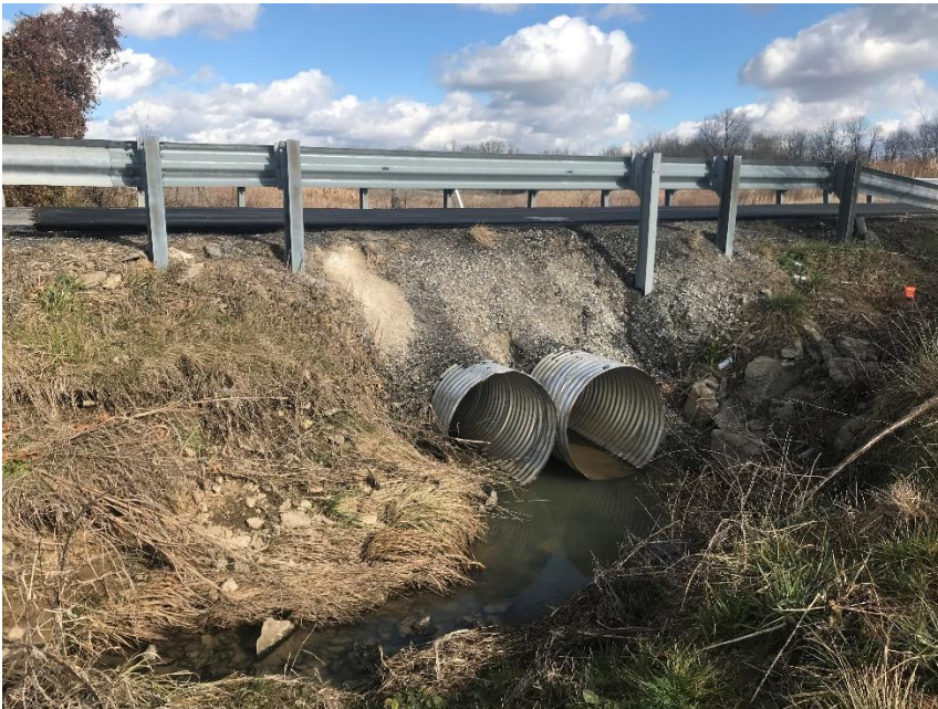
Photo 10. Project culvert outlet, facing northeast (1.15.2021).
