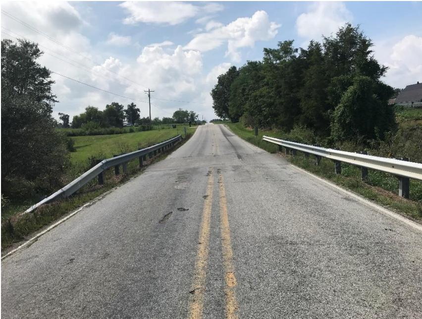
Photo 6. SR 250 approach roadway, facing west (9.3.2020).
