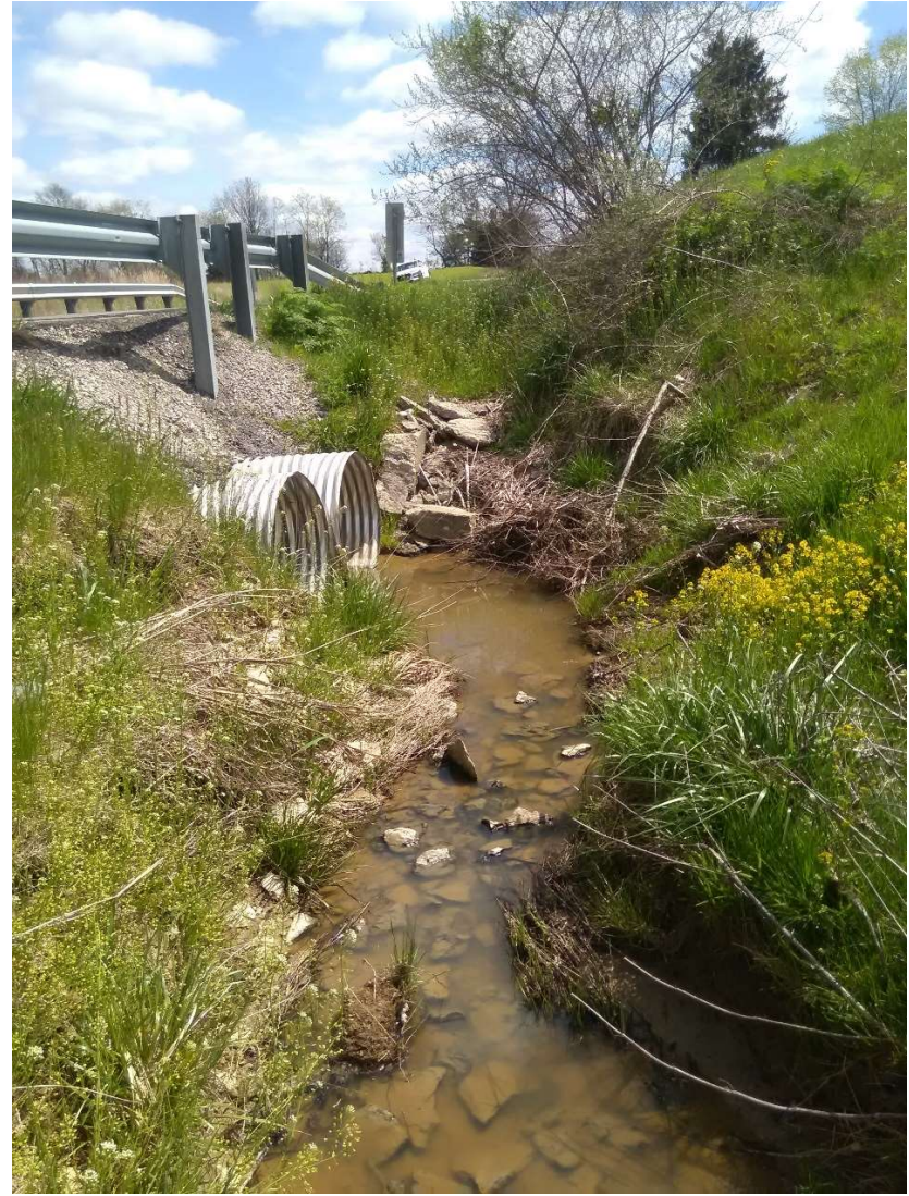
Photo 8. Facing east toward UNT 1 to Bear Branch and structure inlet. (4.16.21)
