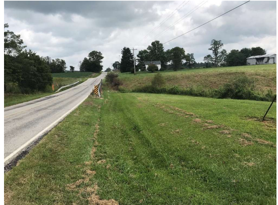
Photo 3. Facing east along south side SR 250 roadside toward project culvert. (9.3.20)
