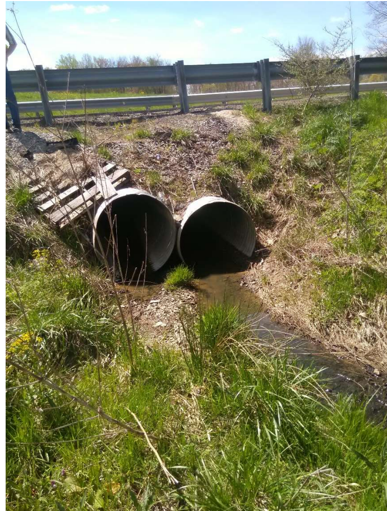
Photo 14. Facing south at UNT 1 to Bear Branch and structure outlet. (4.16.21)
