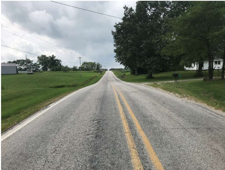
Photo 2. Facing west along SR 250 away from project culvert. (9.3.20)
