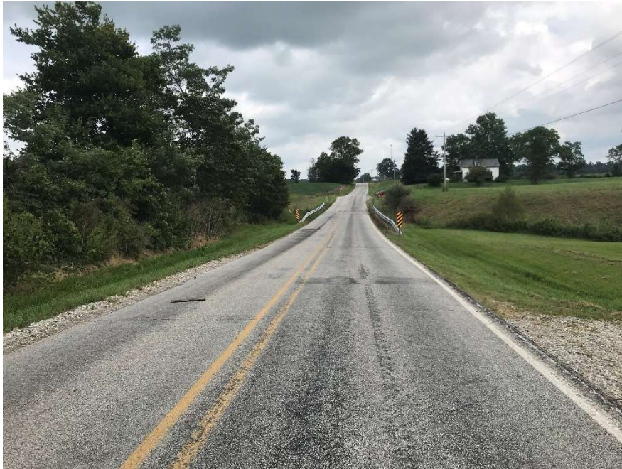
Photo 1. Facing east along SR 250 toward project culvert. (9.3.20)
