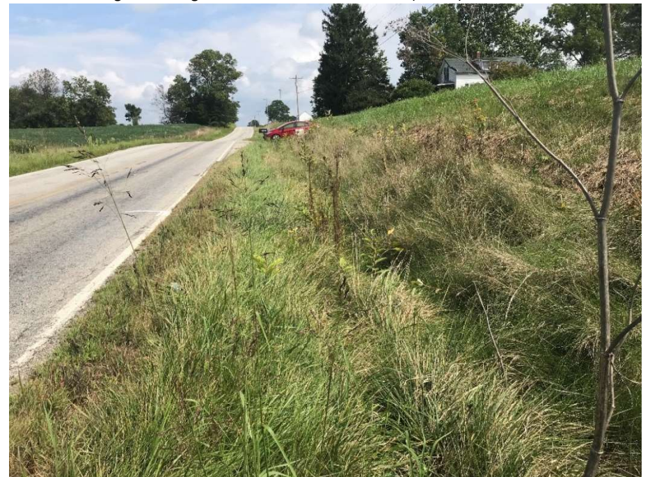
Photo 11. Facing east along south side of SR 250 away from project culvert. (9.3.20)
