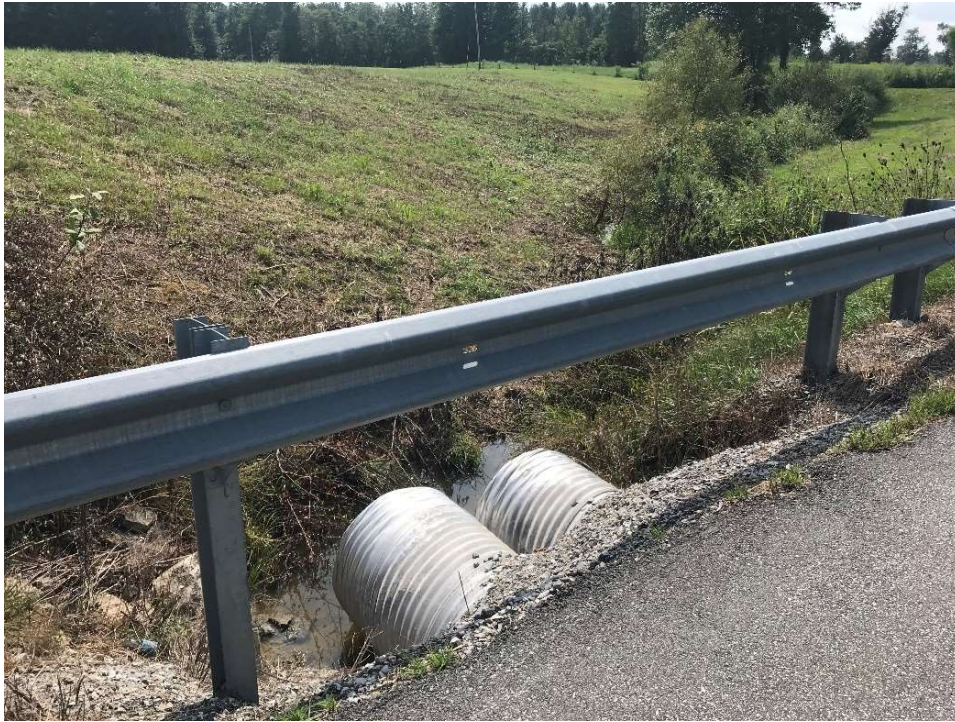
Photo 5. Facing southwest at culvert inlet from SR 250. (9.3.20)
