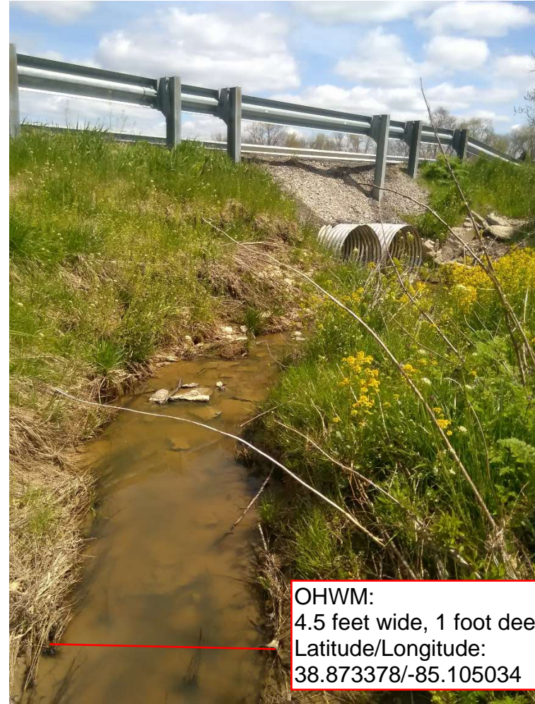
Photo 6. Facing northeast at UNT 1 to Bear Branch and structure inlet. (4.16.21)
