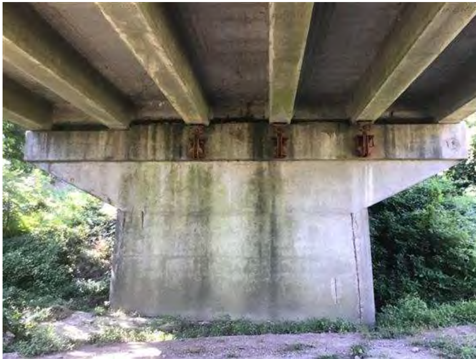
PHOTO 14 Condition Description Pier #2 facing South
