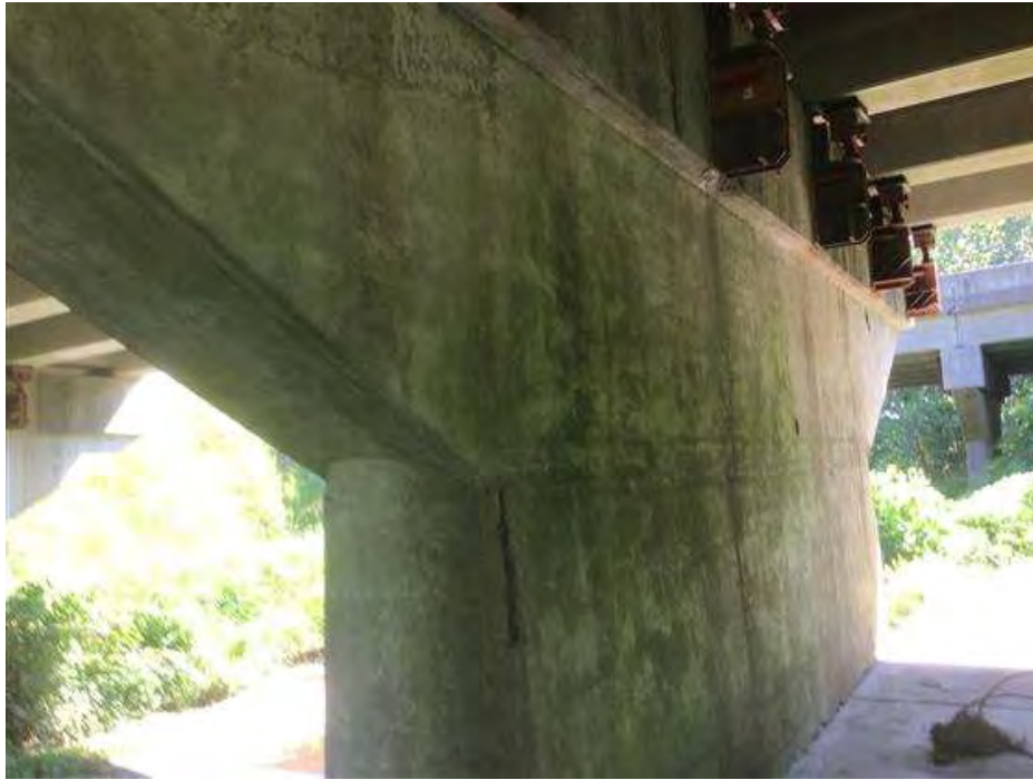
PHOTO 13 Condition Description Pier #2 facing Northeast
