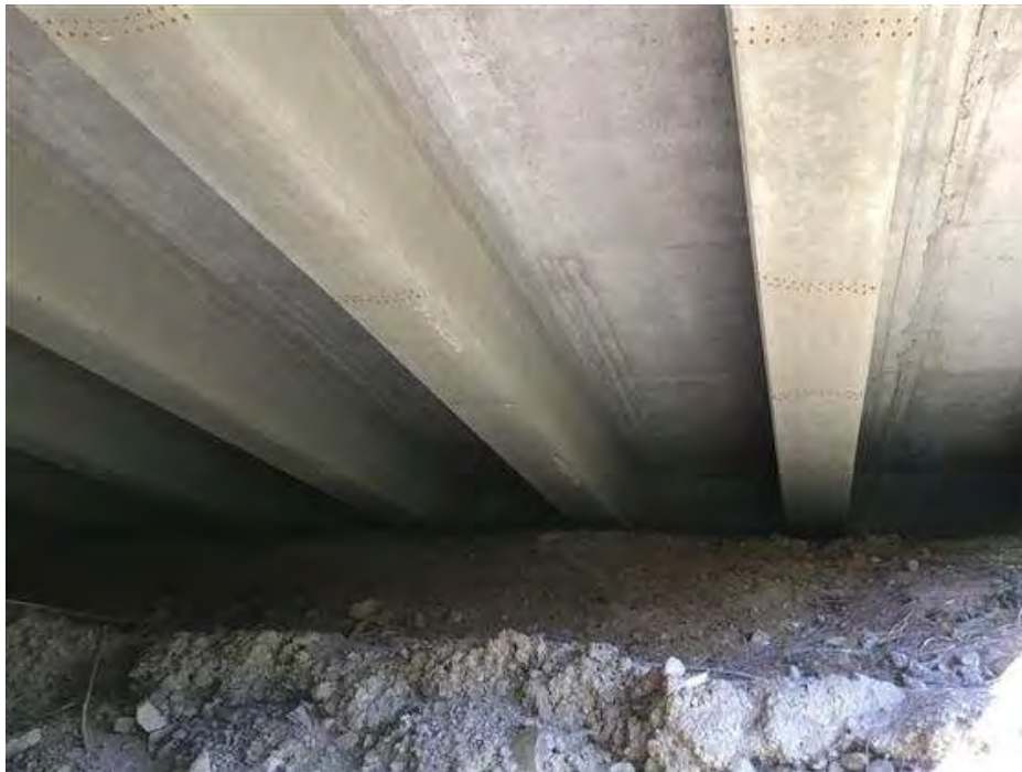
PHOTO 22 Condition Description Abutment #4 facing North
