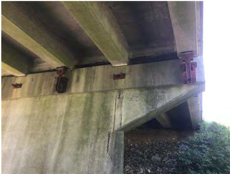
PHOTO 16 Condition Description Temporary Bearings on Pier #2 facing South
