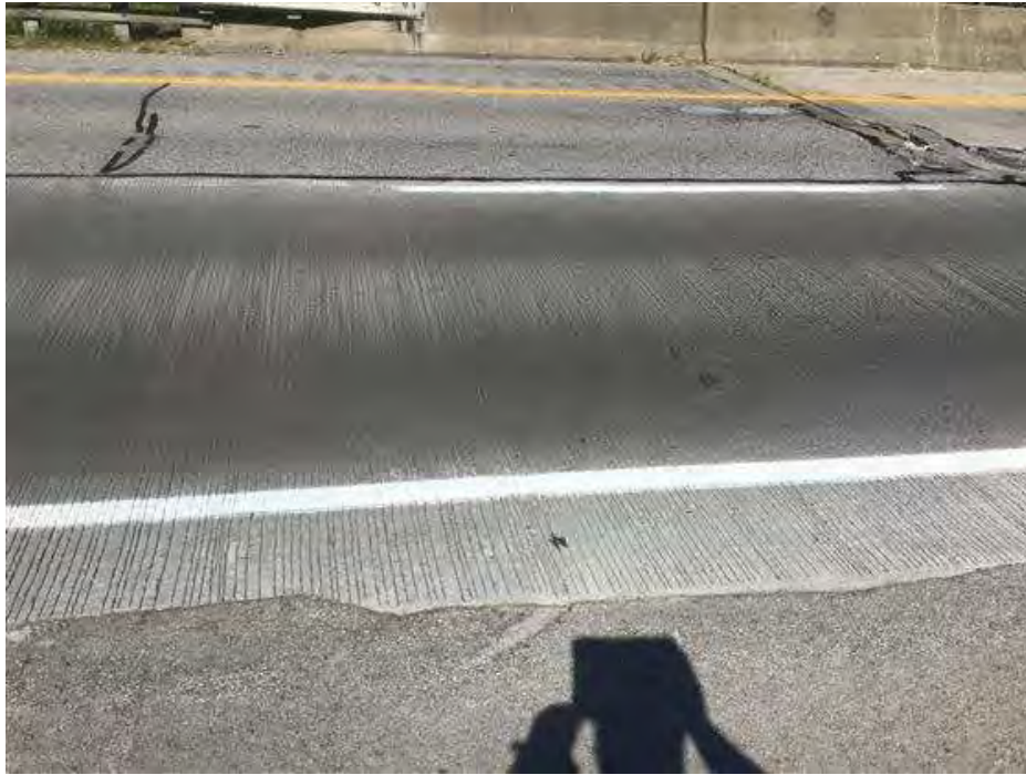
PHOTO 1 Condition Description South Approach facing West
