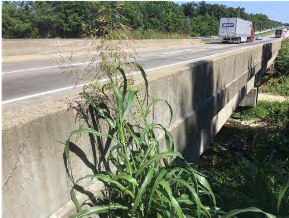
PHOTO 11 Elevation, Condition Description Side facing Northwest
