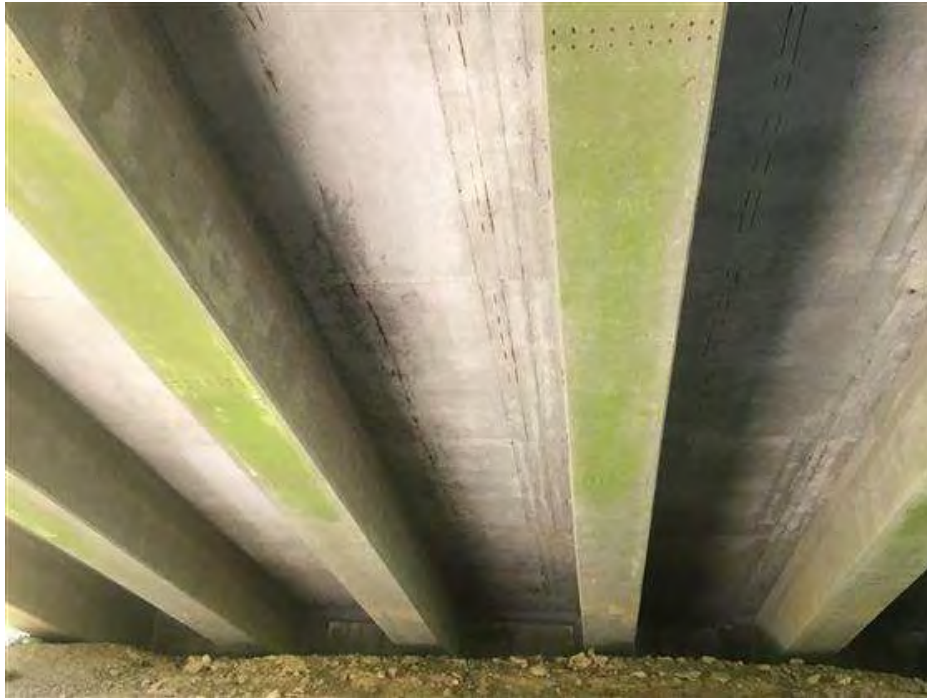
PHOTO 11 Condition Description Underside Span A and Abutment #1 facing South
