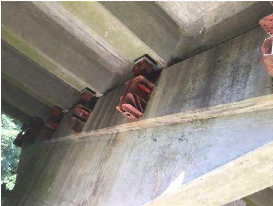
PHOTO 14 Condition Description Temporary Bearings on South Side Pier #2
