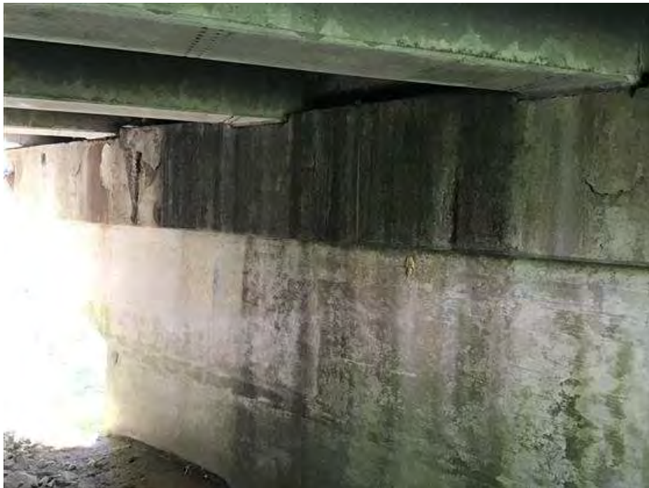
PHOTO 18 Condition Description Pier 3 north side.
