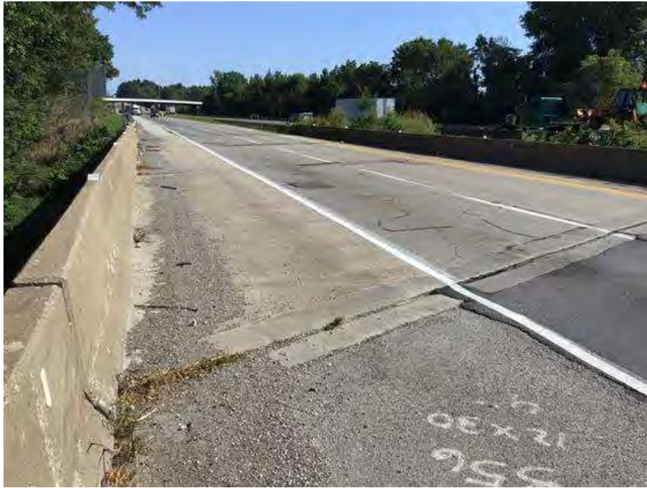
PHOTO 3 Condition Description Roadway north.
