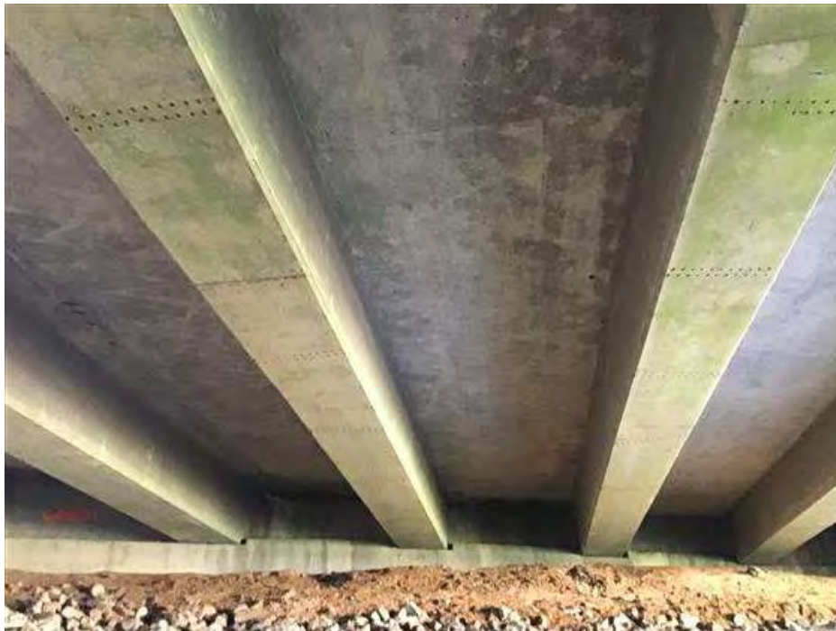
PHOTO 10 Condition Description Span A facing south.
