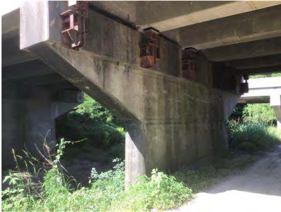
PHOTO 17 Condition Description Pier #3 facing Southwest
