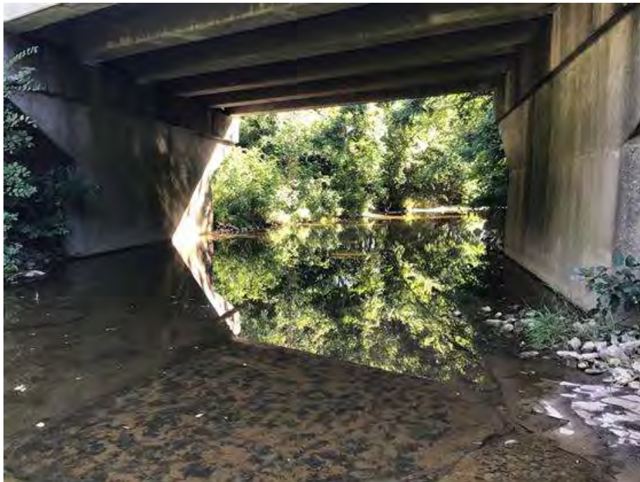
PHOTO 20 Condition Description Channel facing east.
