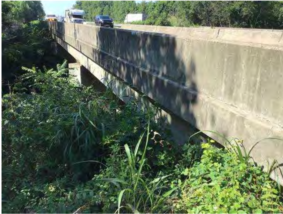
PHOTO 1 Elevation, Condition Description East side.
