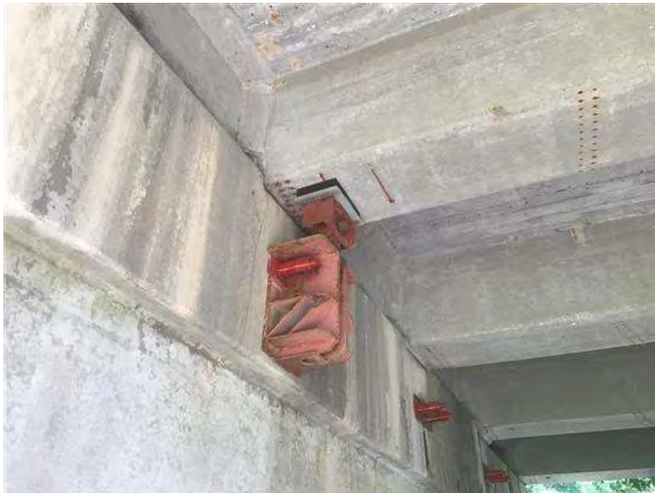
PHOTO 20 Condition Description Temporary Bearing on Pier #3
