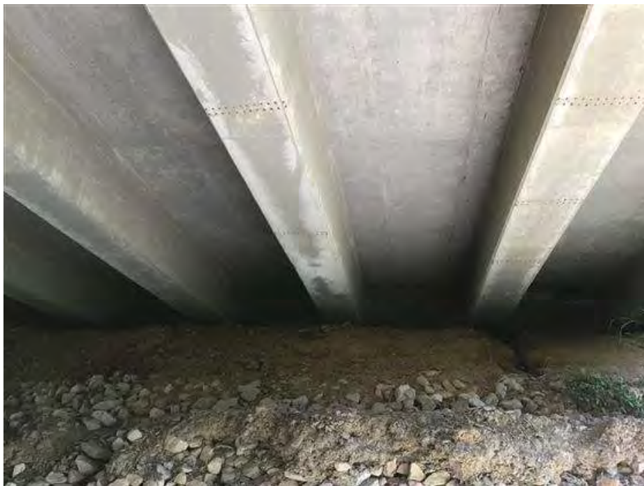
PHOTO 20 Condition Description Abutment #4 facing North
