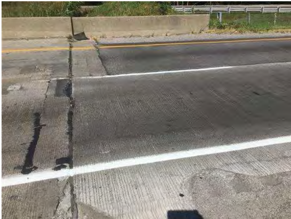
PHOTO 10 Condition Description North Approach facing West
