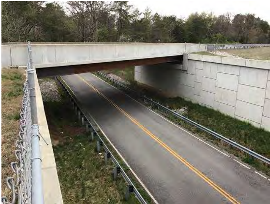
PHOTO 2 Elevation, Condition Description East side.
