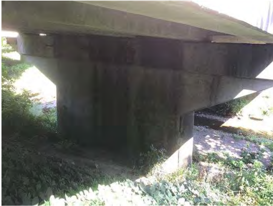
PHOTO 13 Condition Description Pier #2 facing North
