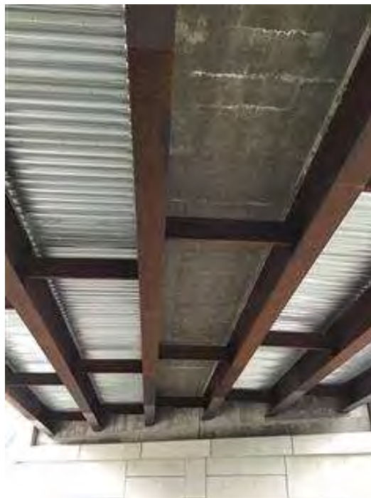
PHOTO 8 Condition Description Underside and south abutment.
