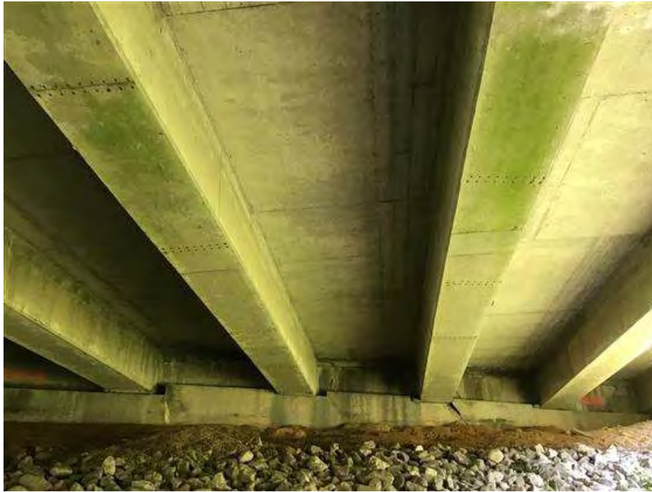
PHOTO 13 Condition Description Span C facing north.
