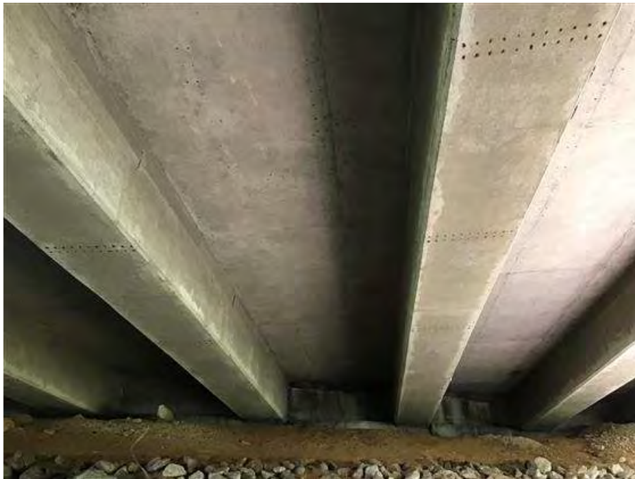
PHOTO 12 Condition Description Span C facing north.
