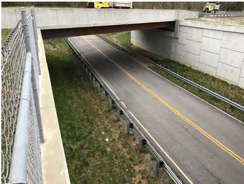
PHOTO 2 Condition Description West side.
