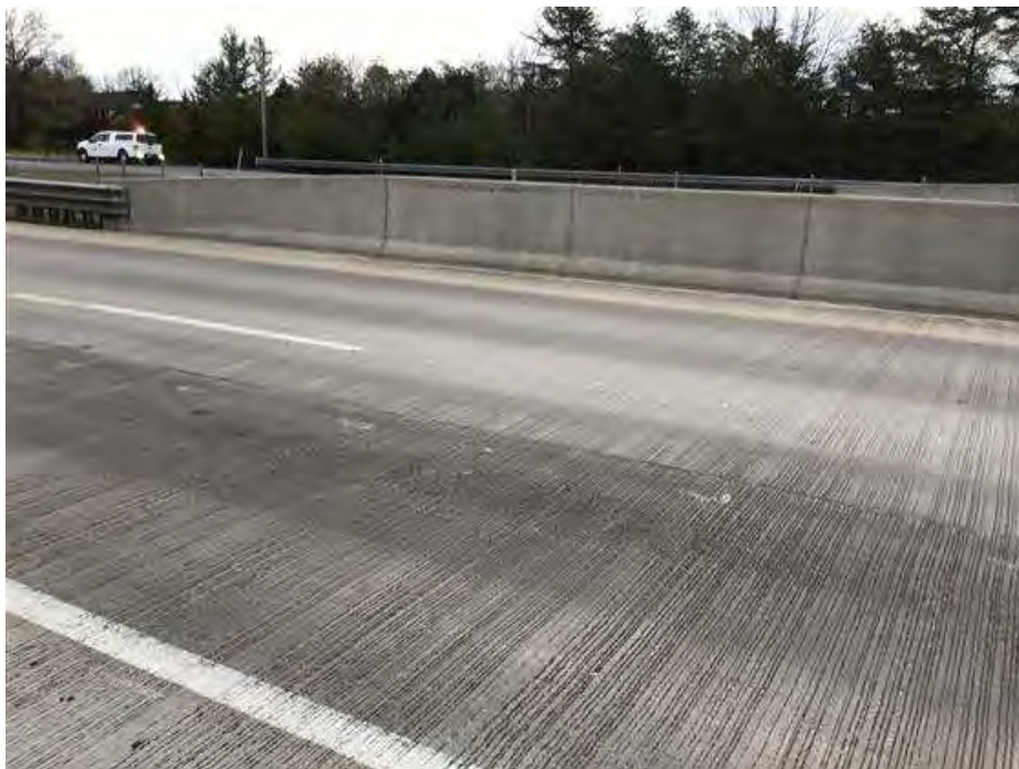
PHOTO 6 Condition Description East barrier wall.
