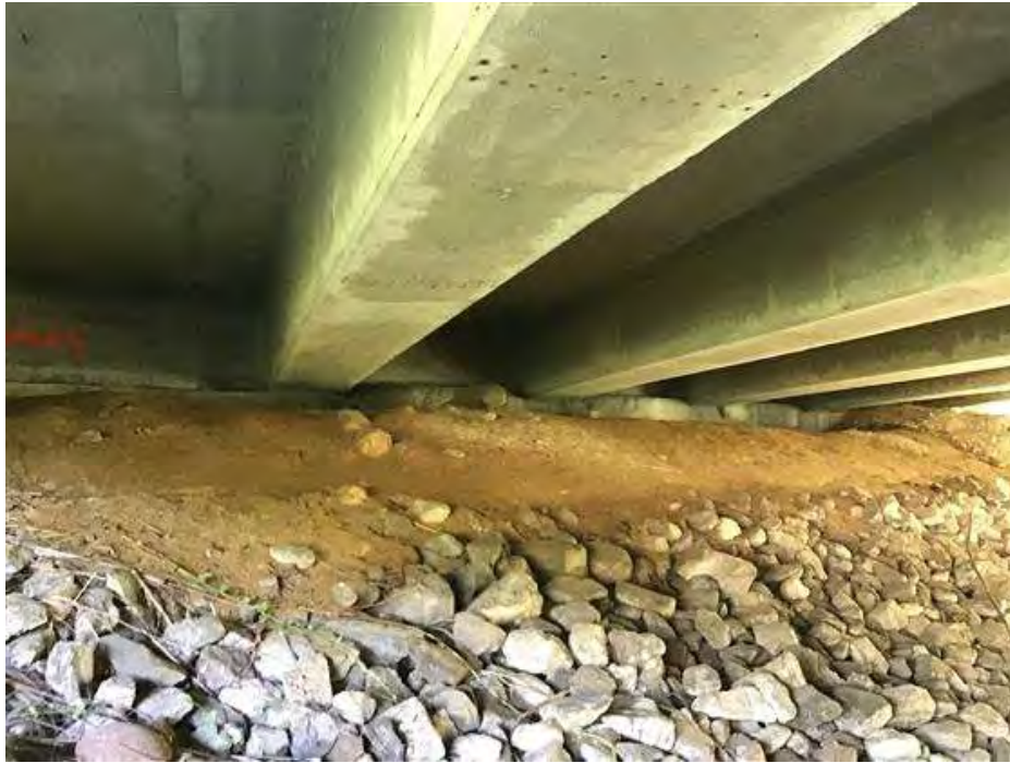
PHOTO 19 Condition Description North abutment.
