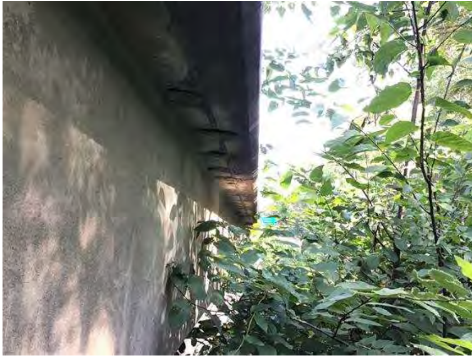
PHOTO 9 Condition Description West coping.
