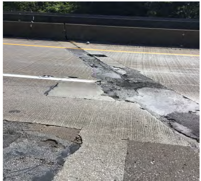
PHOTO 2 Description Joint 3 facing east.
