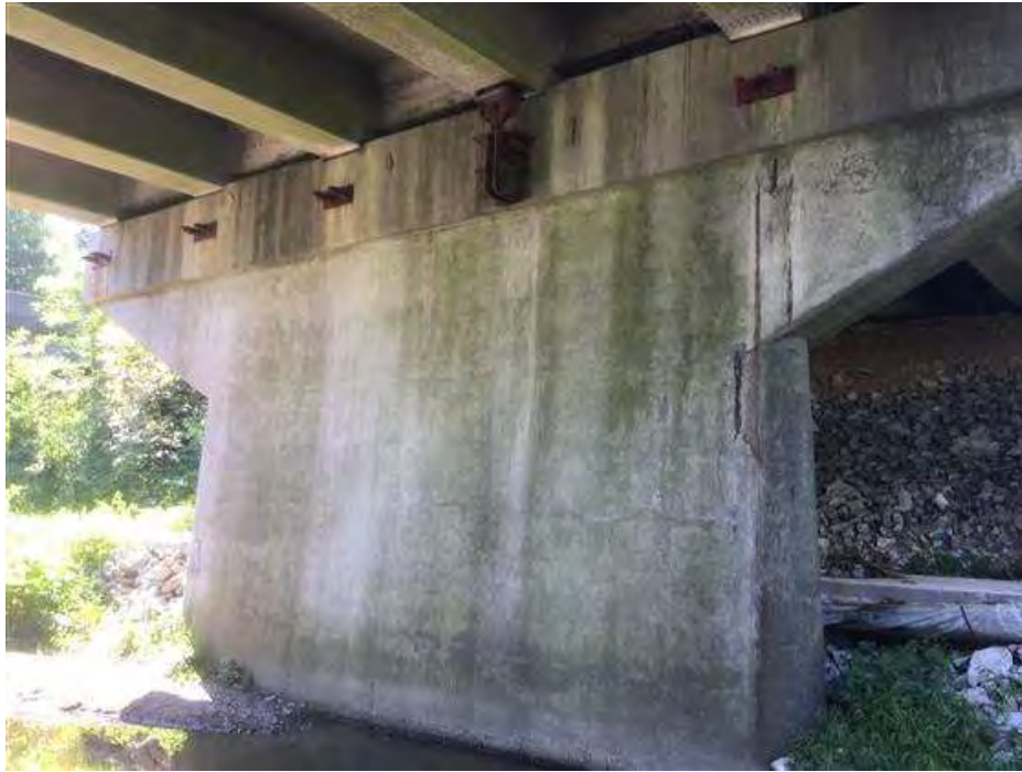
PHOTO 15 Condition Description Pier #2 facing South
