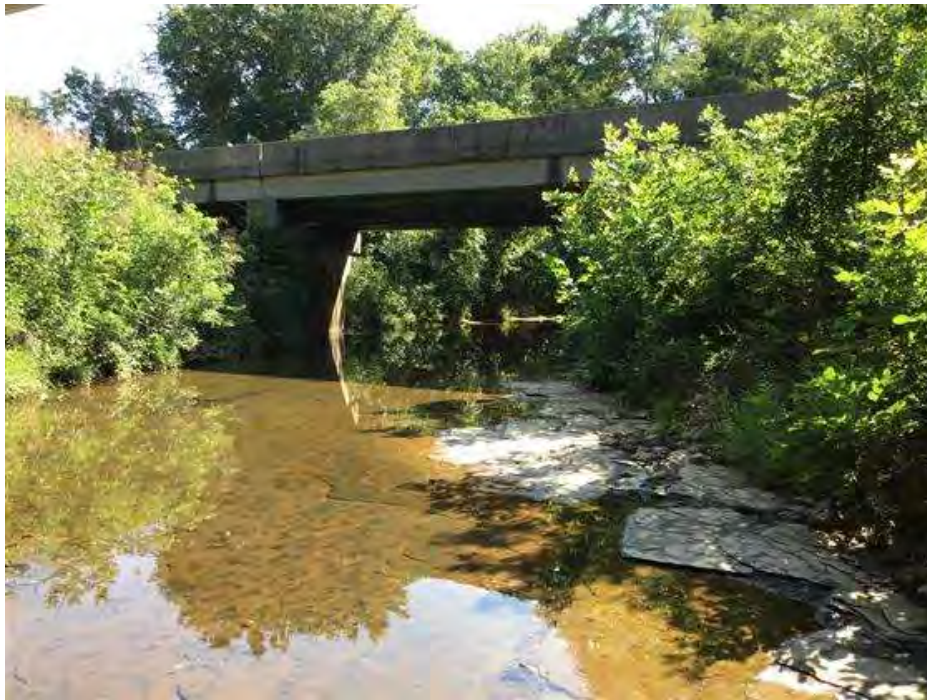
PHOTO 2 Elevation, Condition Description West side.
