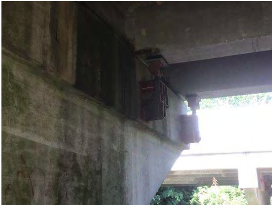
PHOTO 18 Condition Description Temporary Bearings on Pier #3
