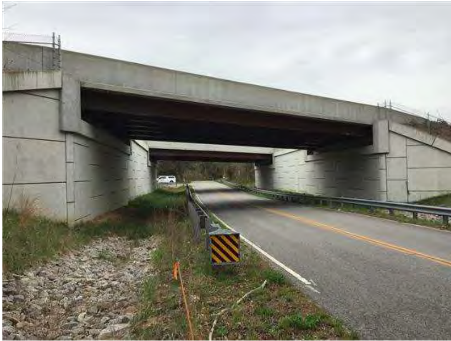
PHOTO 1 Elevation, Condition Description West side.
