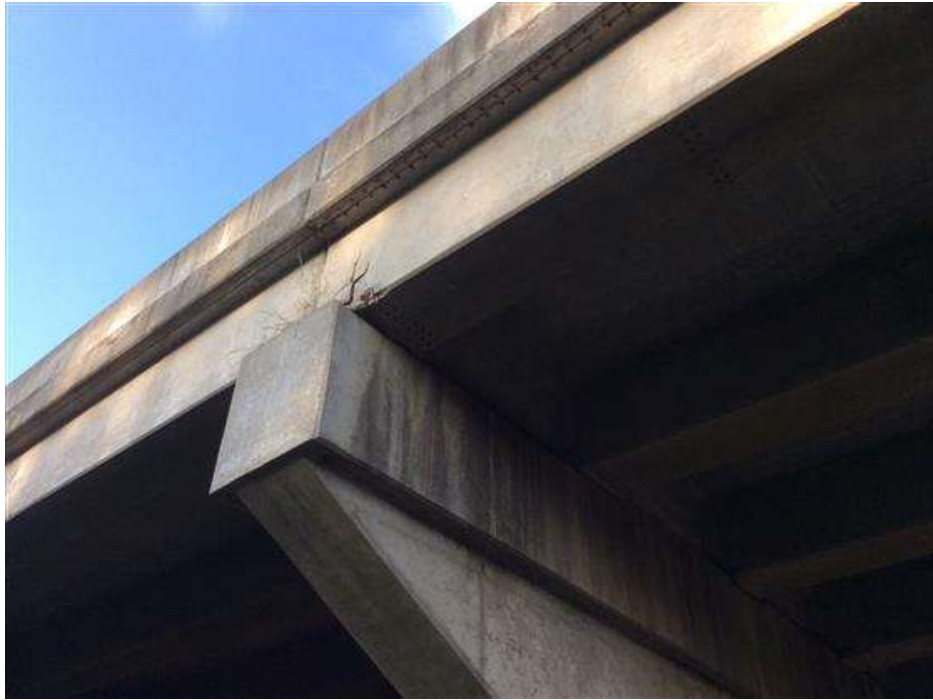
PHOTO 25 Condition Description South end beam 6 at pier 2 span b.
