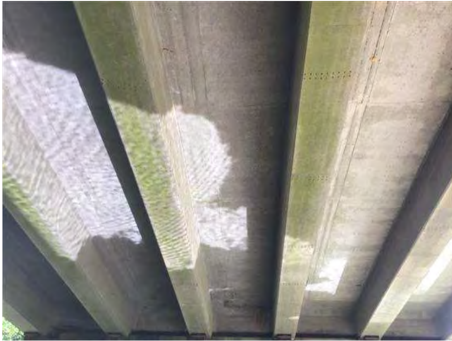
PHOTO 17 Condition Description Underside Span B facing North
