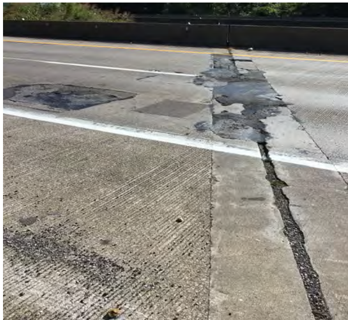
PHOTO 1 Description Joint 3 facing east.
