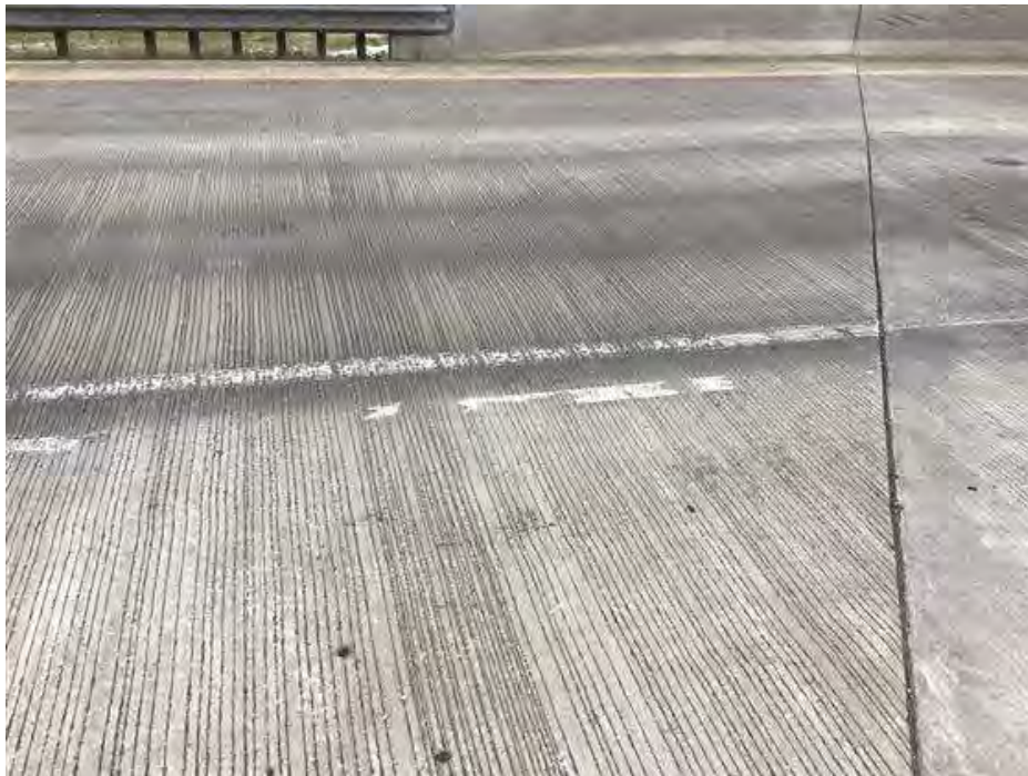
PHOTO 4 Condition Description South joint and approach slab.
