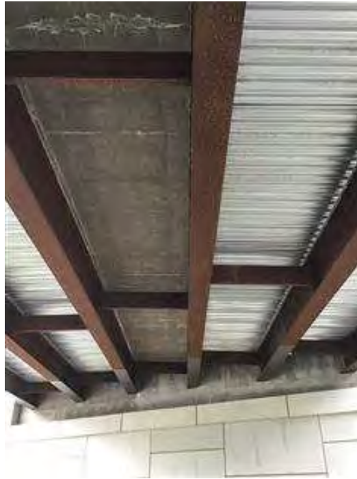
PHOTO 7 Condition Description Underside and north abutment.
