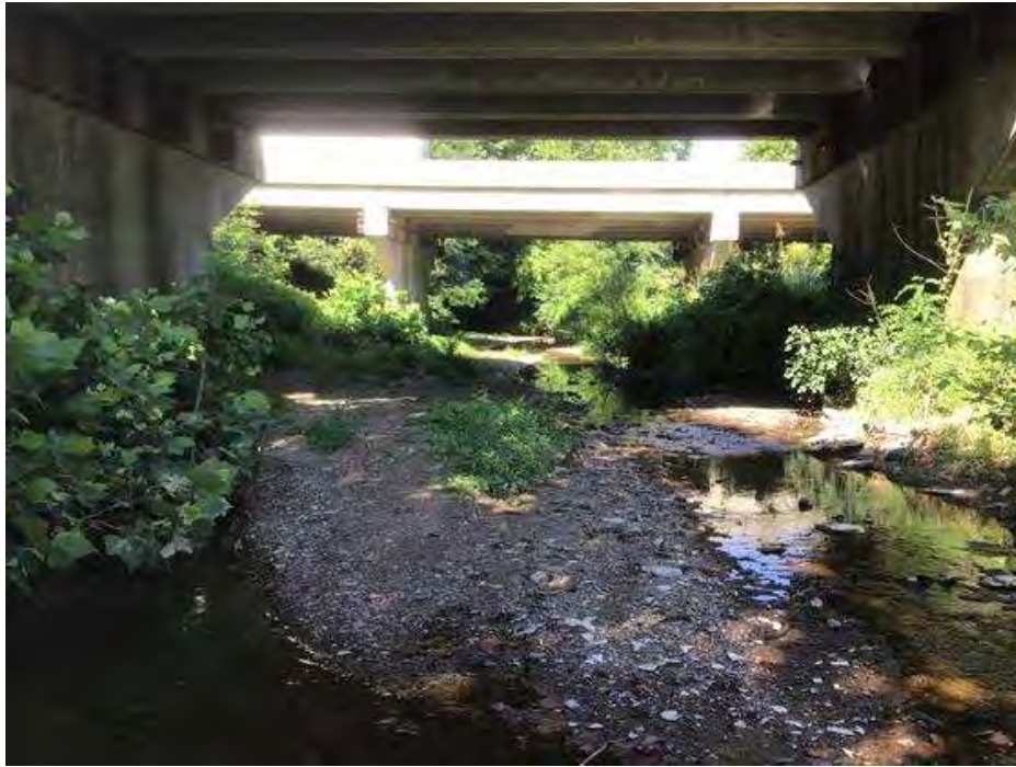
PHOTO 21 Condition Description Channel facing West
