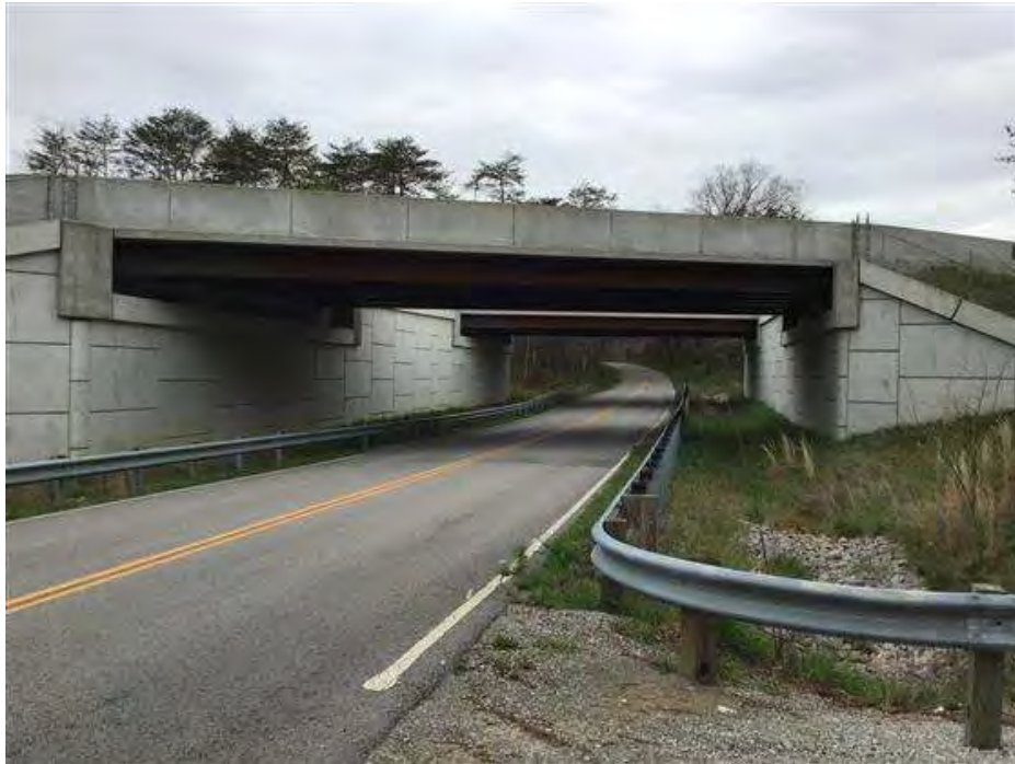
PHOTO 1 Elevation, Condition Description East side.
