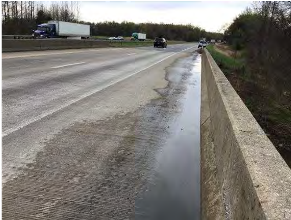
PHOTO 4 Condition Description Roadway north.
