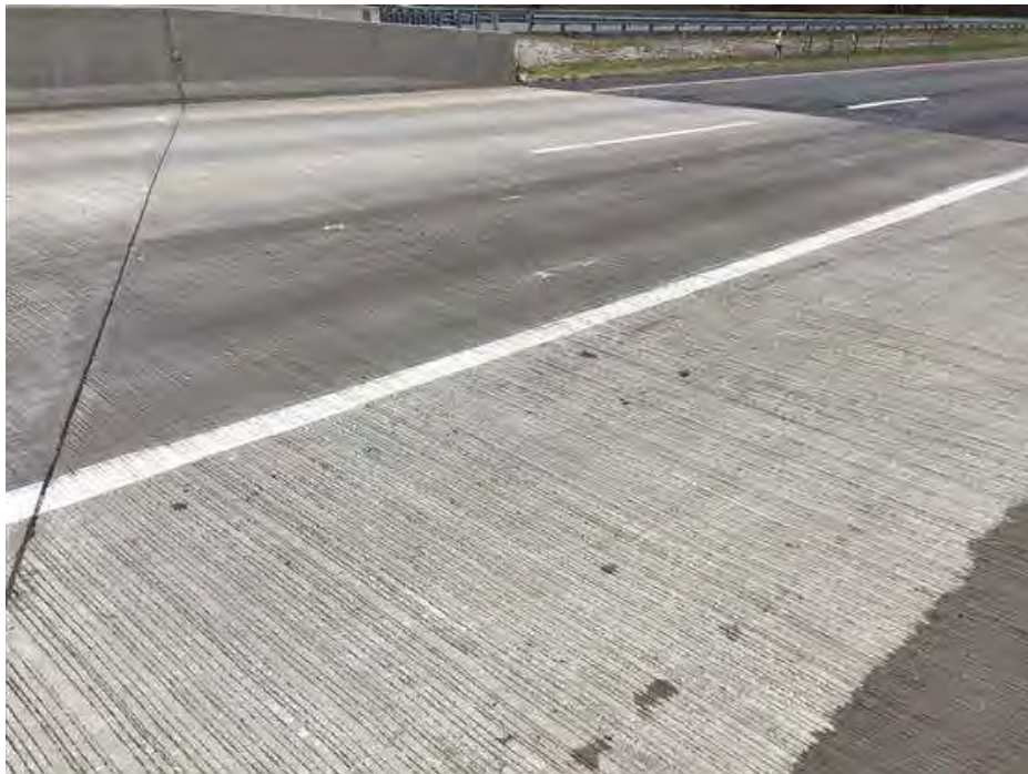
PHOTO 4 Condition Description South joint and approach slab.
