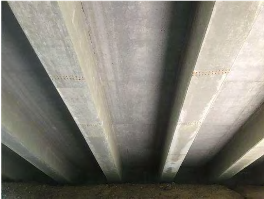
PHOTO 19 Condition Description Underside Span C facing North
