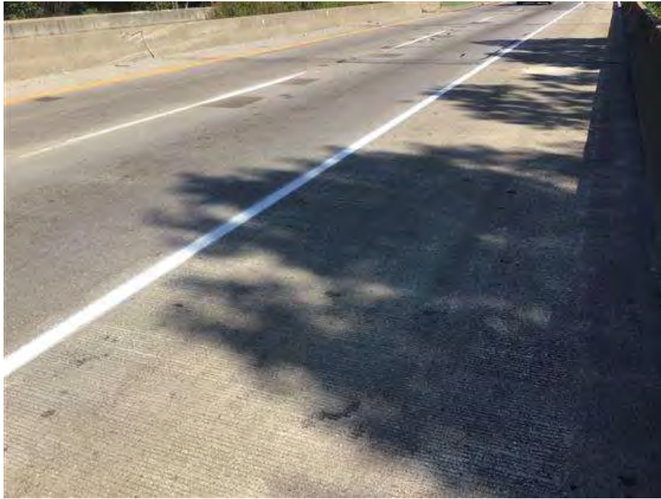
PHOTO 3 Condition Description Deck facing North
