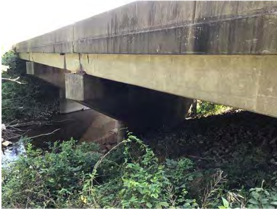
PHOTO 1 Elevation, Condition Description West side.
