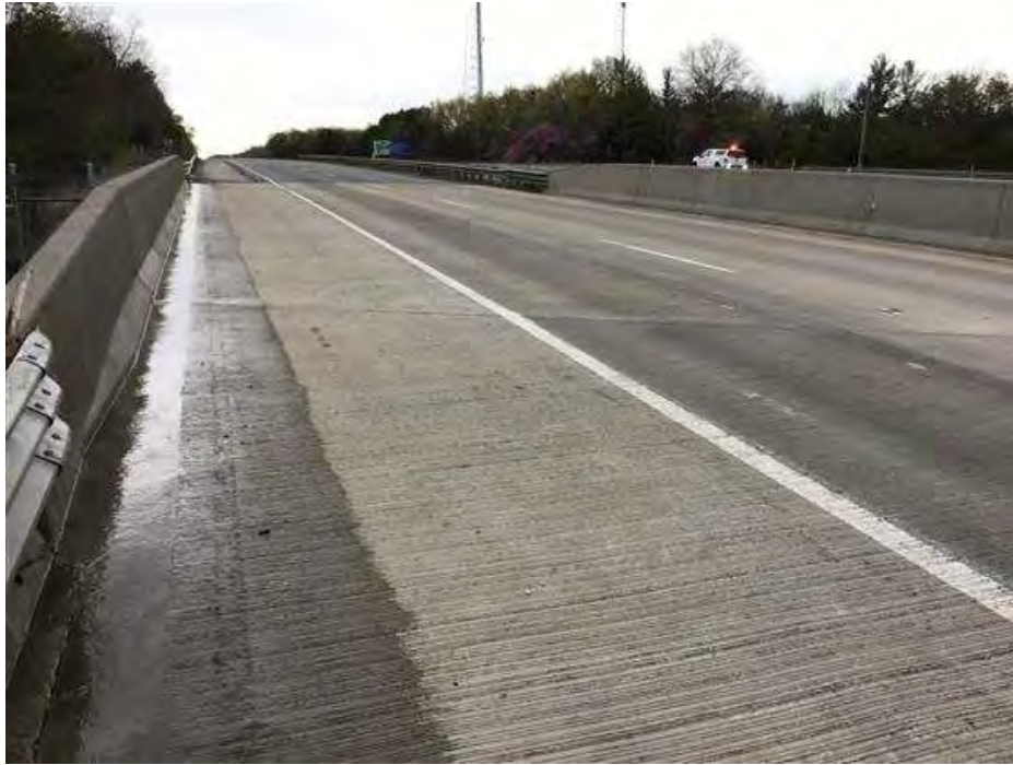
PHOTO 3 Condition Description Roadway north.
