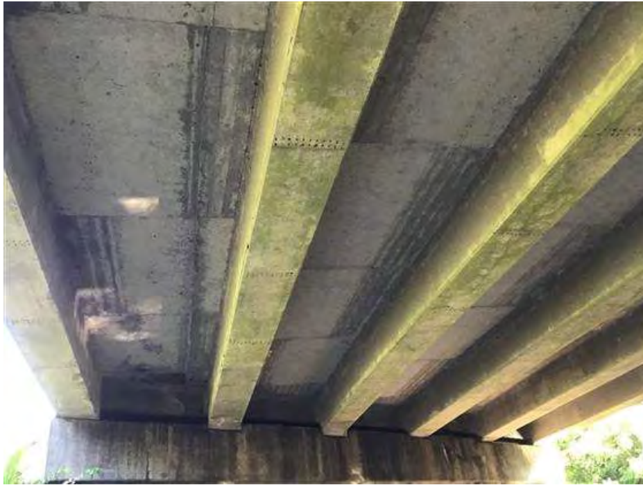
PHOTO 11 Condition Description Span B facing north.
