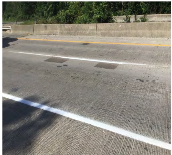
PHOTO 2 Description Patches over Span A
