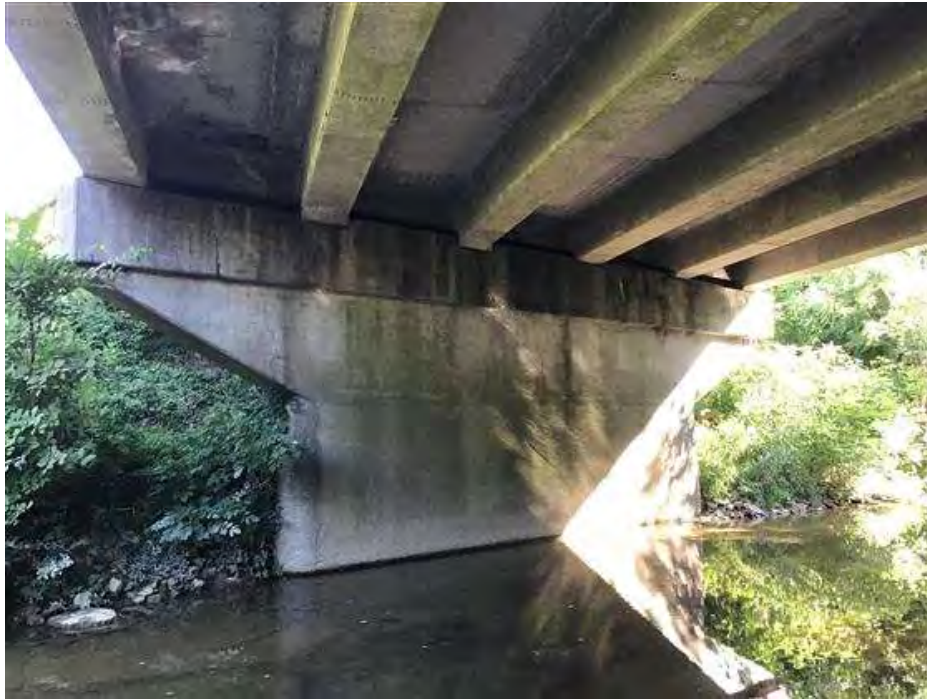
PHOTO 17 Condition Description Pier 3 south side.
