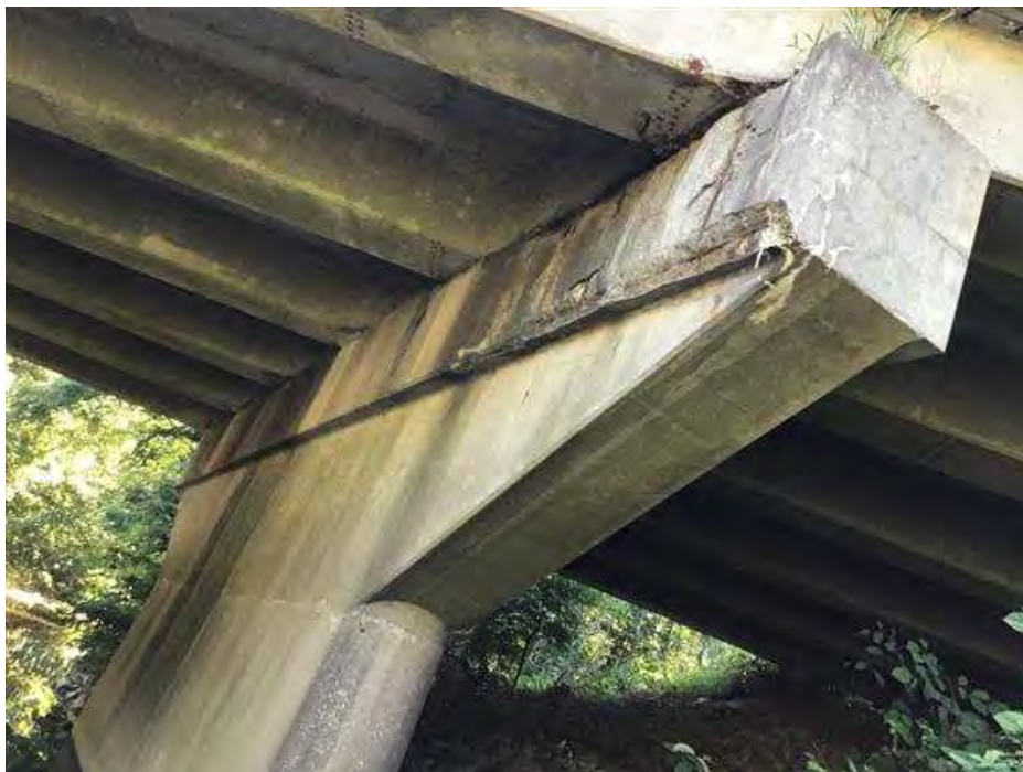
PHOTO 16 Condition Description Pier 2 north side, west nose.
