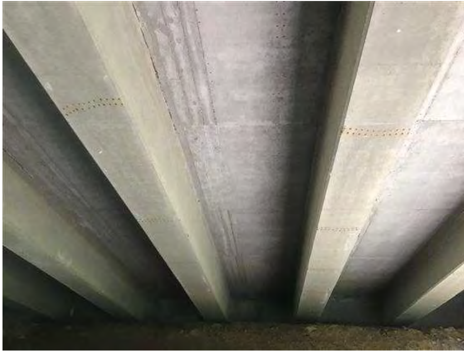
PHOTO 21 Condition Description Underside Span C facing North
