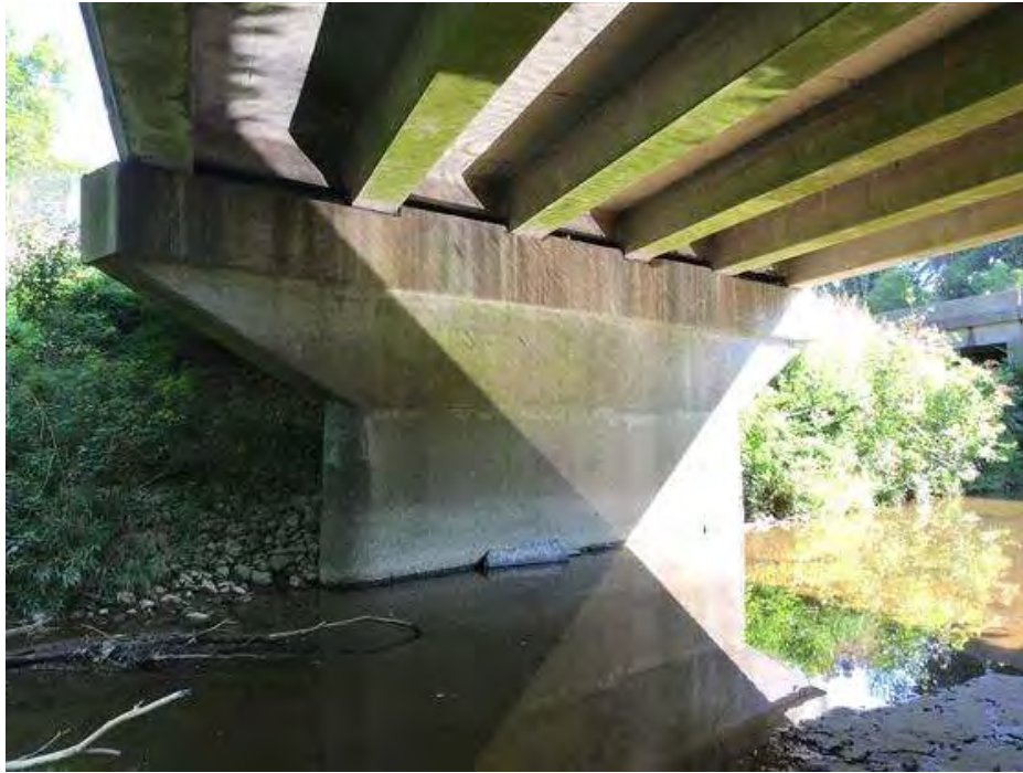
PHOTO 17 Condition Description Pier 3 south side.
