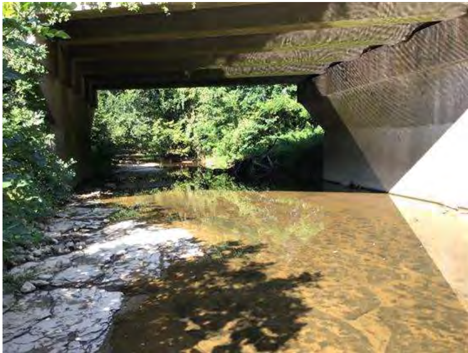
PHOTO 20 Condition Description Channel facing west.
