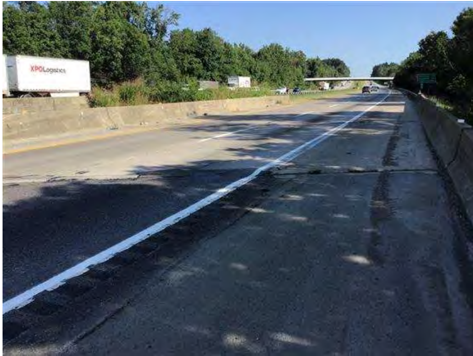
PHOTO 3 Condition Description Roadway north.
