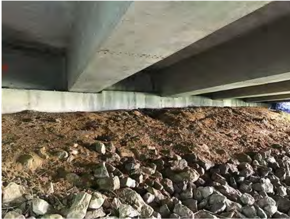
PHOTO 13 Condition Description South abutment.
