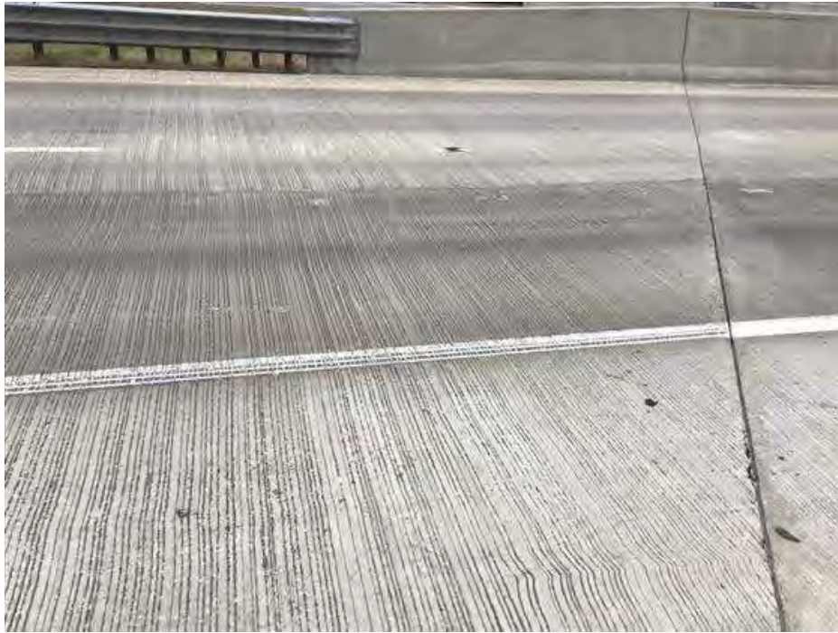
PHOTO 5 Condition Description North joint and approach slab.
