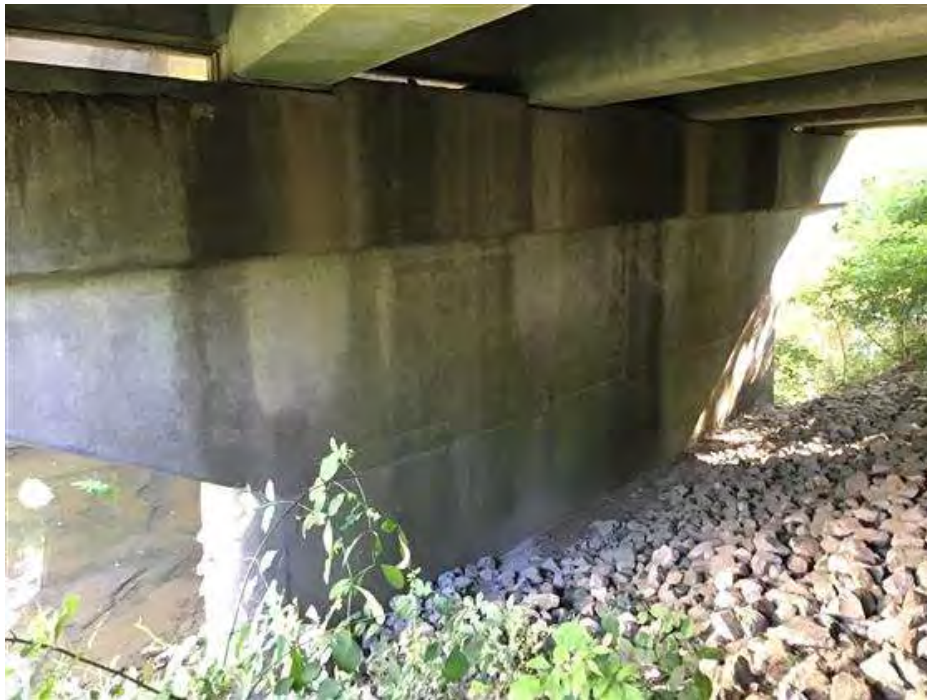
PHOTO 14 Condition Description Pier 2 south side.
