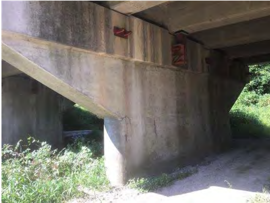
PHOTO 19 Condition Description Pier #3 facing Southwest
