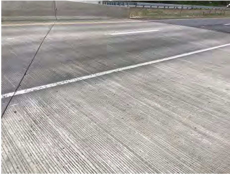
PHOTO 5 Condition Description North joint and approach slab.
