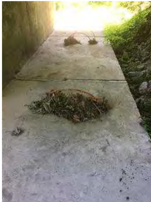
PHOTO 12 Condition Description Concrete Pad at South Side Pier #2 facing East
