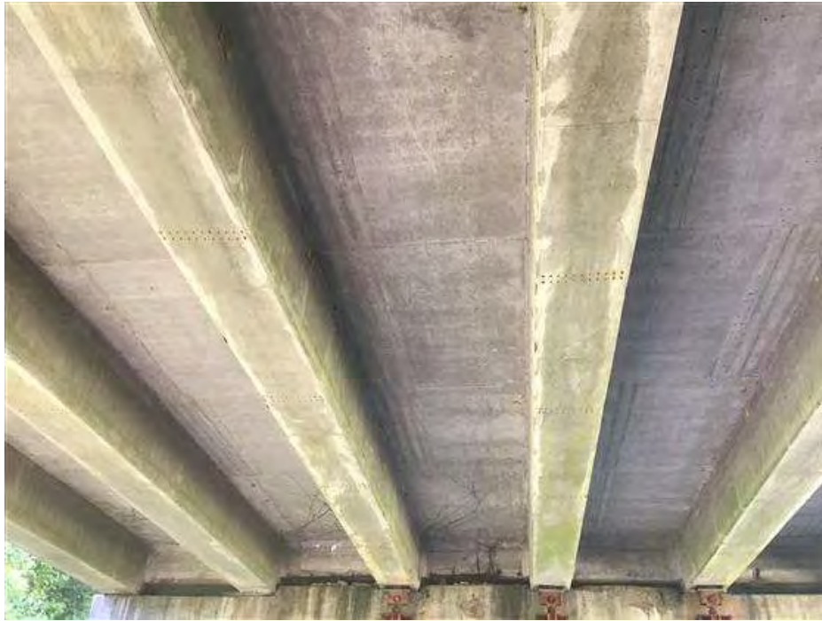
PHOTO 15 Condition Description Underside Span B facing South
