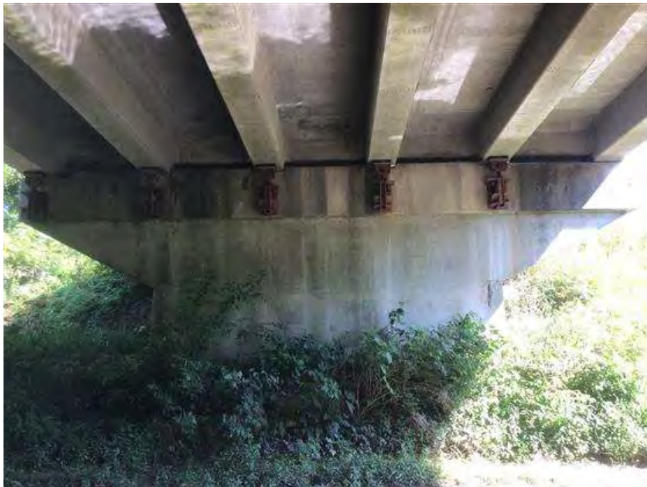
PHOTO 18 Condition Description Pier #3 facing North
