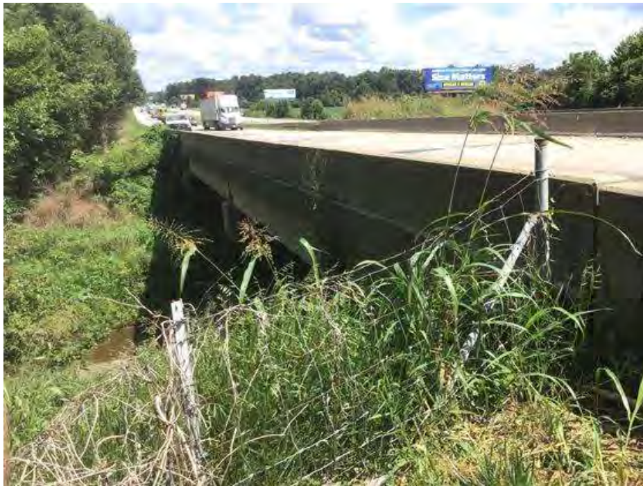
PHOTO 10 Elevation, Condition Description Side facing Northeast
