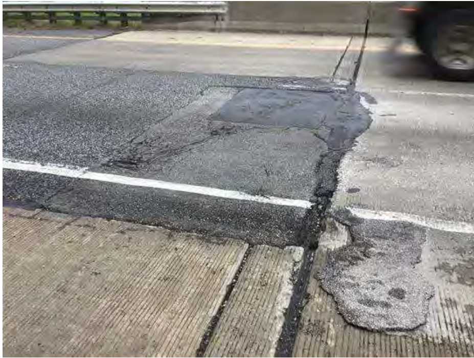
PHOTO 5 Condition Description South joint and approach slab.
