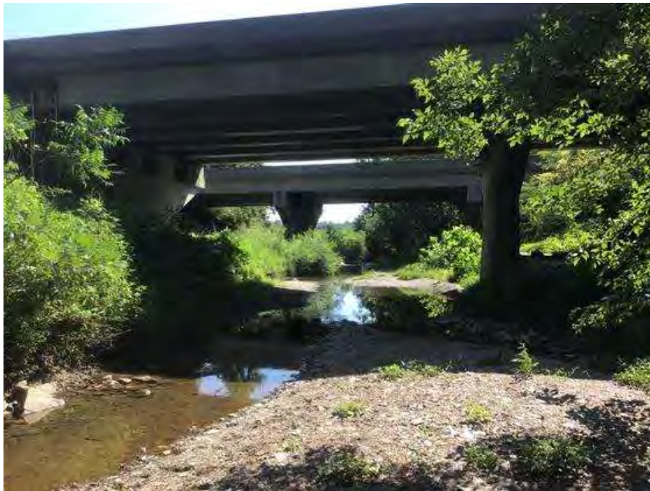
PHOTO 22 Condition Description Channel facing East
