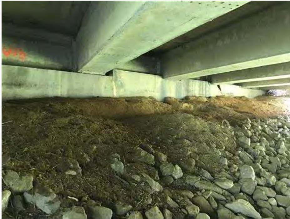
PHOTO 19 Condition Description North abutment.
