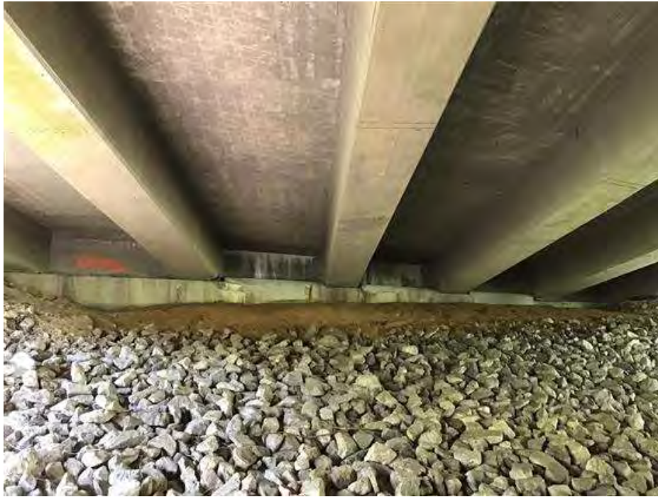
PHOTO 15 Condition Description South abutment.
