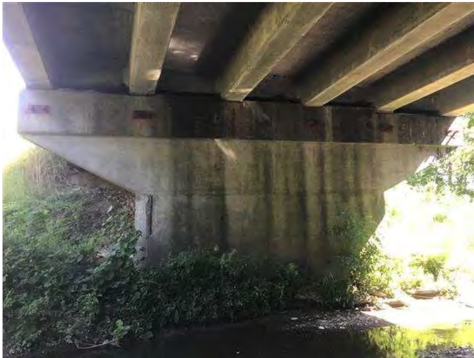
PHOTO 16 Condition Description Pier #3 facing North
