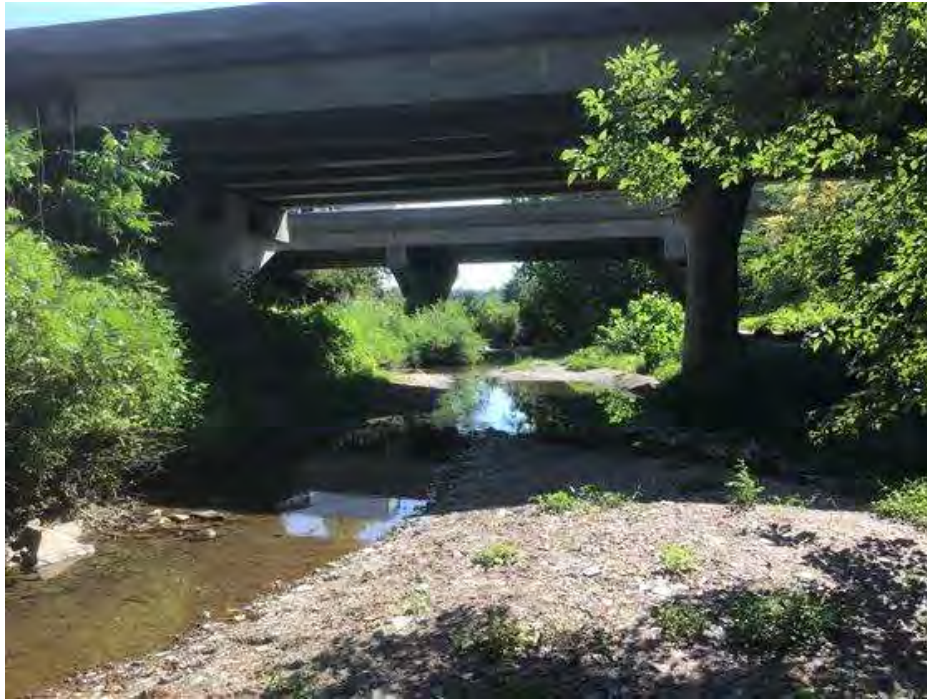
PHOTO 23 Condition Description Channel facing East
