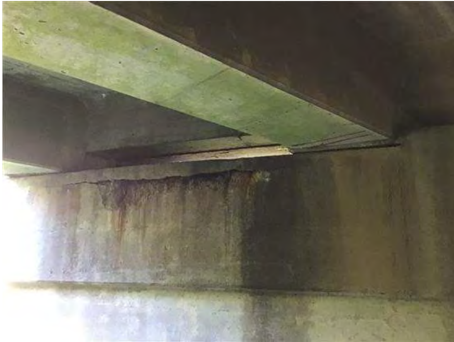
PHOTO 15 Condition Description Pier 2 south side, west nose.
