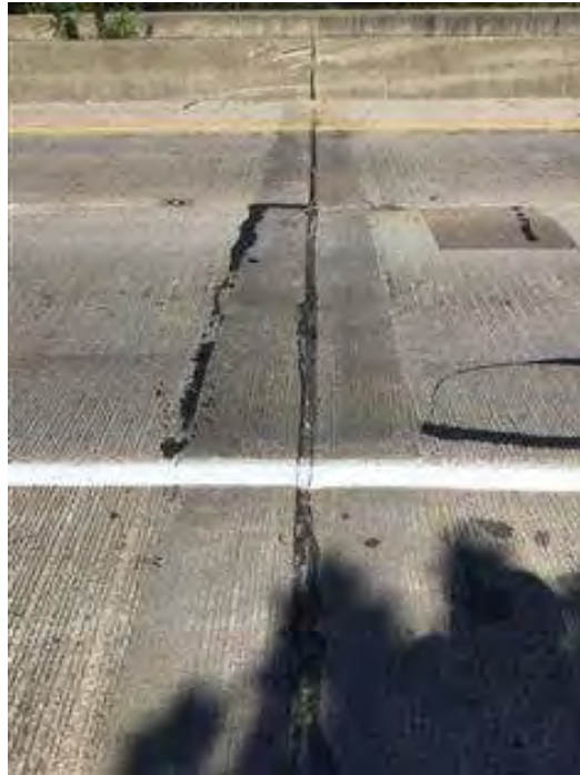
PHOTO 5 Condition Description Joint over Pier #2 facing West
