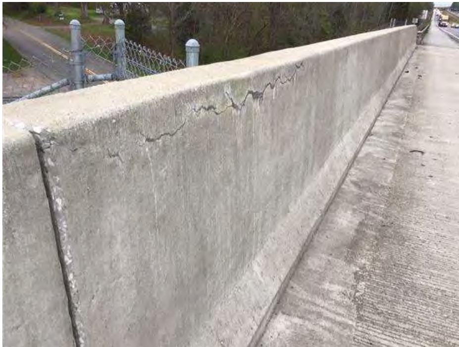
PHOTO 6 Condition Description East barrier wall.
