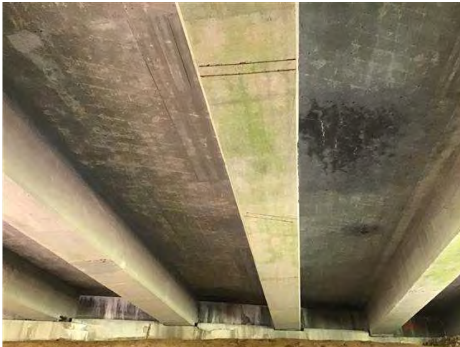
PHOTO 10 Condition Description Span A facing south.
