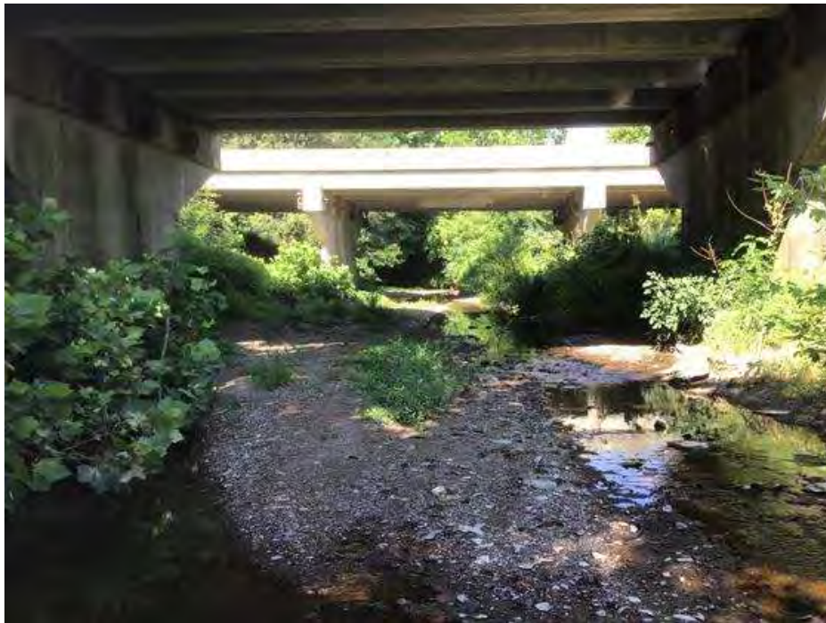
PHOTO 24 Elevation, Condition Description Channel facing West
