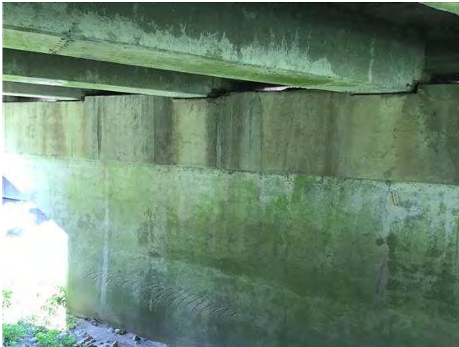
PHOTO 18 Condition Description Pier 3 north side.
