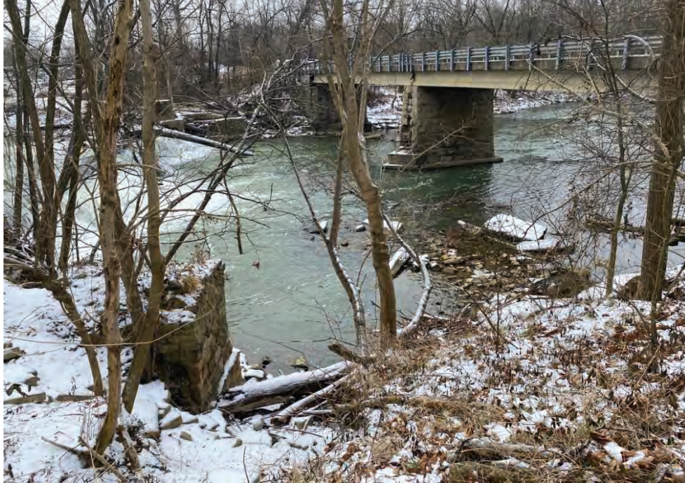
Photo 25. View overlooking former mill site facing south toward Bridge No. 51
