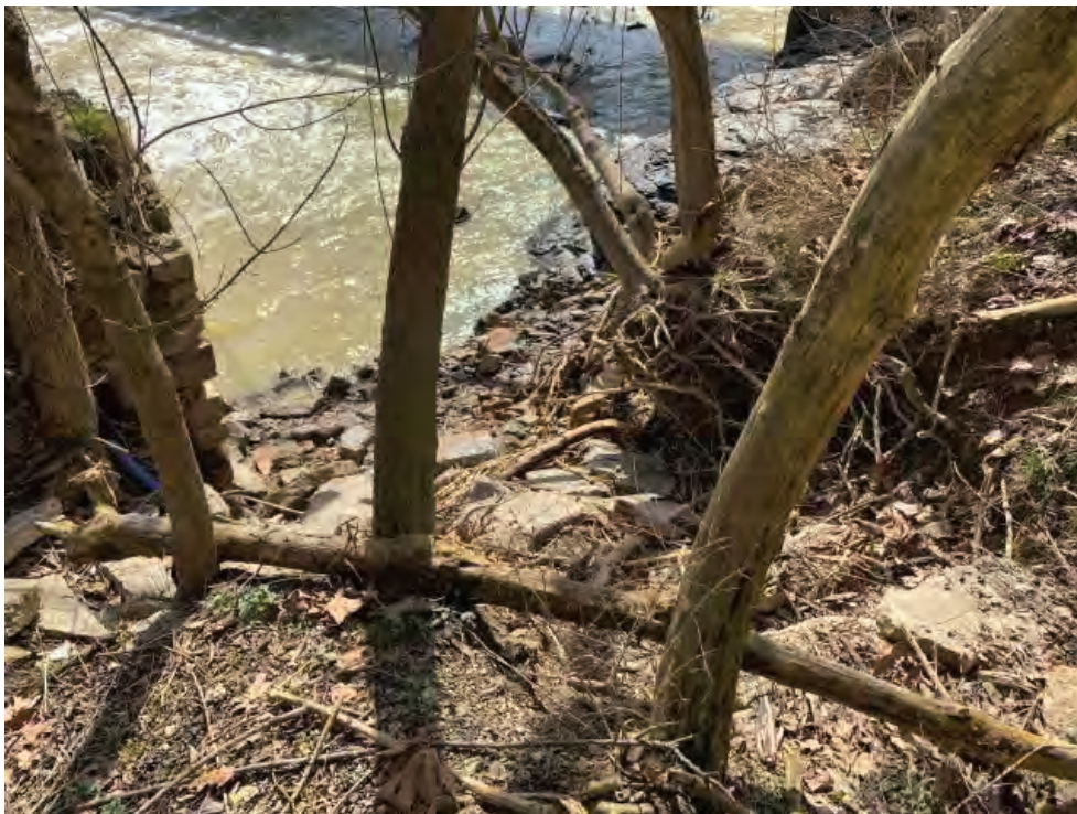
Photo 26. View of the mill's foundation facing southwest
