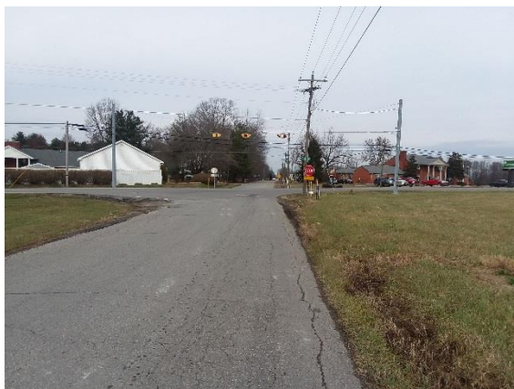
Looking North at Intersection from South
