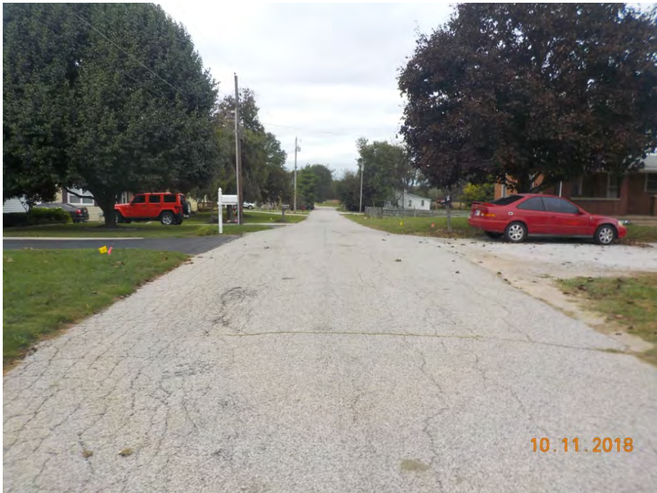
F 93. View of marked utilities along Hacker Drive, looking west.
