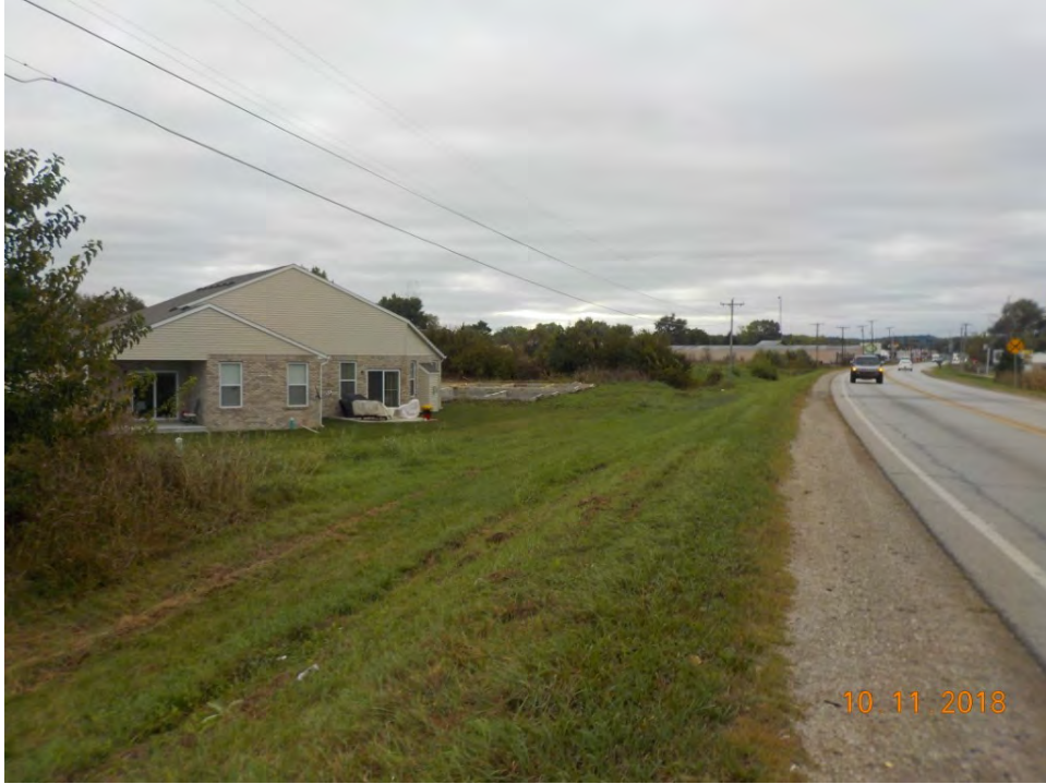
F 76. View of Post 2015 construction on the east side of the project area, looking Southeast along SR 39.
