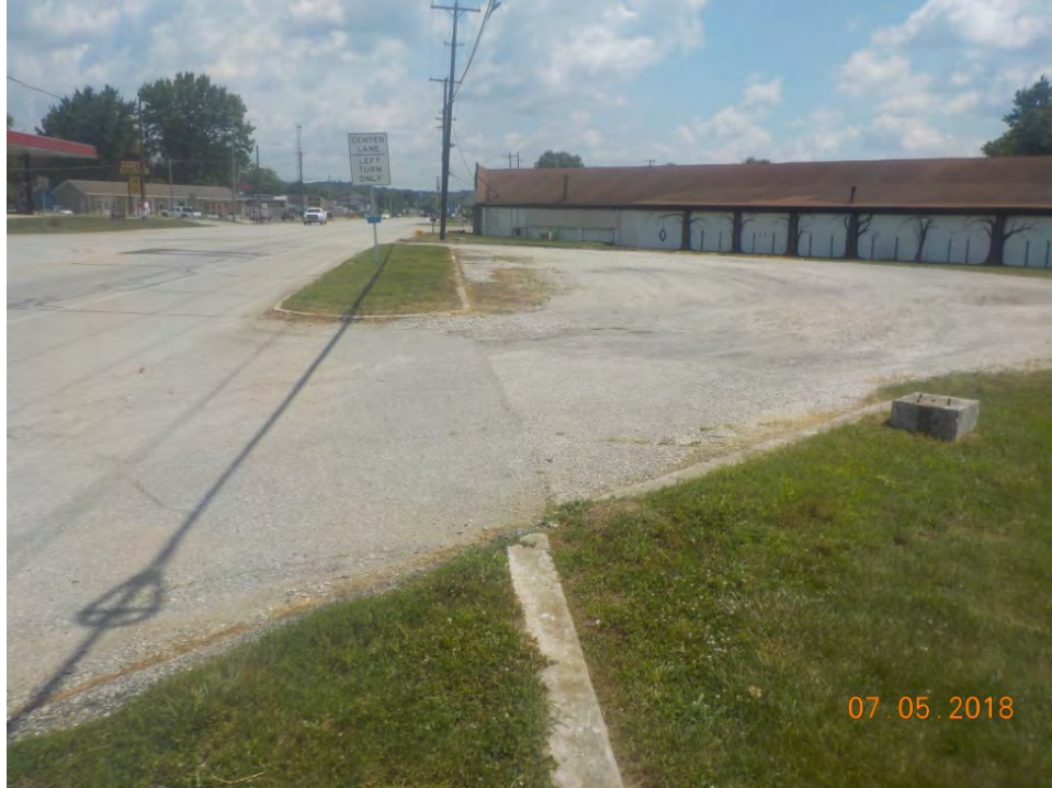
F 36. View of the east side of the project area showing the area disturbed by a parking lot and island, looking northeast along SR 39.
