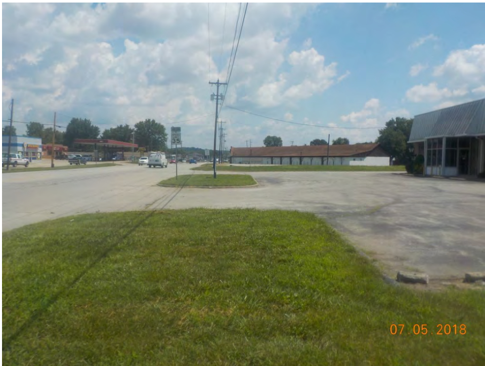
F 35. View of the east side of the project area, north of Burton Lane showing the area disturbed by a parking lot and parking island, looking northeast along SR 39.
