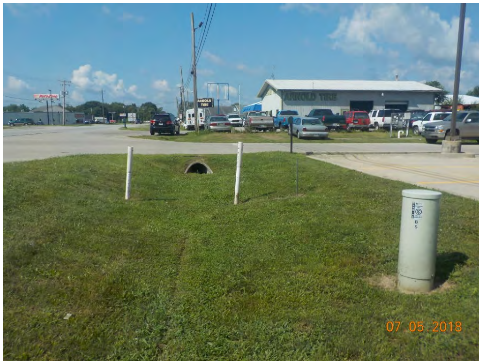
F 27. View of the west side of the project area showing the area disturbed by a culvert, ditch, and underground utilities, looking southwest along SR 39.
