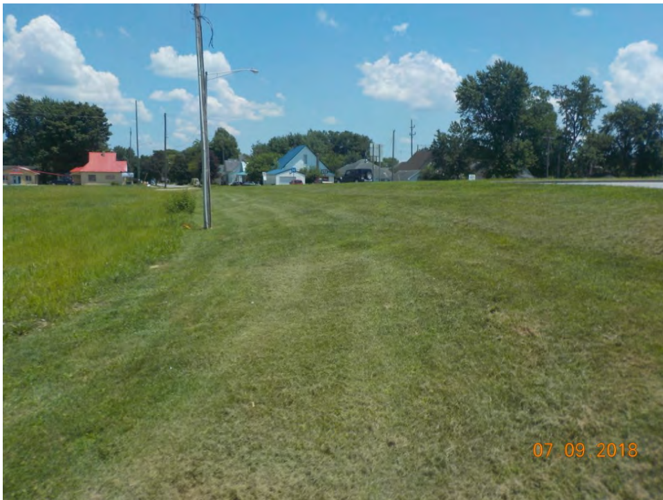
F 85. View of the east side of the project area at Morgan Street showing restored area of recently demolished complex, looking east.
