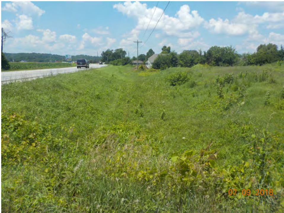
F 77. View of the east side of the project area north of the railroad tracks showing disturbance by a large ditch, looking northwest along SR 39.
