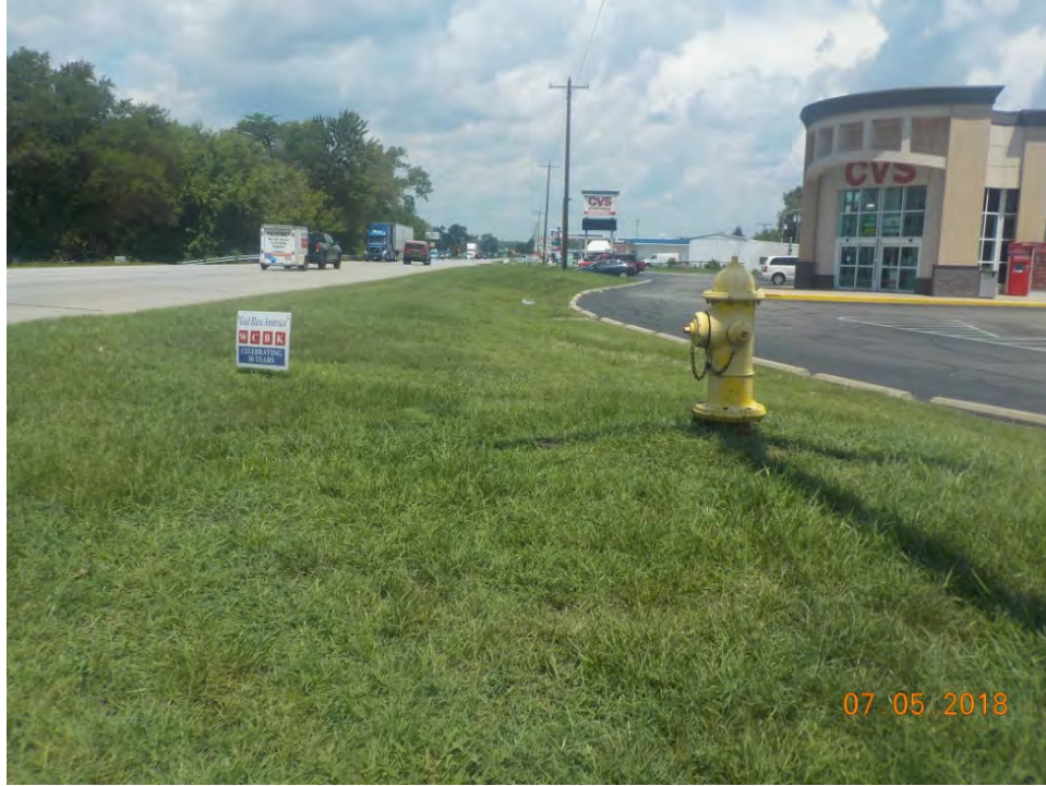
F 60. View of the east side of the project area north of Randolph Street showing the area disturbed by a fire hydrant, storm drain, and parking lot, looking northwest along SR 39.
