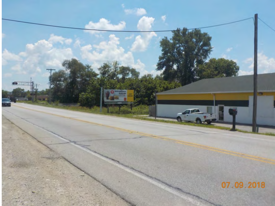
F 66. View of the west side of the project area at the railroad tracks showing the sloping road grade down to a gravel parking area, looking southwest along SR 39.
