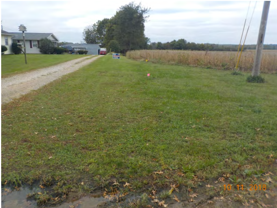
F 95. View of marked utilities at the west end of the project limits on Hacker Drive, looking west.
