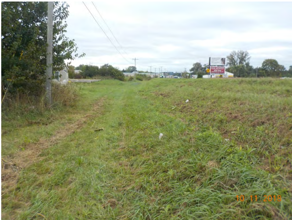
F 75. View of east side of the project area showing the disturbance by the road grade and shallow ditch, looking southeast along SR 39.
