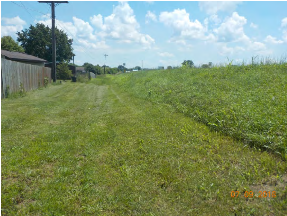
F 73. View of the east side of the project area at Washington Street showing the disturbance by the road grade and shallow ditch, looking southeast along SR 39.
