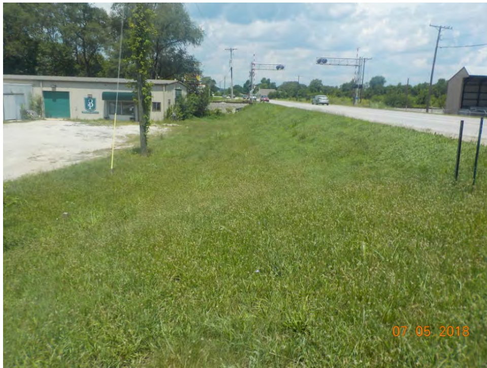
F 57. View of the project area at the north side of Mitchell Avenue showing the sloping road grade, looking northwest along SR 39.
