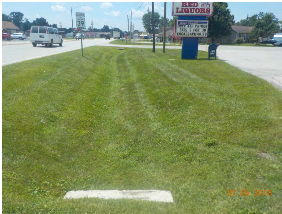
F 41. View of the west side of the project area at the intersection of SR 39 and Morton Avenue showing the area disturbed by a roadside ditch and culverts, looking southwest along SR 39.
