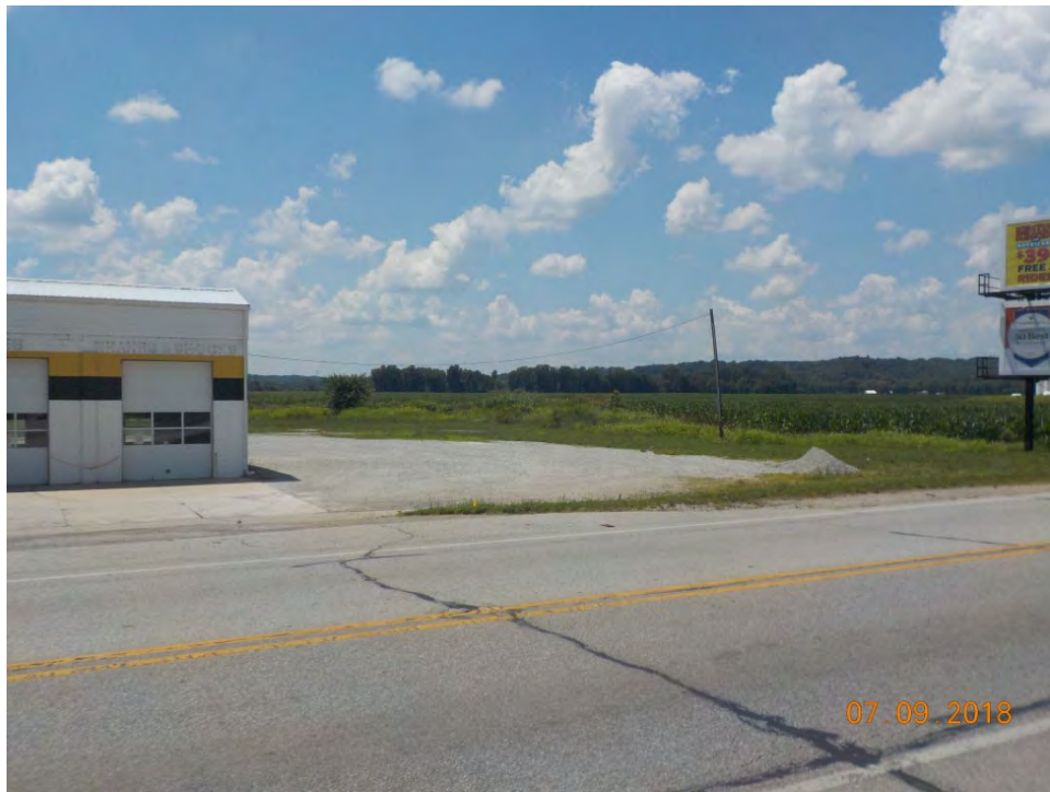
F 67. View of the west side of the project area at the railroad tracks showing the sloping road grade down to a gravel parking area, looking west along SR 39.
