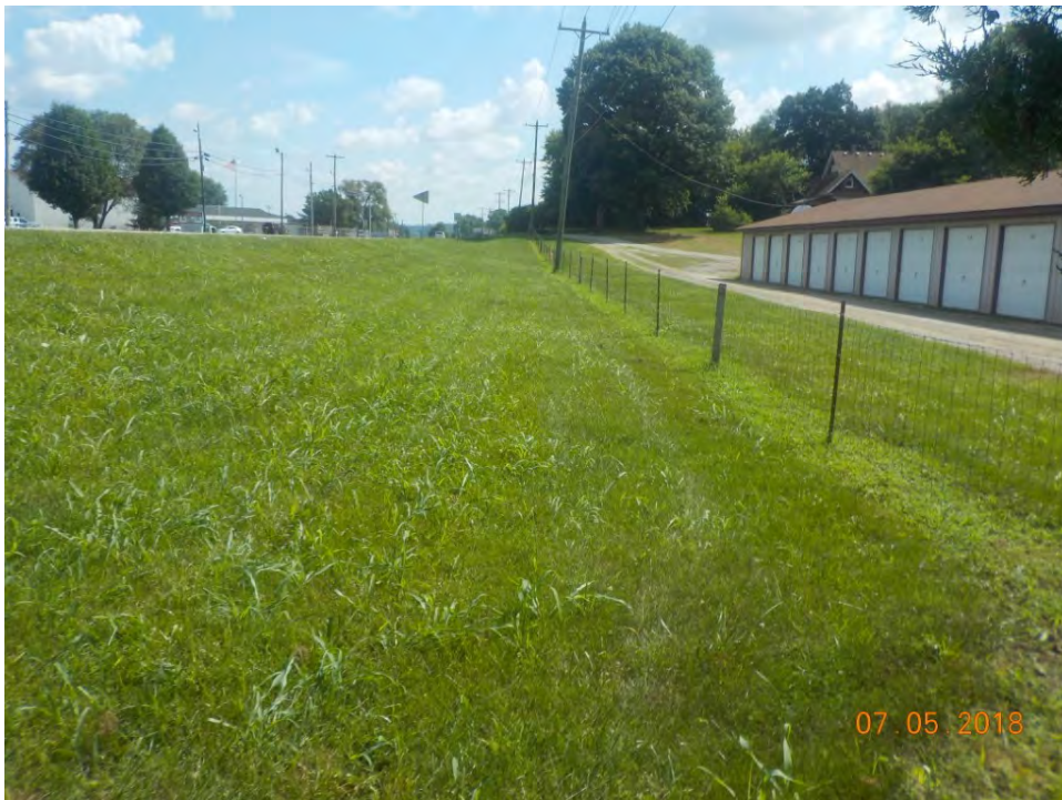
F 23. View of the east side of the project area showing the area disturbed by grading of the road grade, looking northeast along SR 39.
