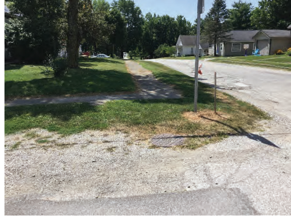
Figure 3: Looking south at the sidewalk and area of the proposed curbs and buffer lawns near the George Seybold House.
