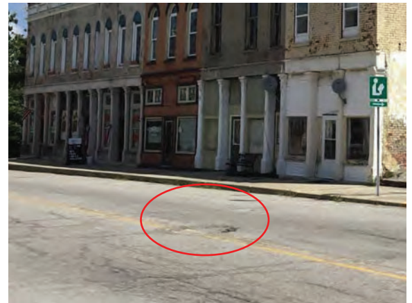
Figure 17: Looking northeast across the Cross Street and alley intersection where surface evidence is visible of a possible cistern below.
