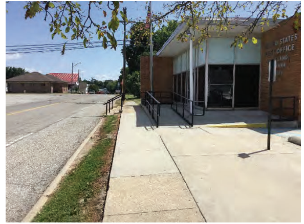
Figure 9: Looking east at the sidewalk, ramp, and steps in front of the Waveland Post Office.
