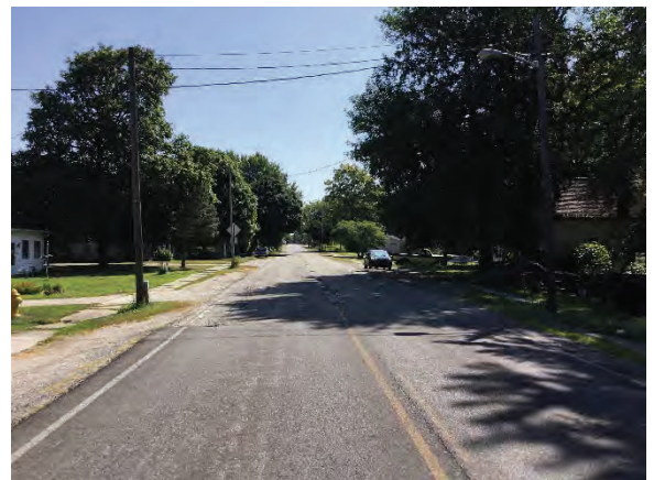
Figure 2: Looking east along SR 59/Main Street in Section 2.
