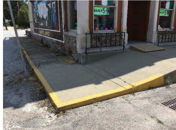
Figure 4: Looking southeast at the non-contributing (post 1985) concrete sidewalk ramp in front of the Union Block.
