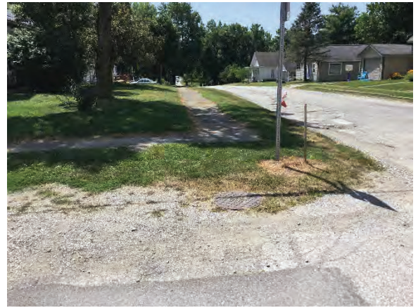
Figure 12: Looking south at the sidewalk and area of the proposed curbs and buffer lawns near the George Seybold House.
