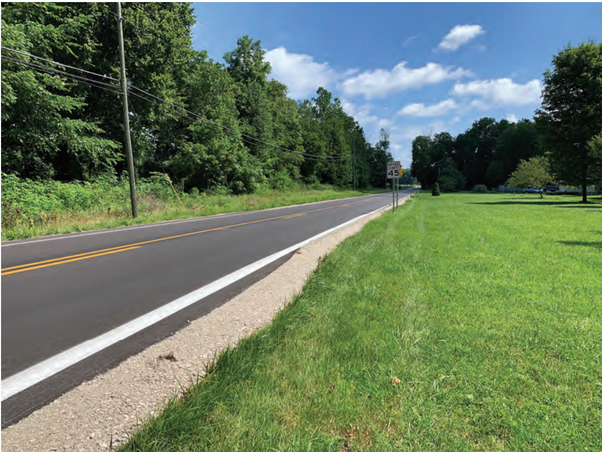
8. View of SR 58 facing northeast
