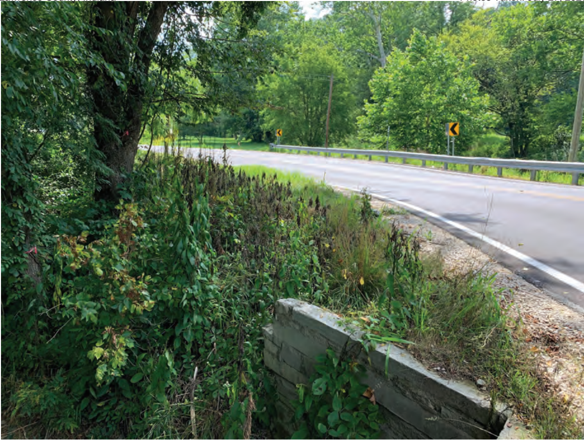
3. View of SR 58, top of culvert facing southeast
