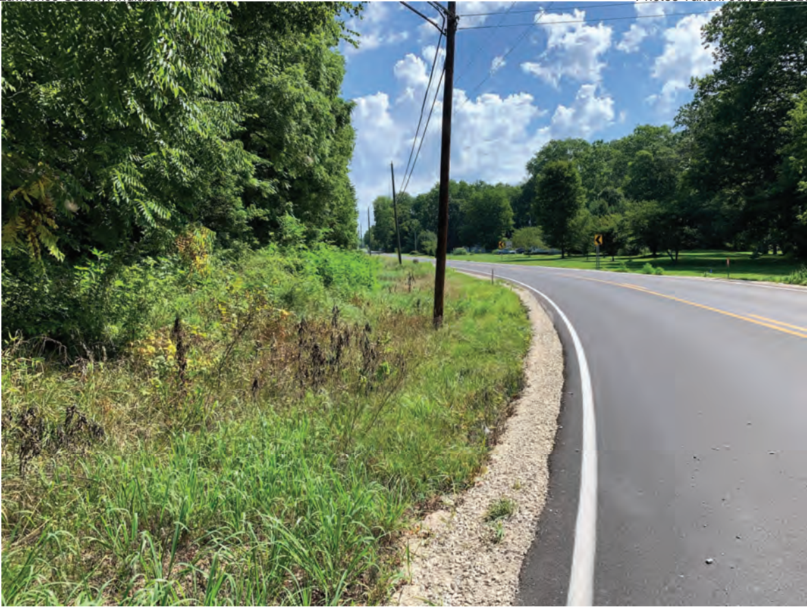
5. View of SR 58 facing northeast
