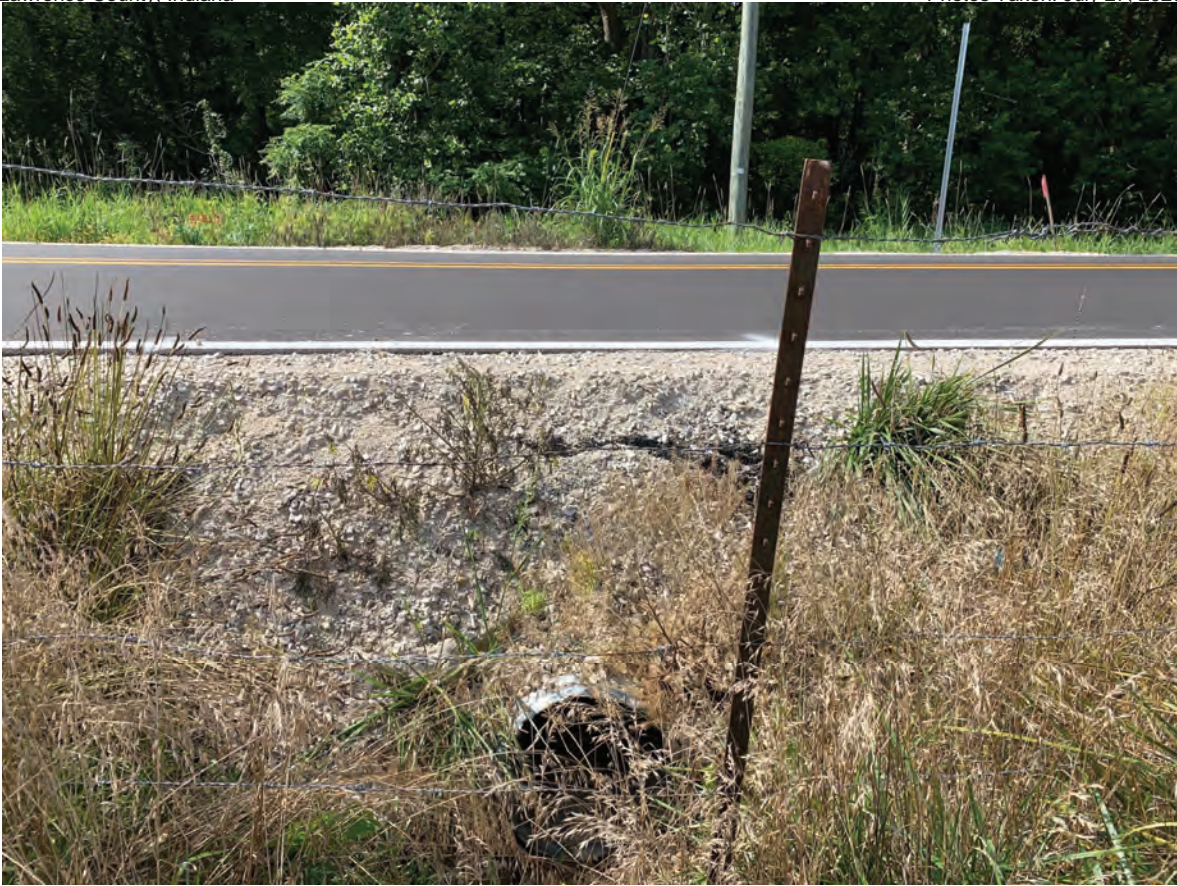
1. View of culvert inlet on north side of SR 58 facing south
