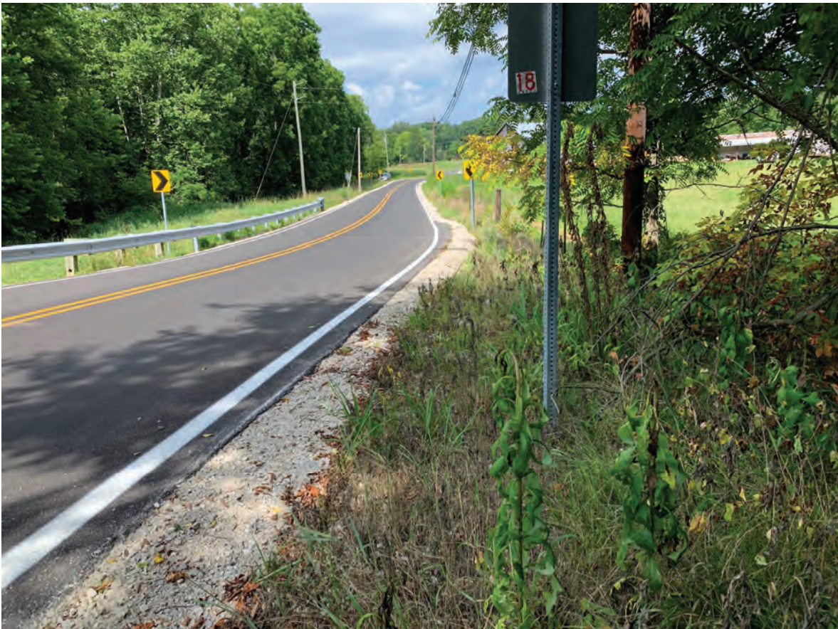
2. View of SR 58, from top of culvert facing west
