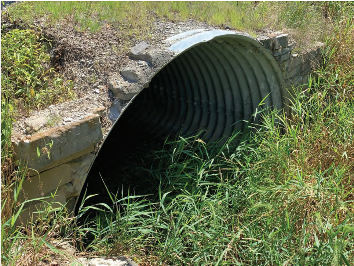
10. View of culvert outlet under SR 58 facing east
