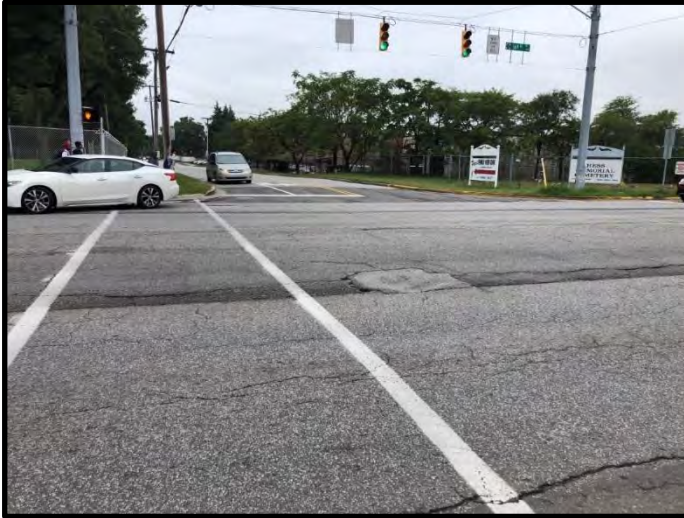
1. View south towards Parrish Avenue and 169 th Street intersection. 10/2/2019
