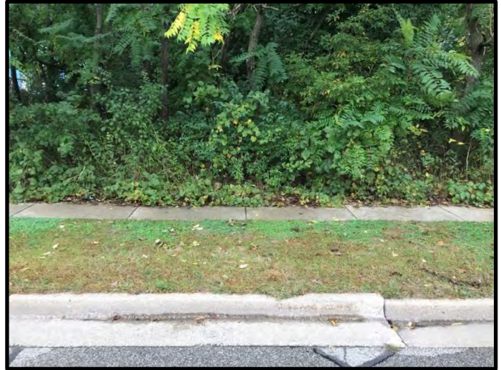
3. View east from Parrish Avenue. 10/2/2019
