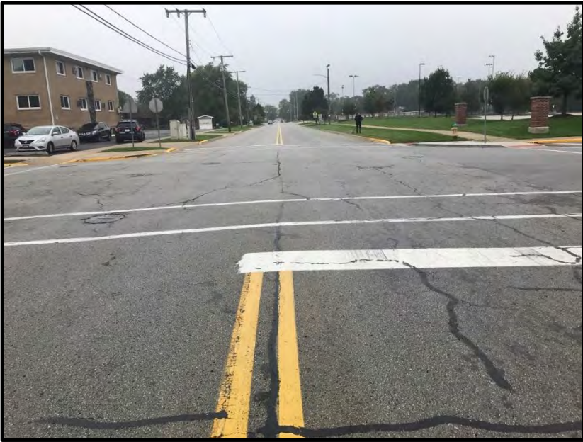
66. View west towards 173 rd Street and Parrish Avenue intersection. 10/2/2019
