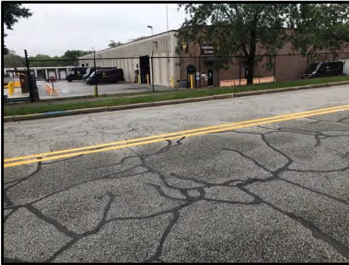
5. View west from Parrish Avenue. 10/2/2019
