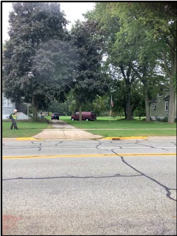
62. View north from 173 rd Street. 10/2/2019
