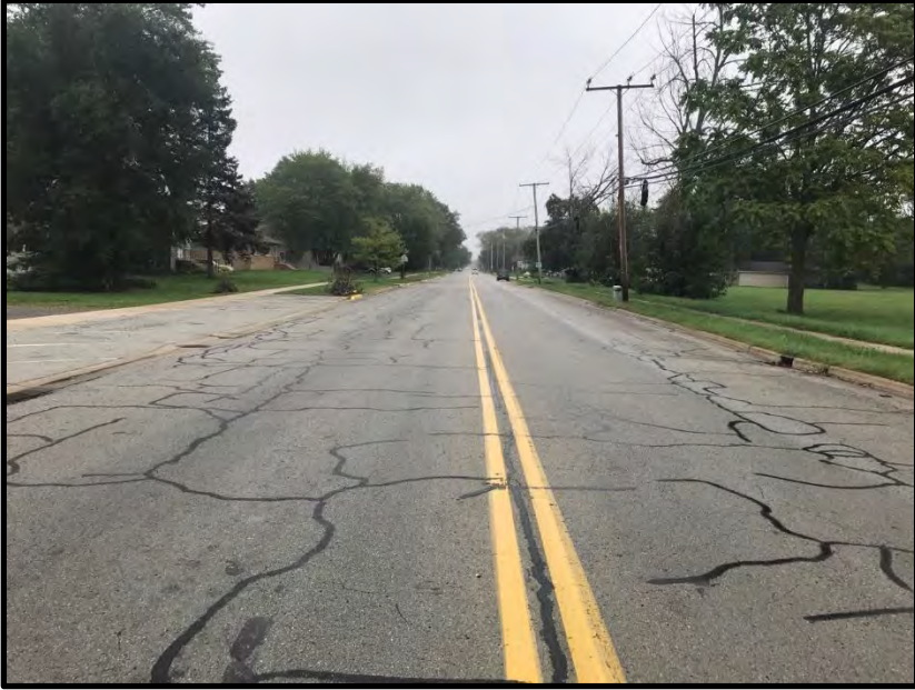
65. View east along 173 rd Street. 10/2/2019
