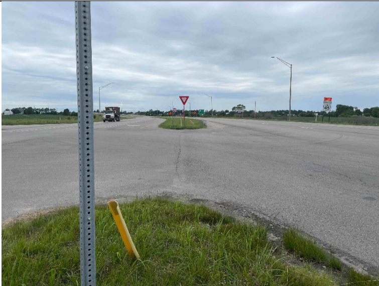
5. Facing northwest in the US 35 median at the US 35/Riggin Road intersection.
