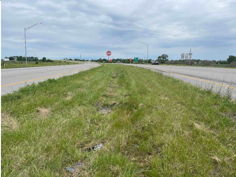
15. Facing north in the median on the north side of the US 35/Riggin Road intersection.
