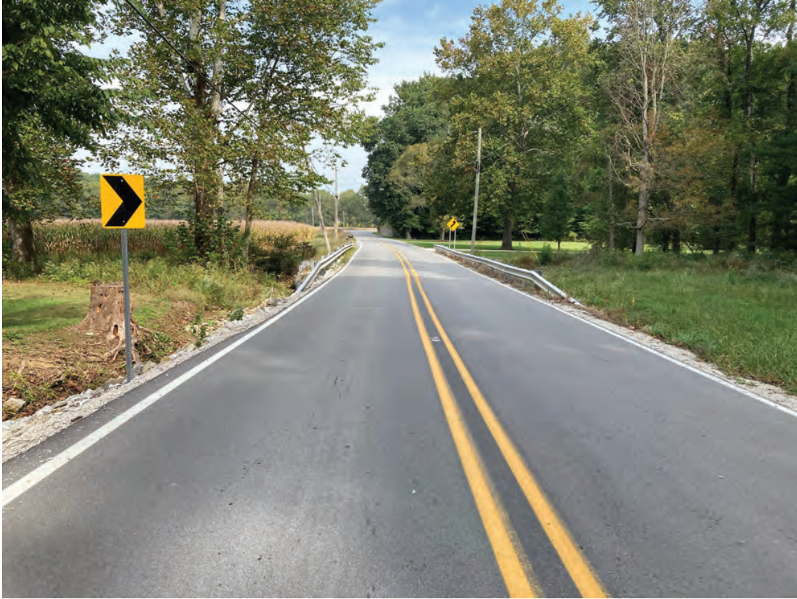
3. Looking north along SR 58 within the northern portion of the project area
