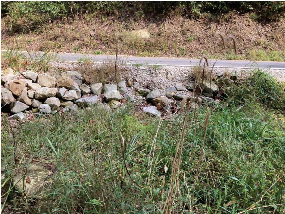
6. Looking northeast at SR 58 westbound shoulder
