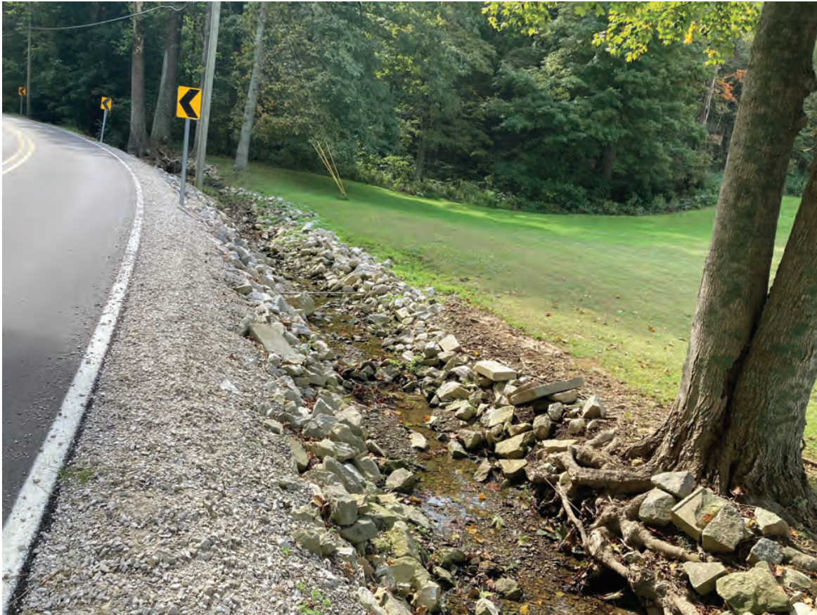
5. Looking south from westbound shoulder at SR 58 embankment and stream
