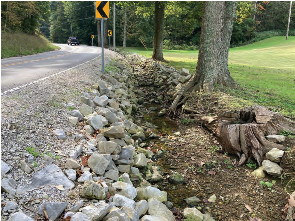
4. Looking south along westbound SR 58 embankment and stream
