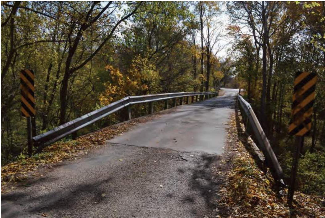
Photo 12. Martin County Bridge No. 58, facing southeast
