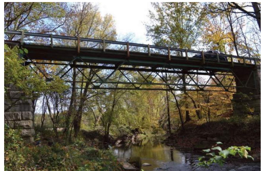
4. View looking east/upstream along Boggs Creek toward bridge crossing
