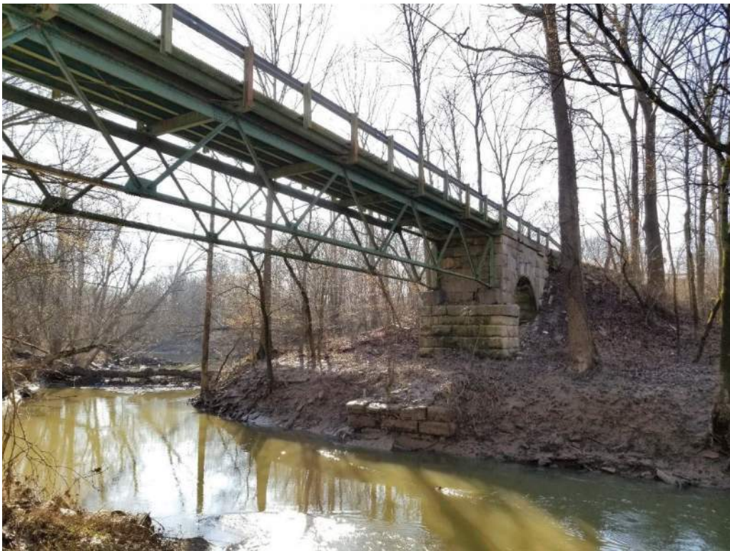
Photo 6: Looking southeast at west truss and south stone arch.
