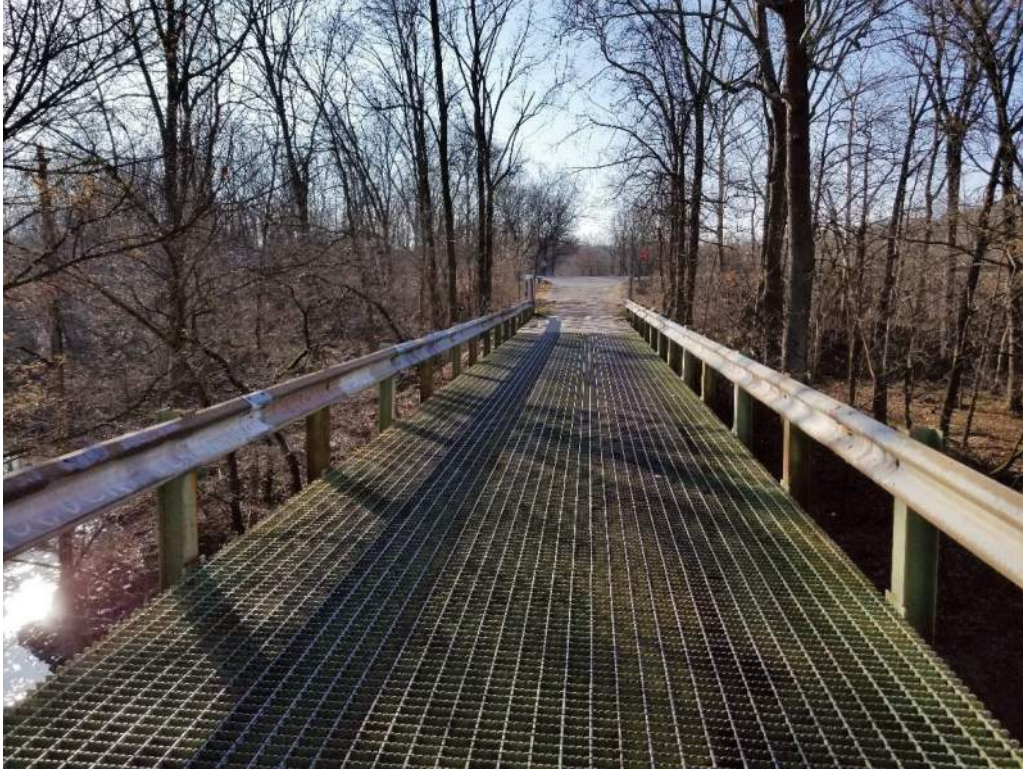
Photo 7: Looking south at steel grid deck.
