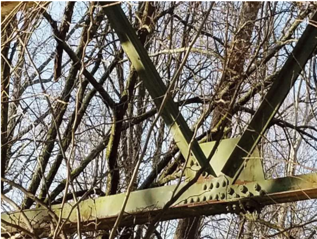
Photo 10: Typical Bottom chord & Diagonal Connection.
