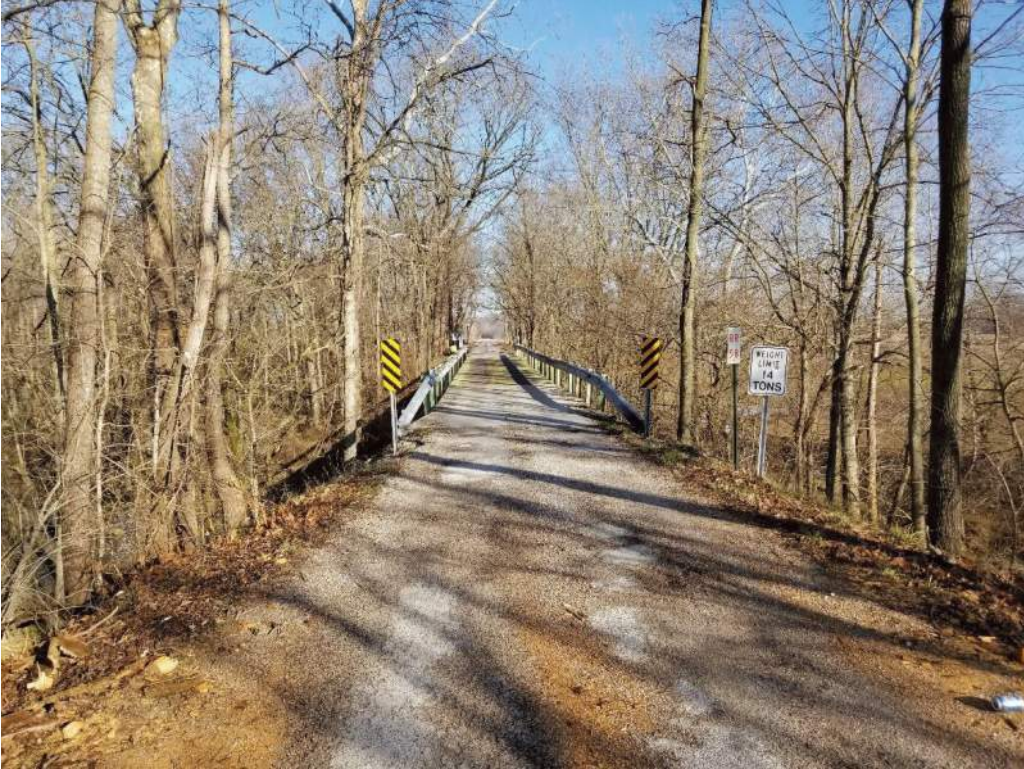
Photo 1: Looking North along Brickyard Road at the approach to Bridge 58.
