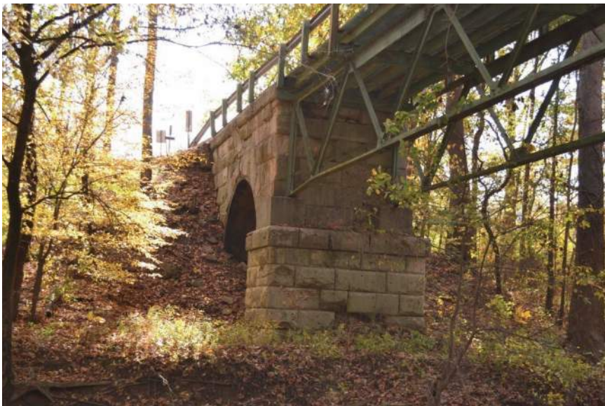
3. View of southern stone abutment
