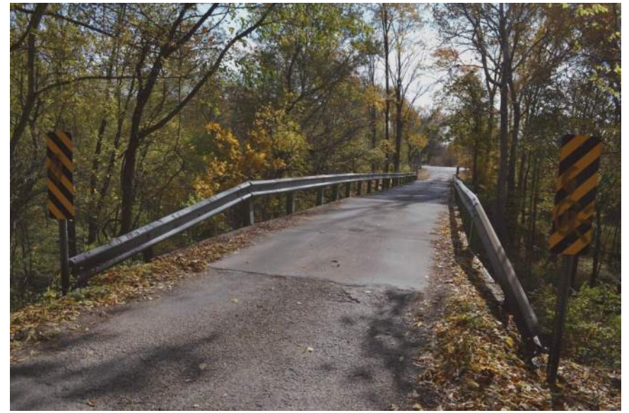
2. View looking south along Brickyard Road toward Project Site
