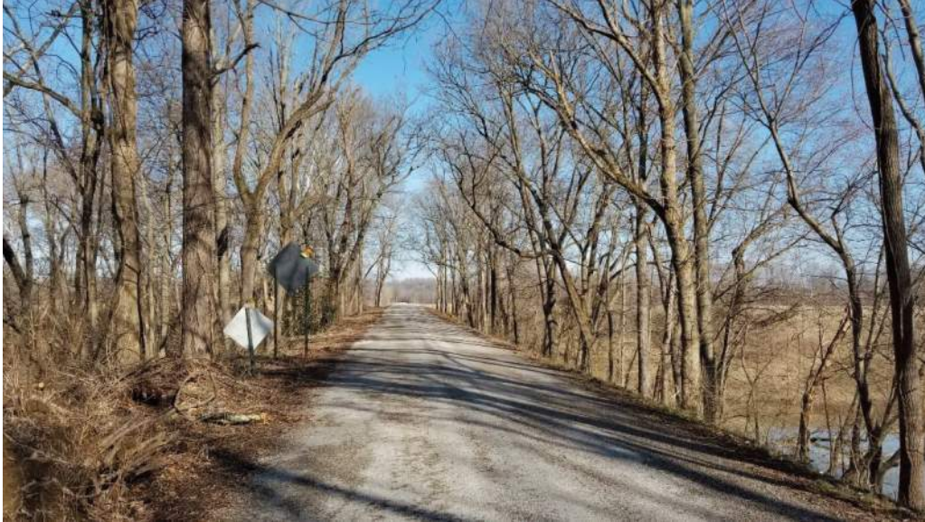
Photo 13: North Approach (Looking North).
