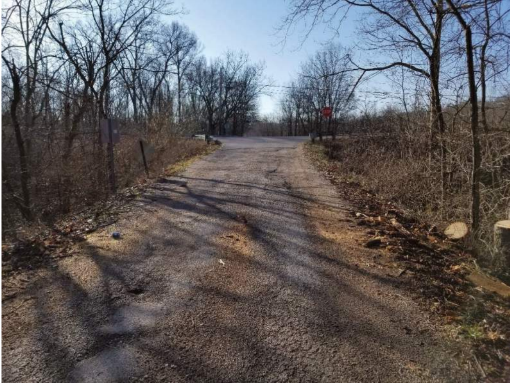
Photo 3: Looking South at US 50 intersection from Bridge 58 south approach.
