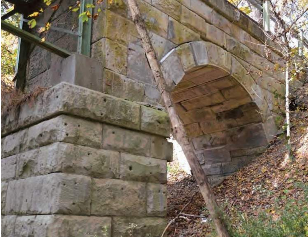
Photo 17. Martin County Bridge No. 58, detail of southern footer, facing east
