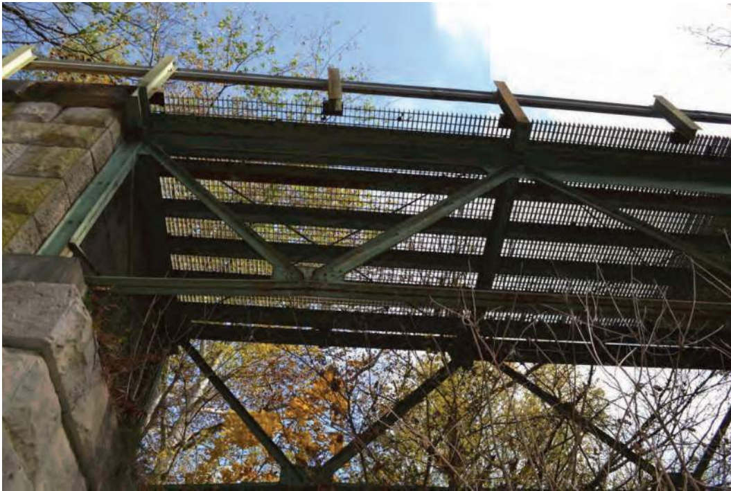
Photo 15. Martin County Bridge No. 58, facing north and up
