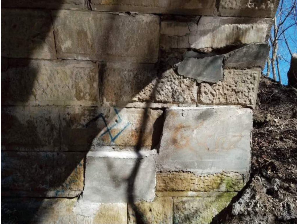
Photo 9: Typical Stone Condition of inside of arches (note: concrete patching).
