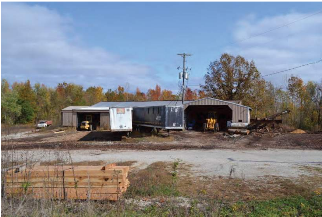
Photo 10. Metal corrugated storage buildings at 2439 Isaacs Road, facing east-northeast
