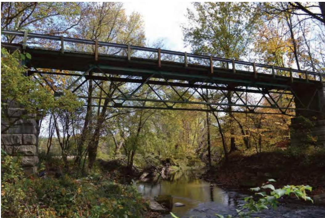
Photo 14. Martin County Bridge No. 58, facing northeast
