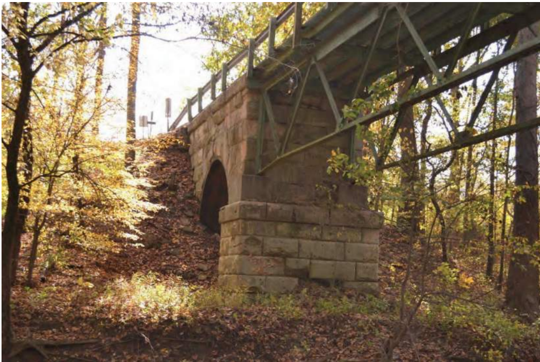
Photo 16. Martin County Bridge No. 58, northern footer, facing north
