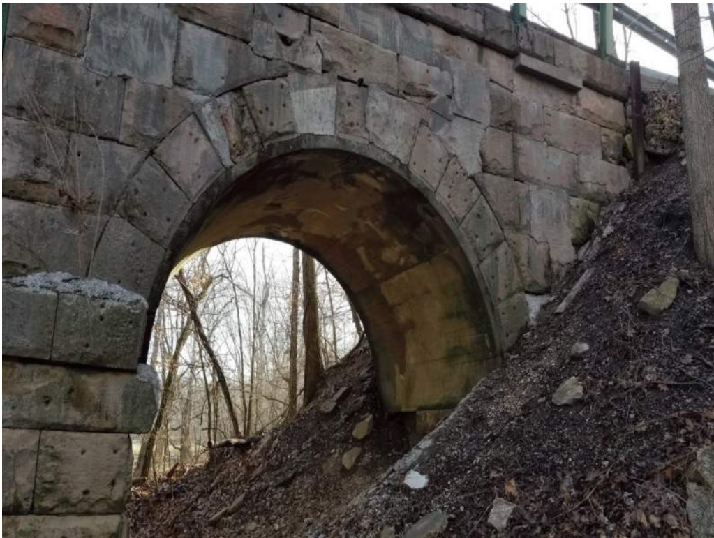
Photo 8: West side of South Stone Arch (typical stone condition).
