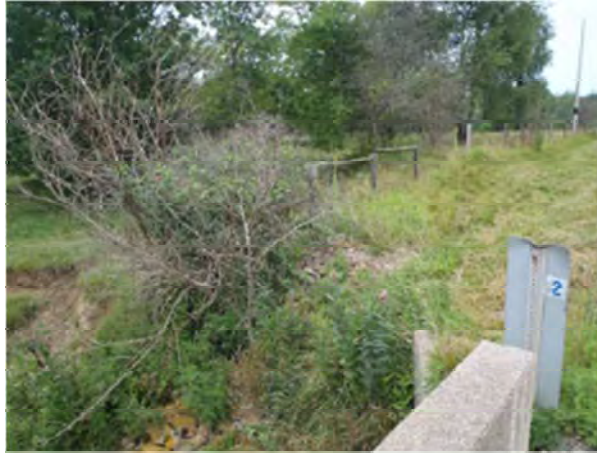
7. Looking southwest from the structure at adjacent vegetation
