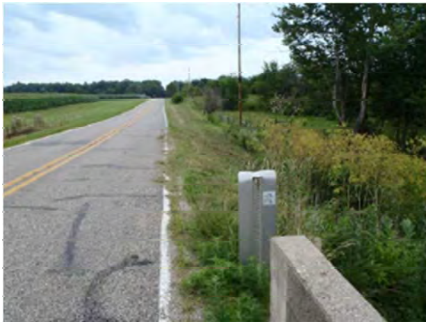
8. Looking east at roadside vegetation along SR 234 from the structure
