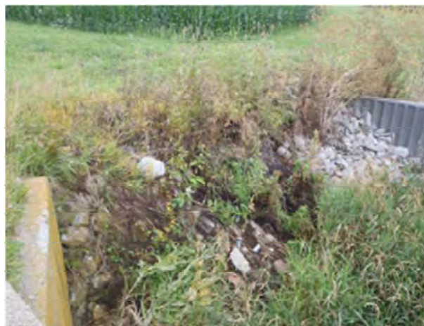
2. Looking northwest from the structure at vegetation
