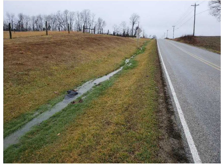
Photo 11. Southwest right-of-way, facing west.
