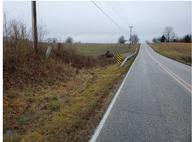
Photo 8. Right-of-way northwest of project, facing east.
