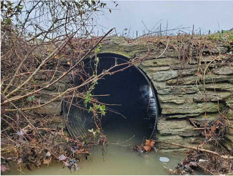
Photo 5. Project culvert outlet, facing north.
