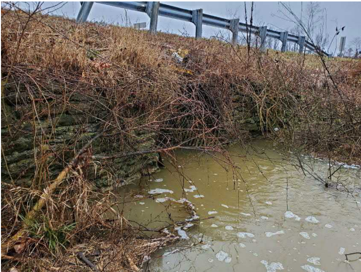
Photo 6. Project culvert inlet, facing southwest.
