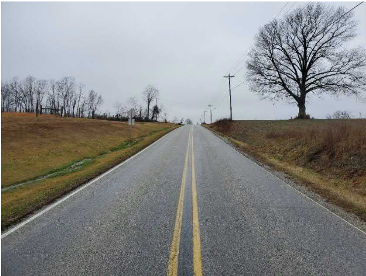
Photo 10. West project approach, facing west.
