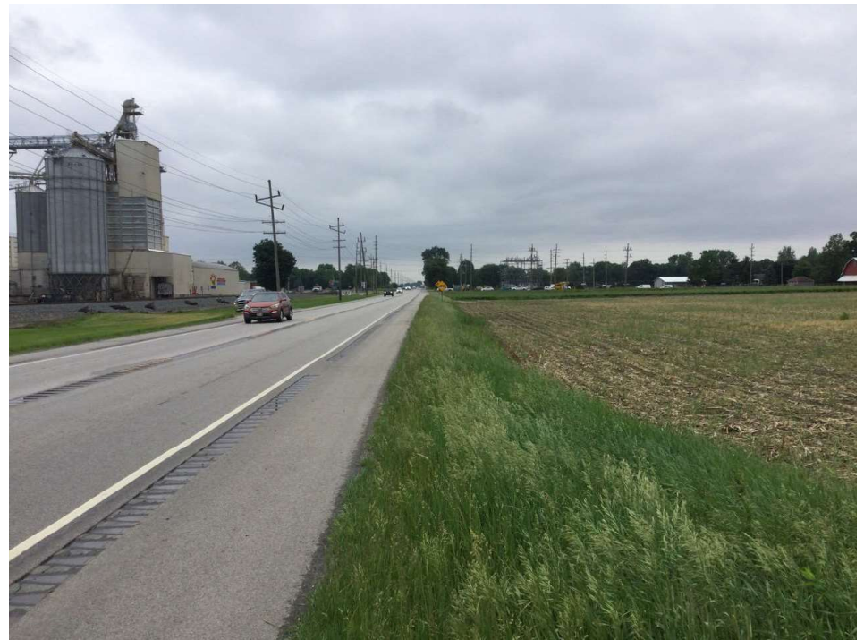
30. Looking south along the west side of SR 15
