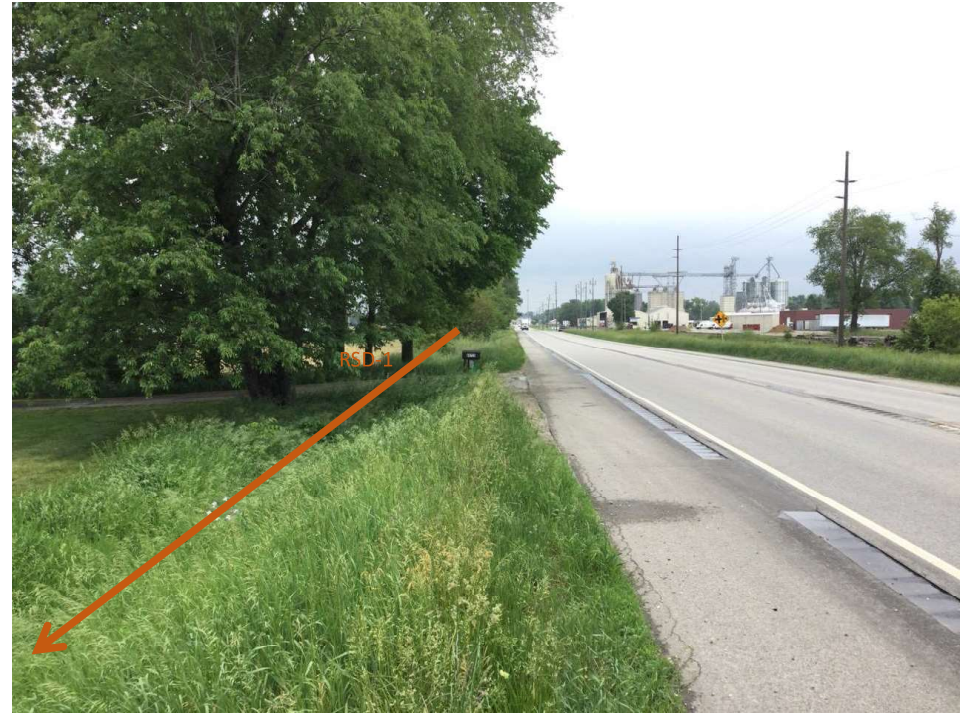
6. Looking north along the west side of SR 15, note RSD 1
