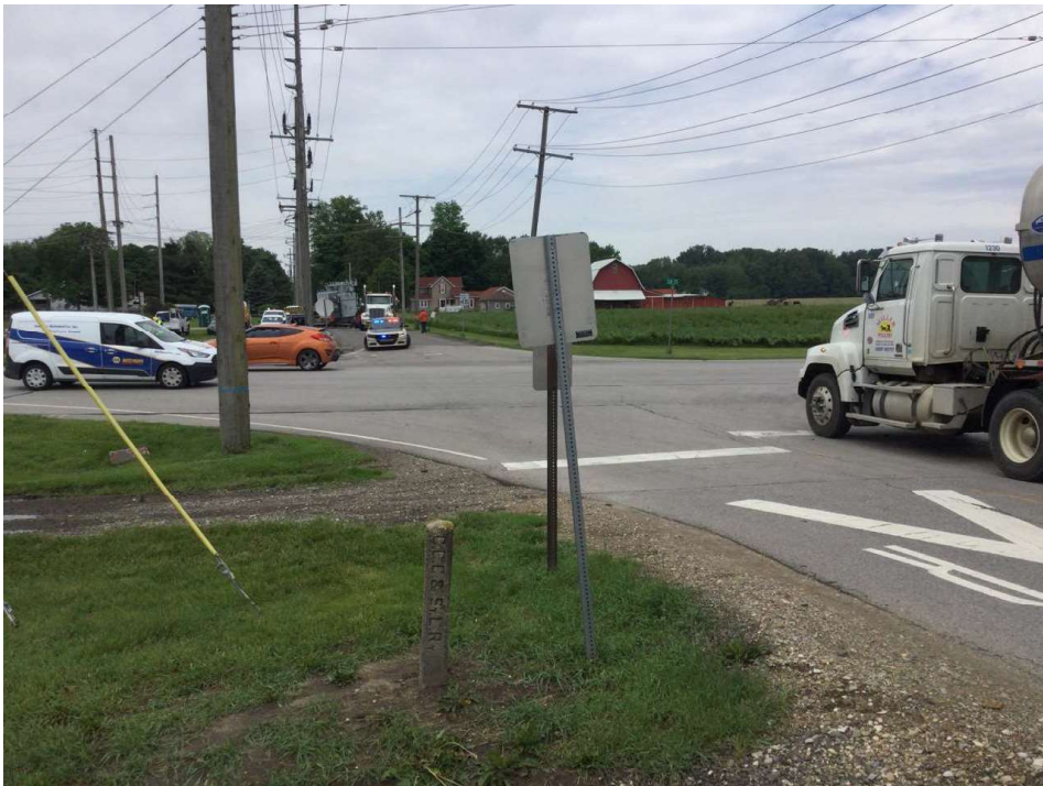
23. Looking west within the southeast quadrant of SR 15 / CR 146 intersection
