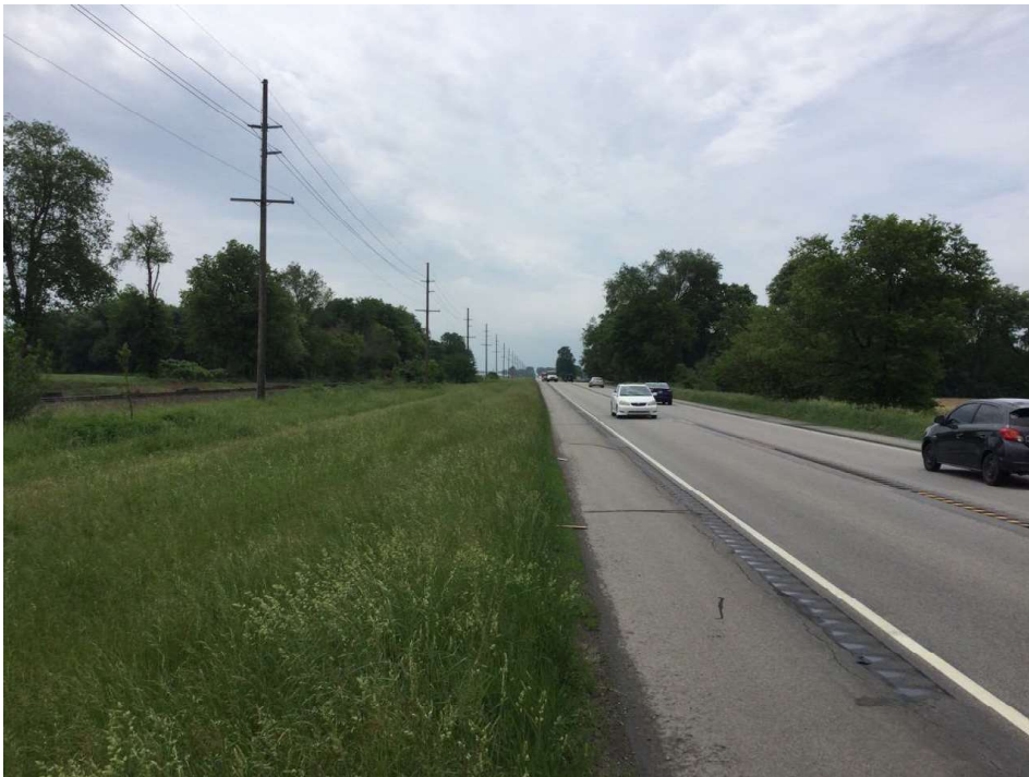
3. Looking south along the east side of SR 15
