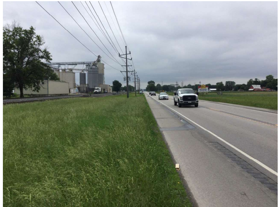
28. Looking south along the east side of SR 15
