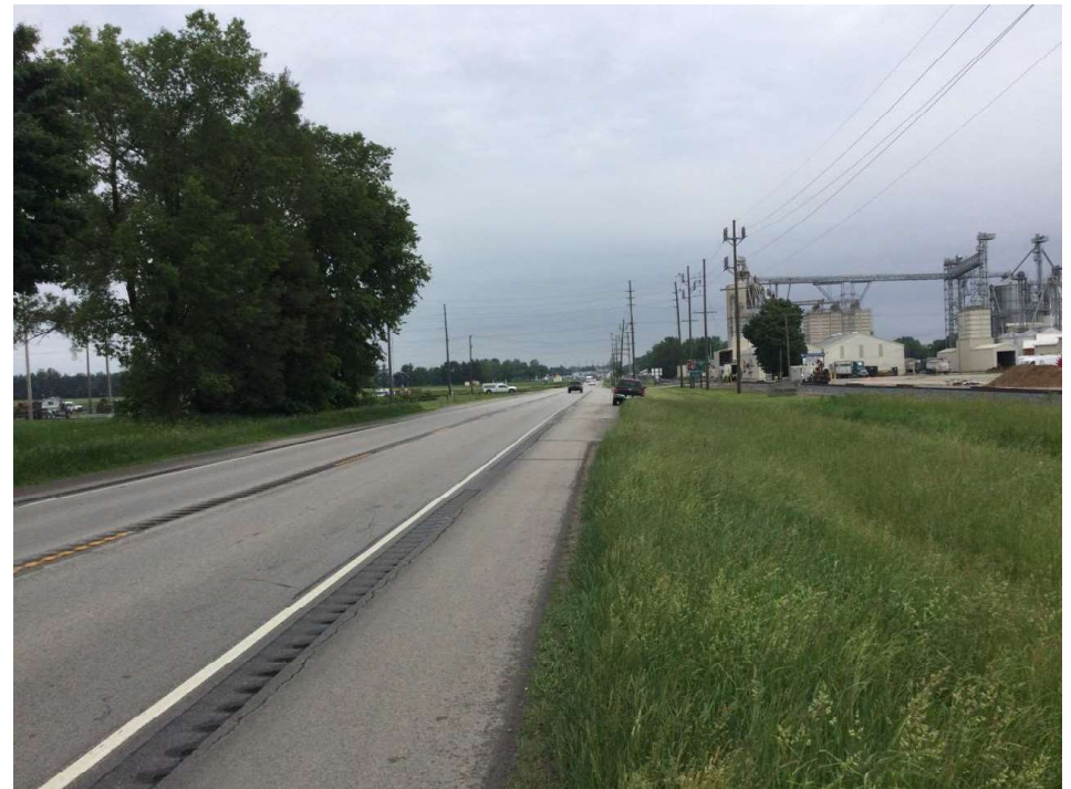
4. Looking north along the east side of SR 15
