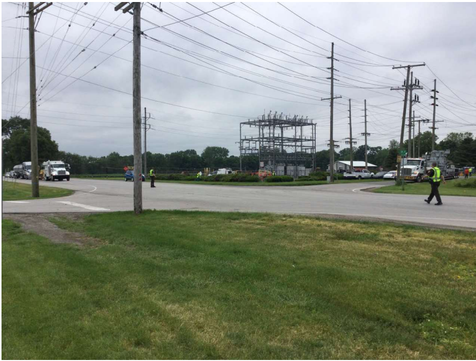
21. Looking southwest within the northeast quadrant of SR 15 / CR 146 intersection
