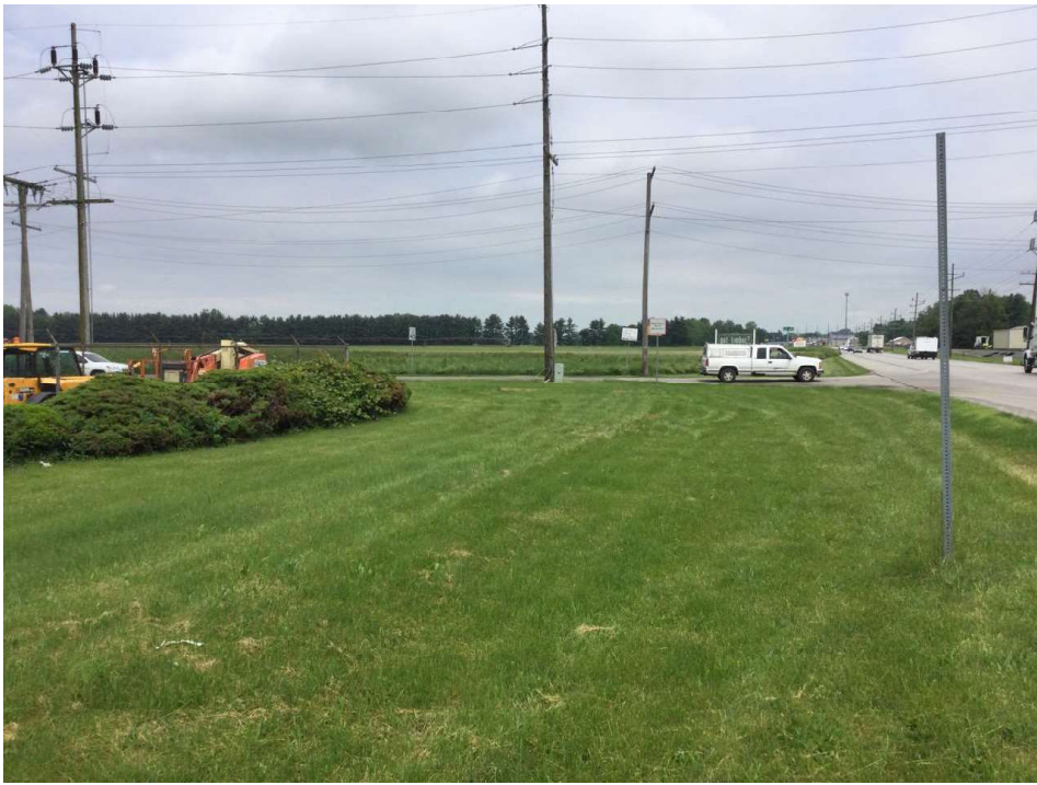
13. Looking north along the west side of SR 15 towards CR 146
