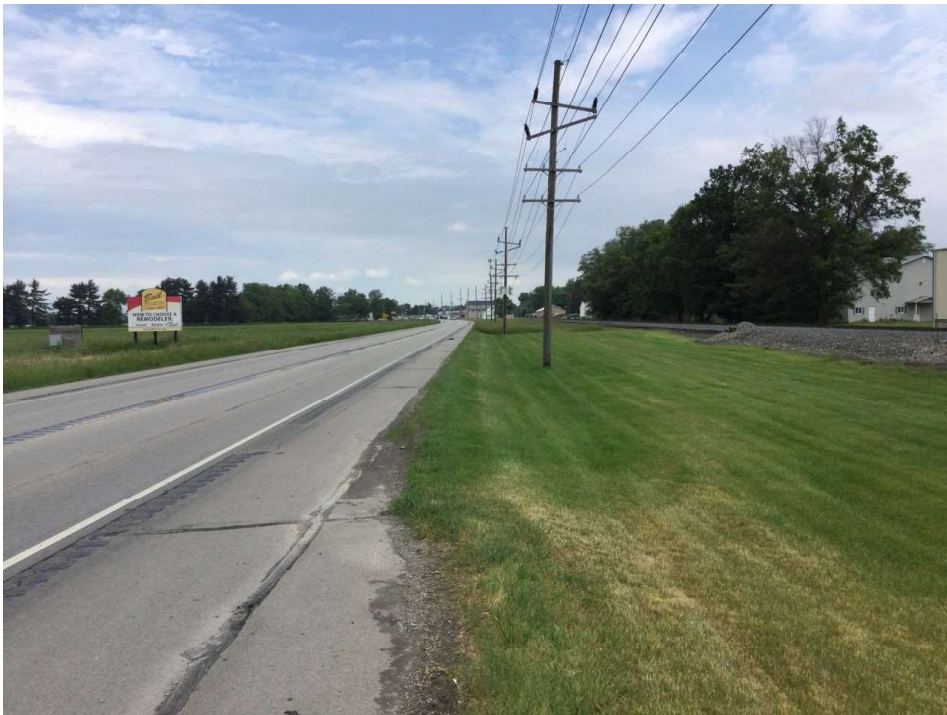
25. Looking north along the east side of SR 15
