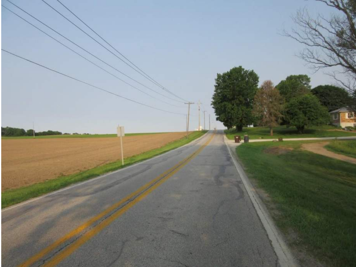
101. Looking along SR 42 facing west within Monrovia. Photo taken 6/3/19.
