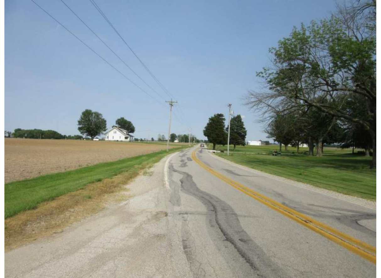
56. Looking east from the intersection of SR 42 and Chas Bray Rd. Photo taken 6/3/19.
