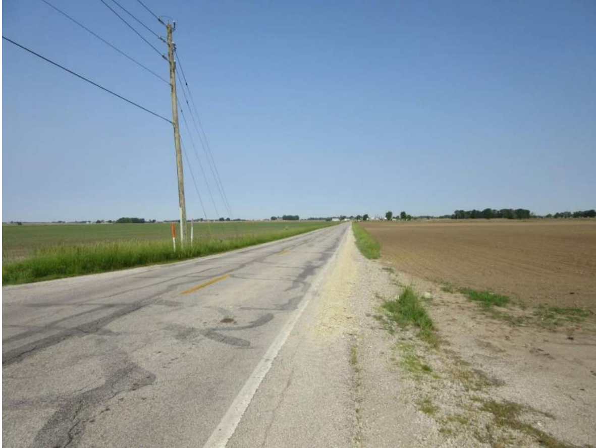
95. Looking west up SR 42 from the intersection of SR 42 and N. Allen Rd. Photo taken 6/3/19.
