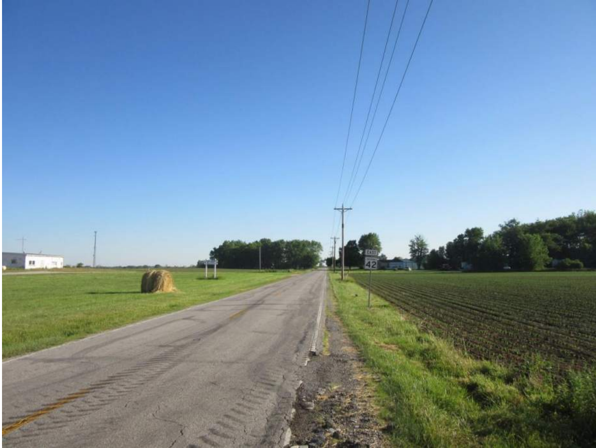
47. From east side of SR 42 looking north up roadway. Photo taken 6/11/19.
