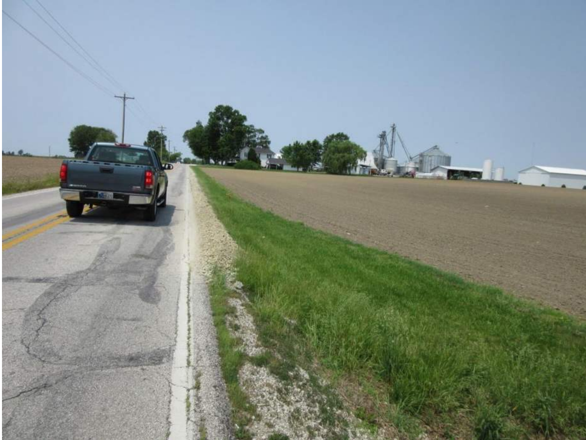
83. Looking west down SR 42 from Structure No. 42 (not pictured). Structure No. 42 conveys UNT 3 to Lake Ditch. Right-of-way is anticipated at this location. Photo taken 6/3/19.
