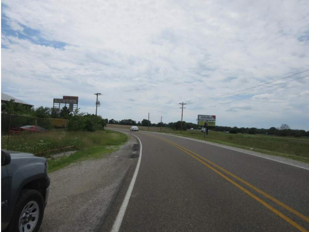
29. From south side of US 42 looking southwest down SR 42. Photo taken 6/12/19.
