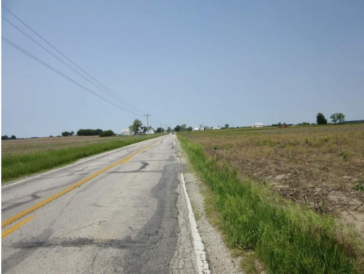
85. Looking west down SR 42 from Lake Ditch road intersection. Photo taken 6/3/19.
