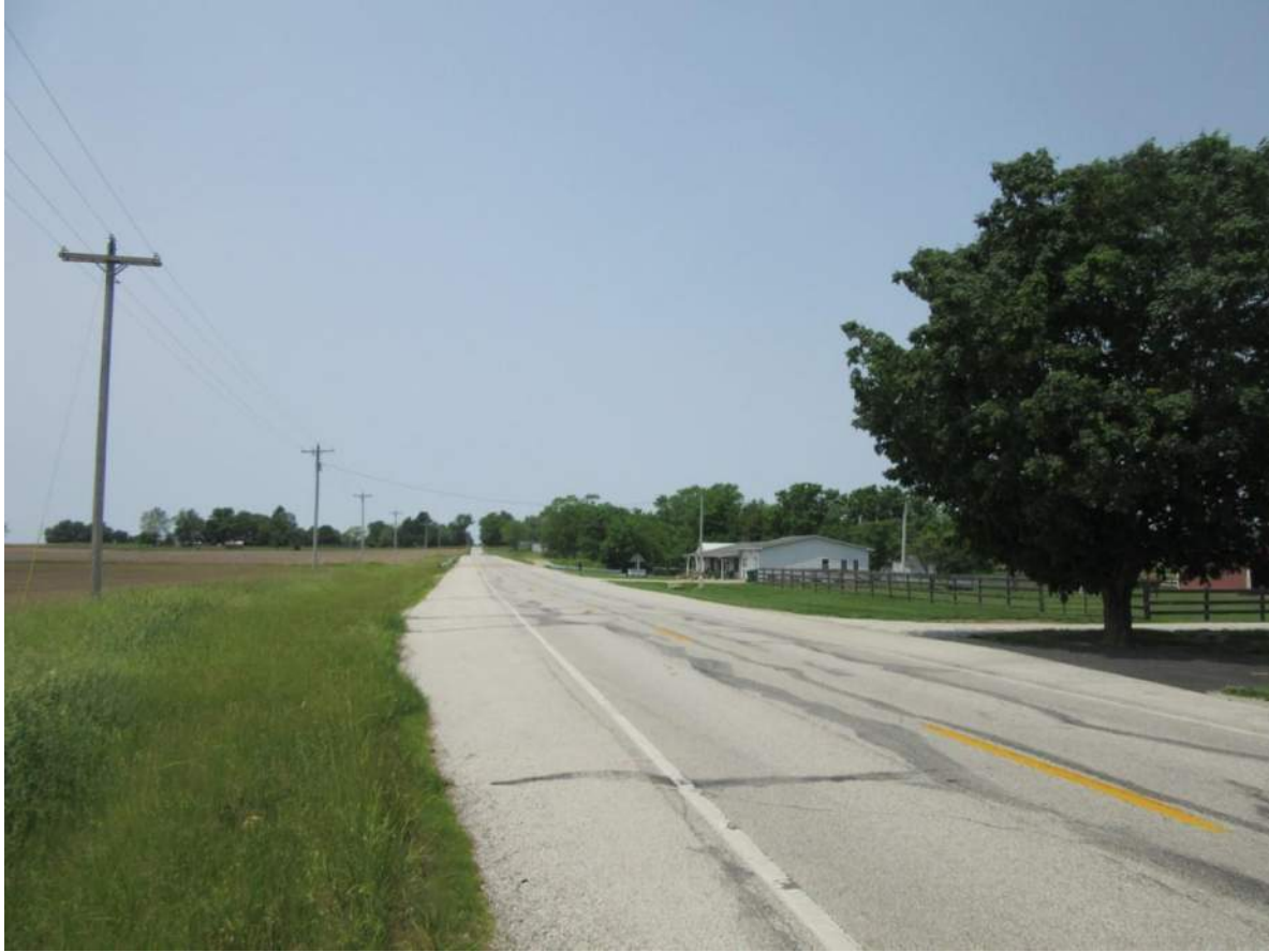
77. Looking west down SR 42. Photo taken 6/3/19.
