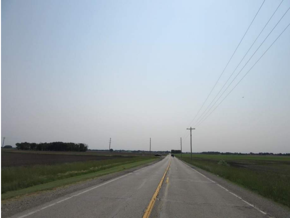
91. Looking east down SR 42. Photo taken 6/3/19.
