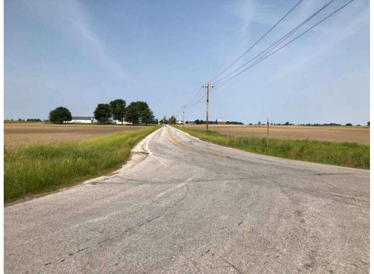
40. Intersection of SR 42, W. Wheeler Rd., and N. Evans Rd. looking west at SR 42. Right-of-way is anticipated at this location. Photo taken 6/4/19.
