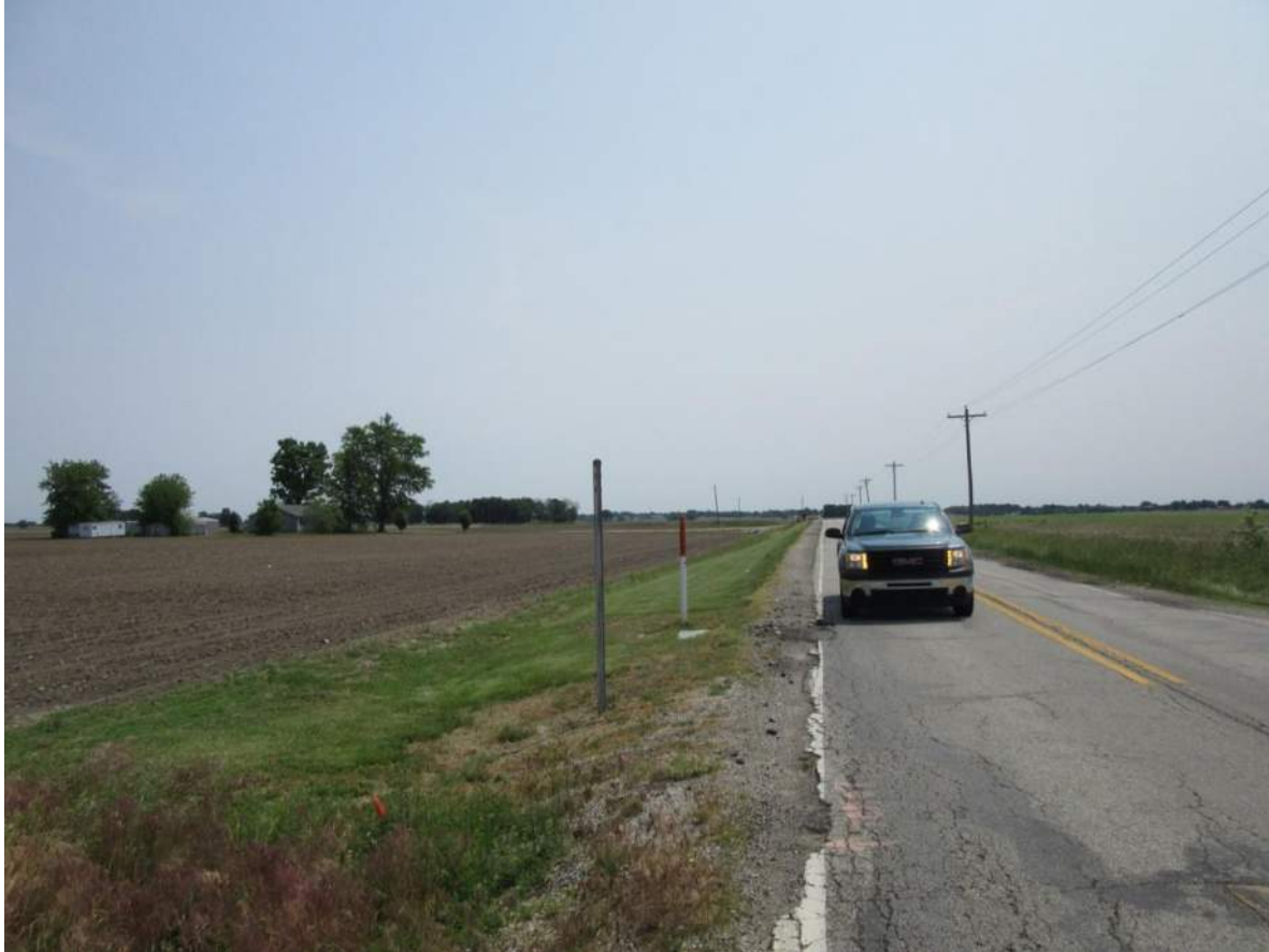
87. Looking east up SR 42 from Lake Ditch Road Intersection. Right-of-way is anticipated at this location. Structure No. 43A (not pictured) but can be partially seen in bottom left of photo. Photo taken 6/3/19.
