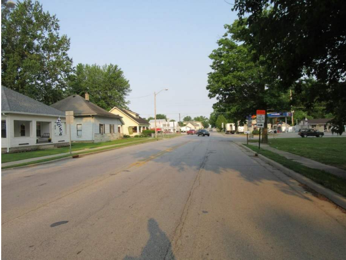
113. From the north side of E Main St/SR 42 looking west within Monrovia. Photo taken 6/3/19.
