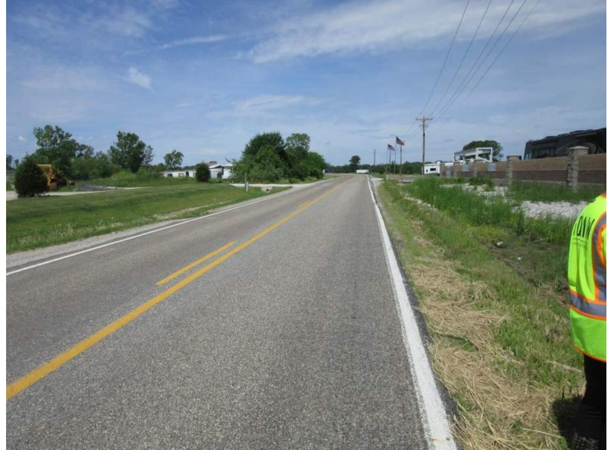
30. From north side of SR 42 looking west down SR 42. Wetland W can be seen to the right of the photo. Photo taken 6/12/19.
