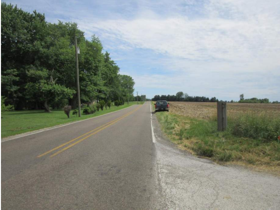
11. From SR 42 looking south at roadway from McClure Road intersection. Photo taken 6/12/19.
