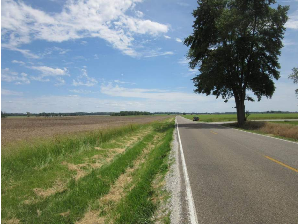
23. Looking south down SR 42 and ditch line from east side of SR 42. Photo taken 6/12/19.
