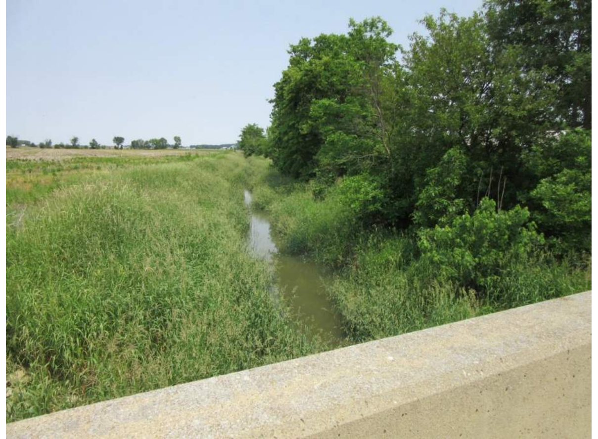
74. Looking northeast from center of structure up UNT 4 to Lake Ditch. This structure is exempted from the project. Photo taken 6/3/19.
