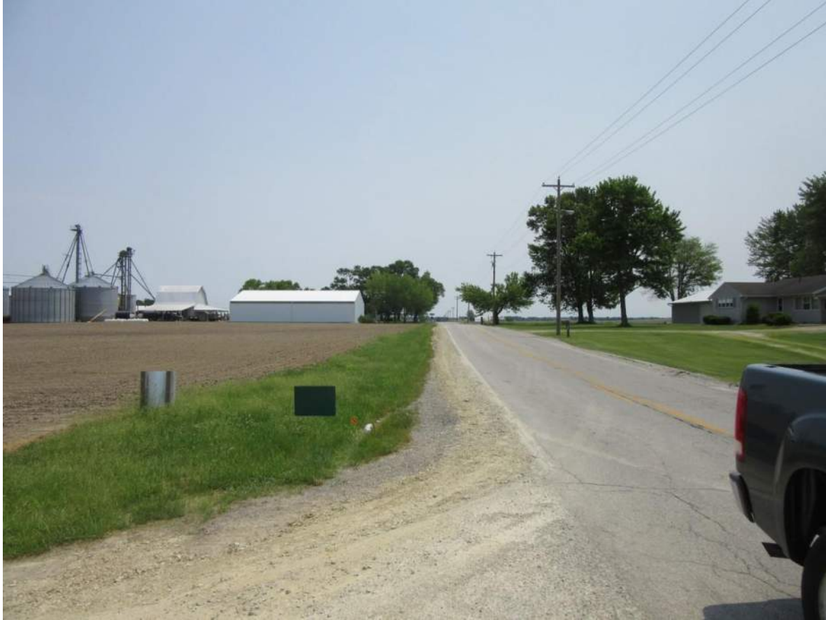
81. Looking east down SR 42 from the intersection of Hall Rd and SR 42. Photo taken 6/3/19.
