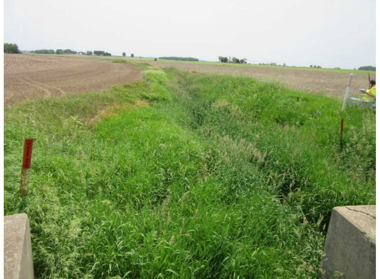
64. Looking southwest down UNT 5 to Lake Ditch from Structure Nos. 40 & 40A. Right-of-way is proposed at this location. Photo taken 6/3/19.
