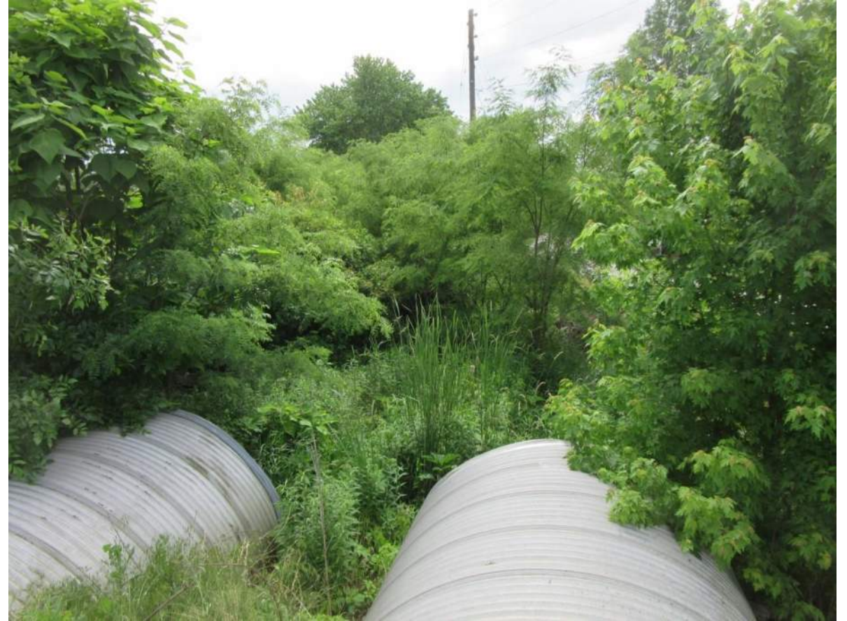
8. Looking west at UNT 11 to Lake Ditch from SR 42. Photo taken 6/12/19.
