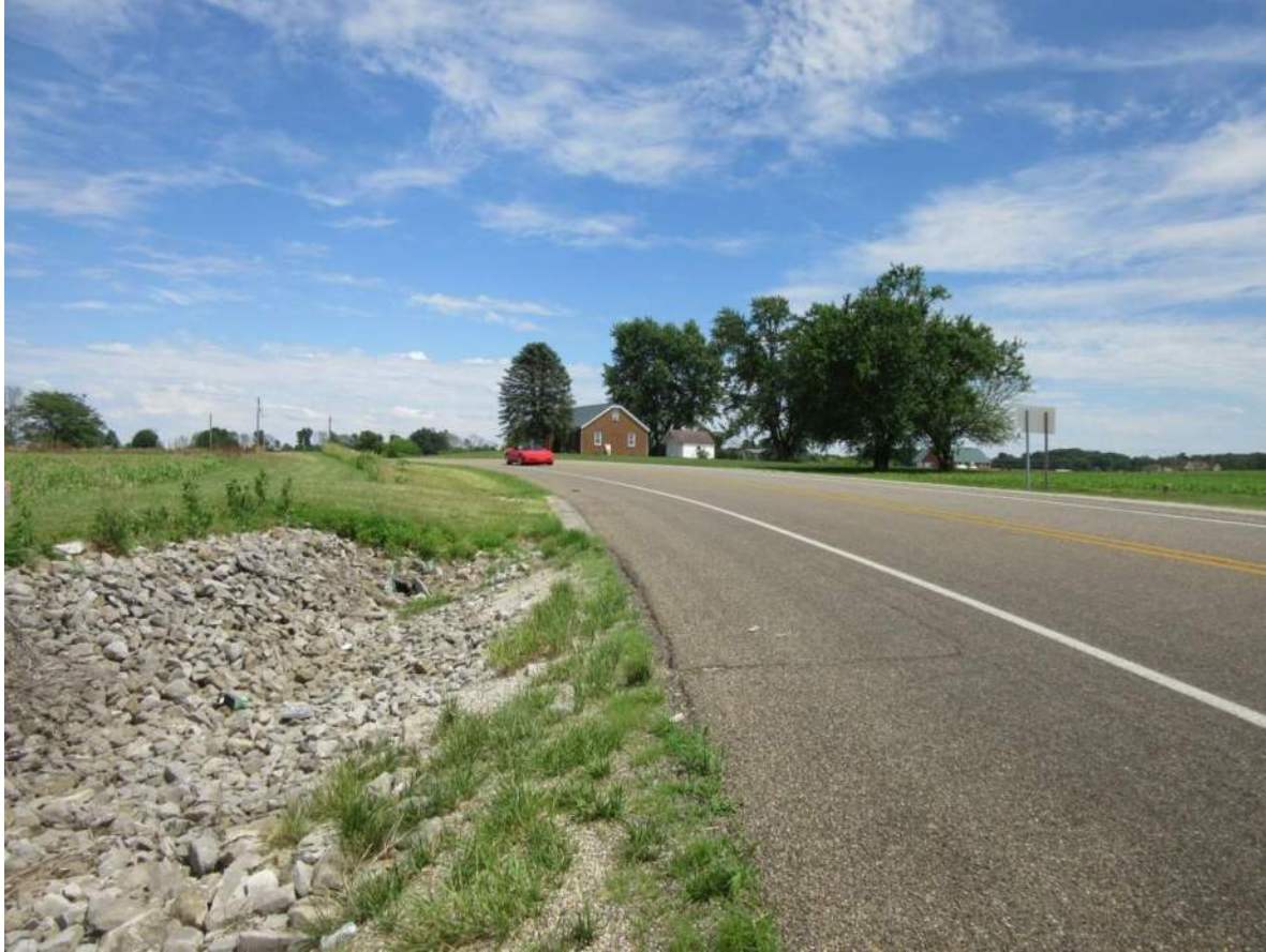
17. Looking southeast down the east side of SR 42. Photo taken 6/12/19.
