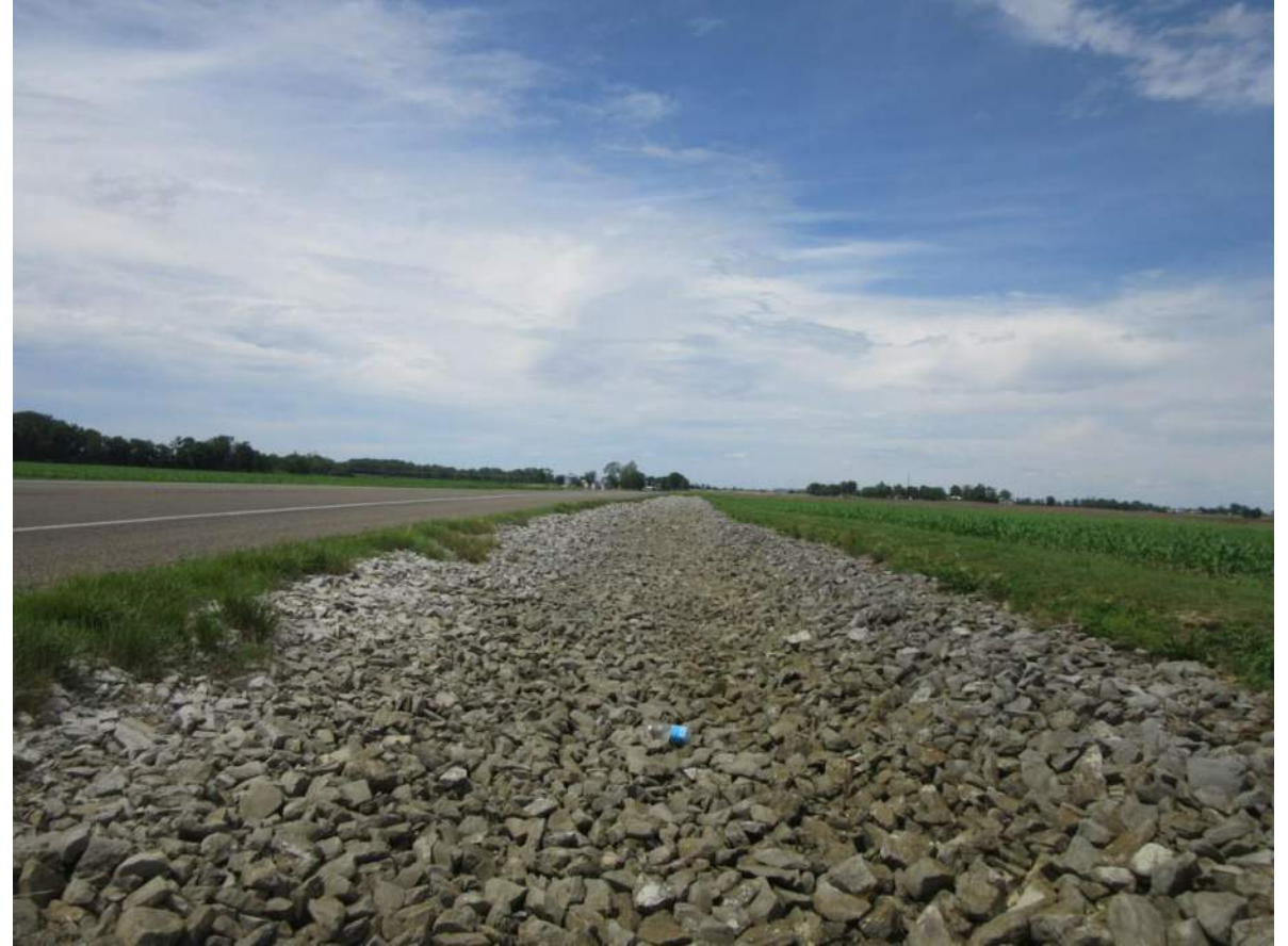
22. Looking north up ditch line on the east side of SR 42. Photo taken 6/12/19.
