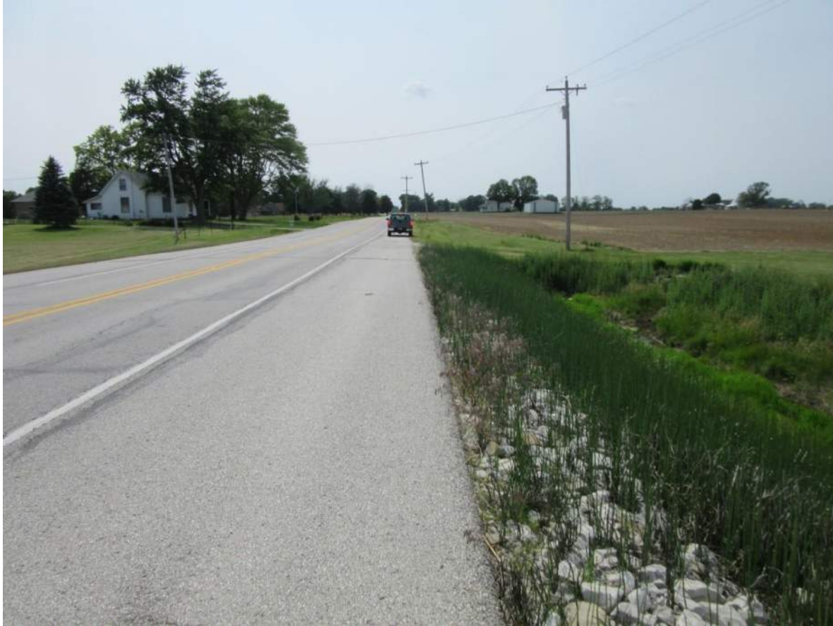
57. Looking west down SR 42 from the north side of roadway at Wetland D1 and UNT 6 to Lake Ditch. Photo taken 6/3/19.
