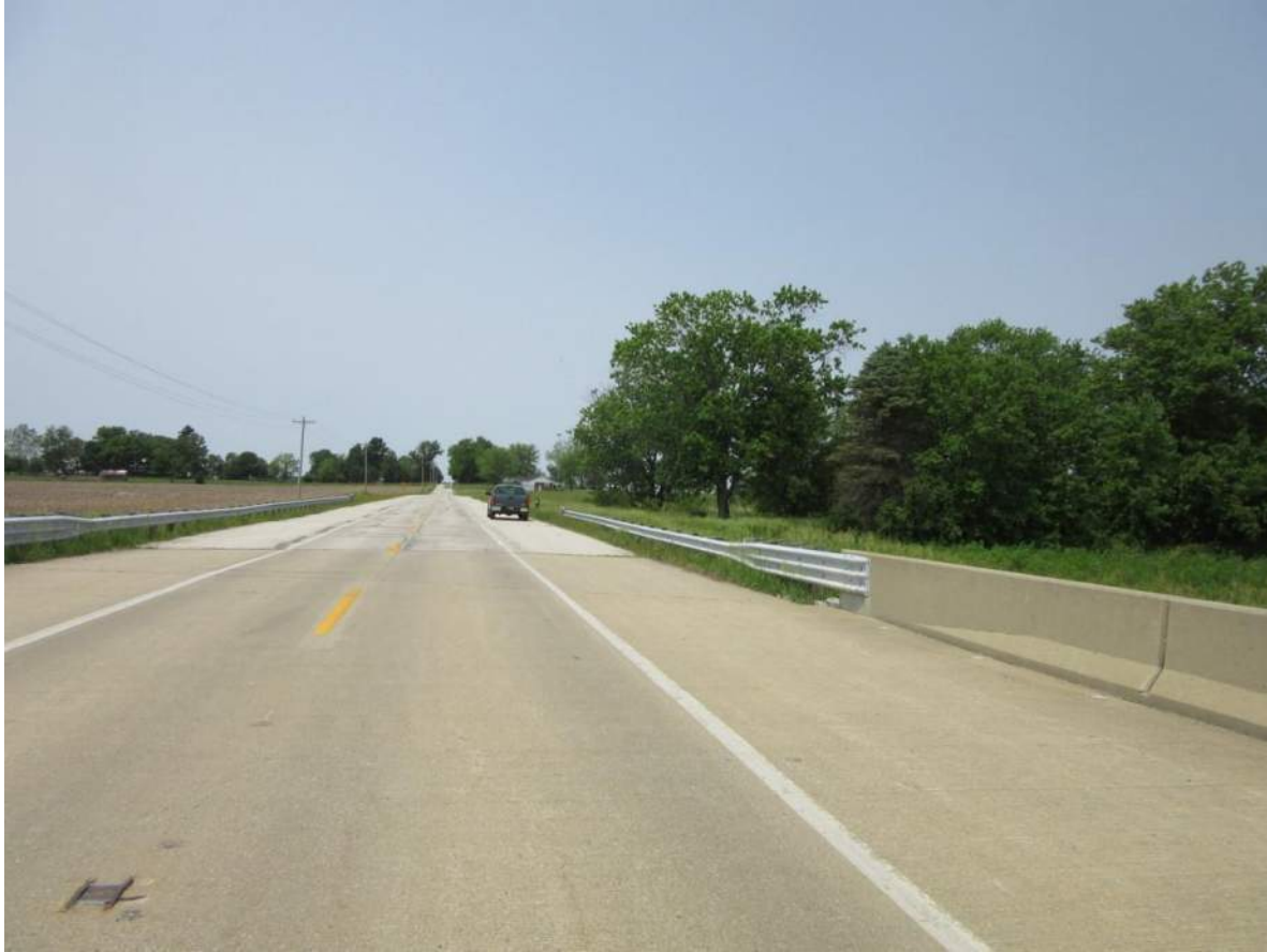
73. Looking west from bridge down SR 42. Photo taken 6/3/19.
