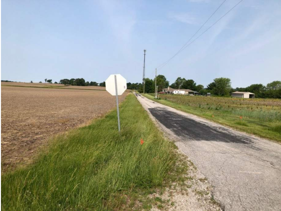
51. Intersection of SR 42, Simpson Rd., and Wellman Rd. looking west down Simpson Rd. Photo taken 6/4/19.
