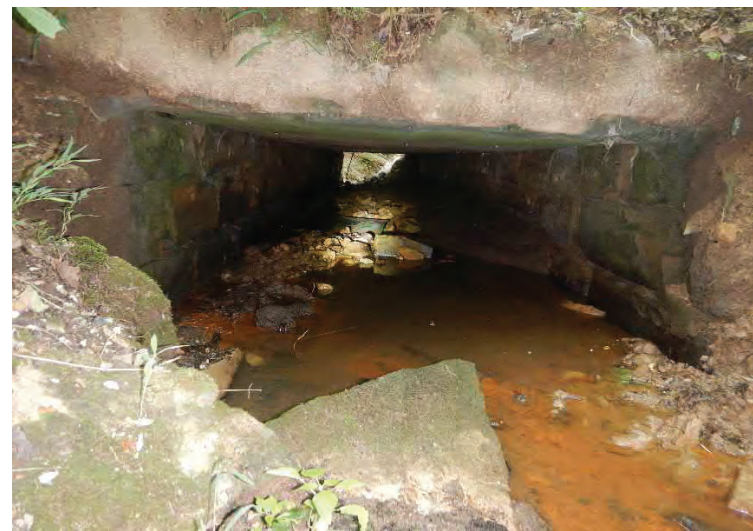
Photo 8- Inside structure, facing south
