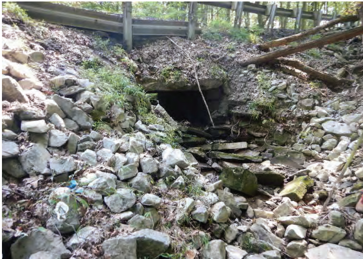
Photo 7- Pipe Inlet, north end of structure
