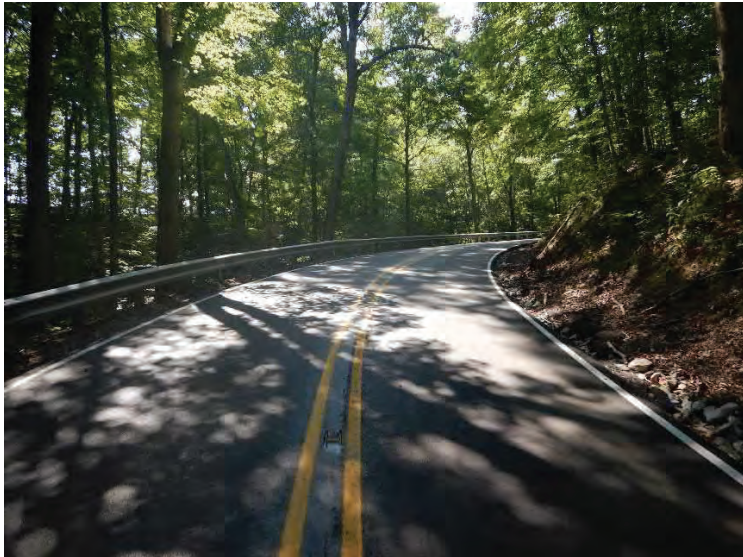
Photo 1- Northeast terminus, SR 58 facing east
