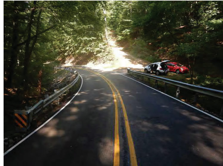
Photo 2- Northeast terminus, SR 58 facing west
