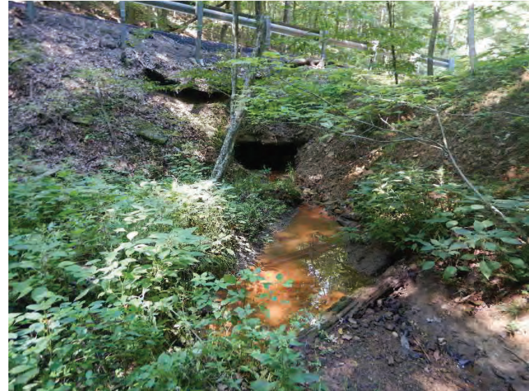
Photo 6- Pipe Outlet, south end of structure
