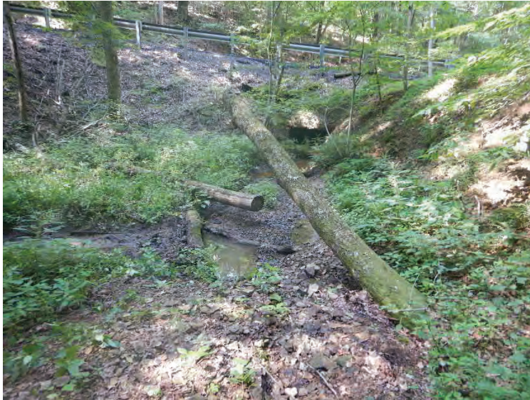
Photo 5- Ditch from south outlet facing north
