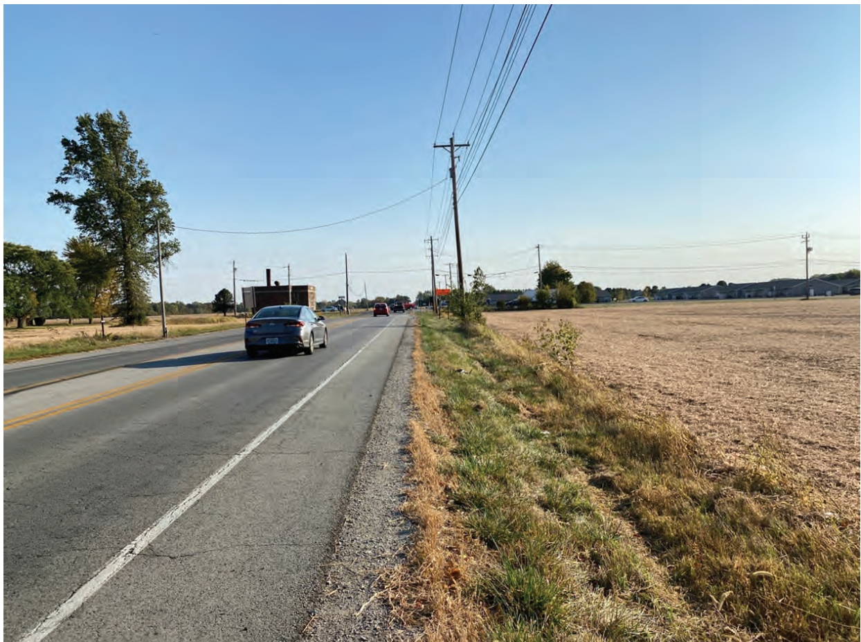
20. Looking south along SR 13
