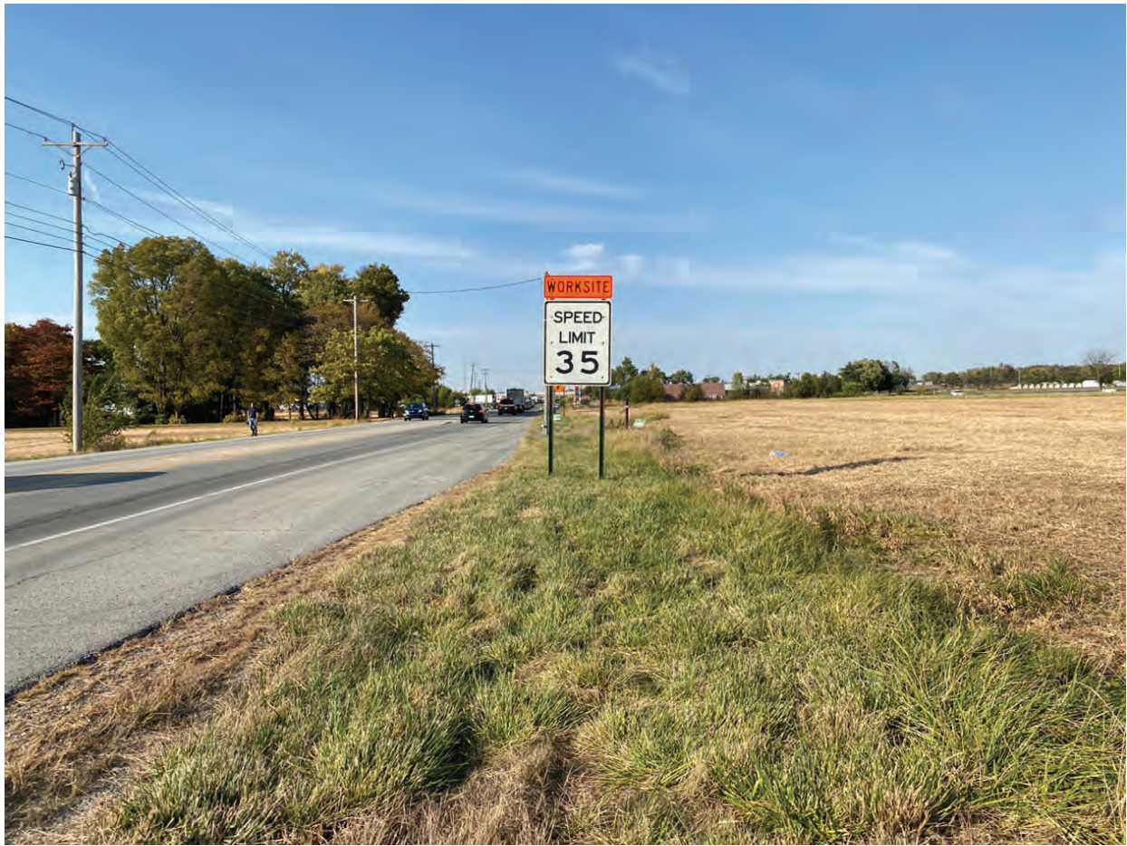
19. Looking north along SR 13
