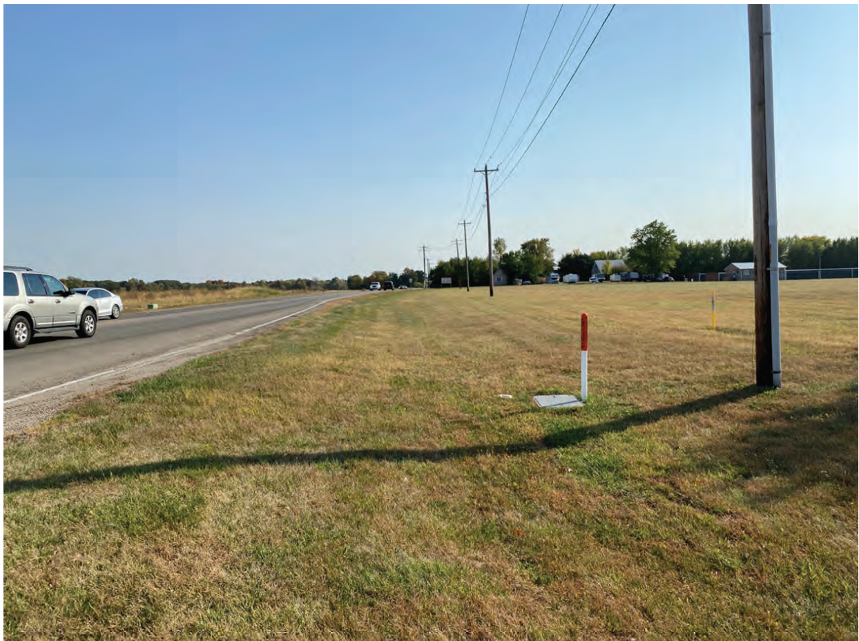
10. Looking south along SR 13
