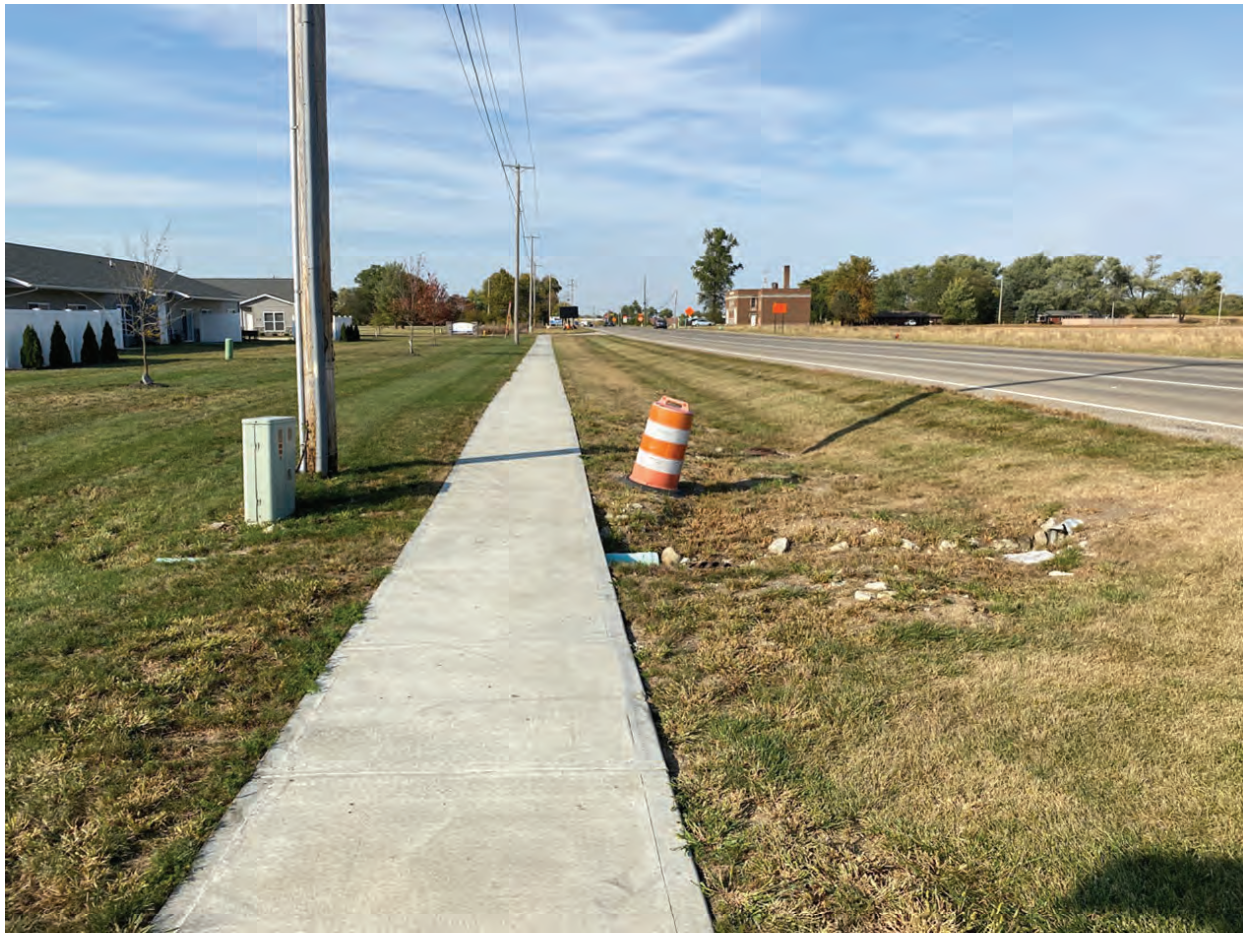
9. Looking north along SR 13, outside of the construction limits
