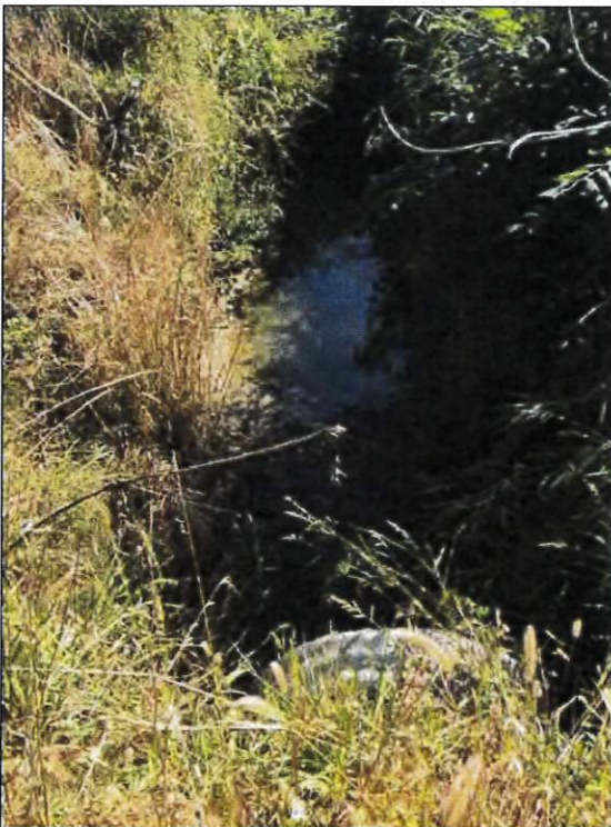
Picture 79— UNT2 to White Creek corrugated metal pipe inlet; east view; 9-23-22.
