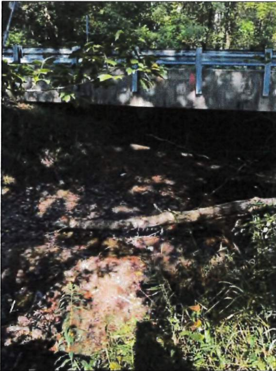
Picture 13—White Creek upstream and project structure 058-03-05882 B; northwest view; 9-23-22.
