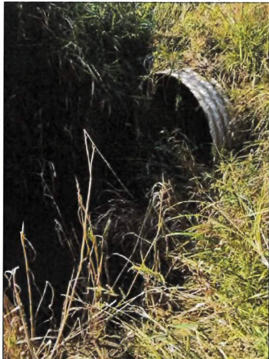
Picture 78—UNT2 to White Creek corrugated metal pipe inlet; southwest view; 9-23-22.
