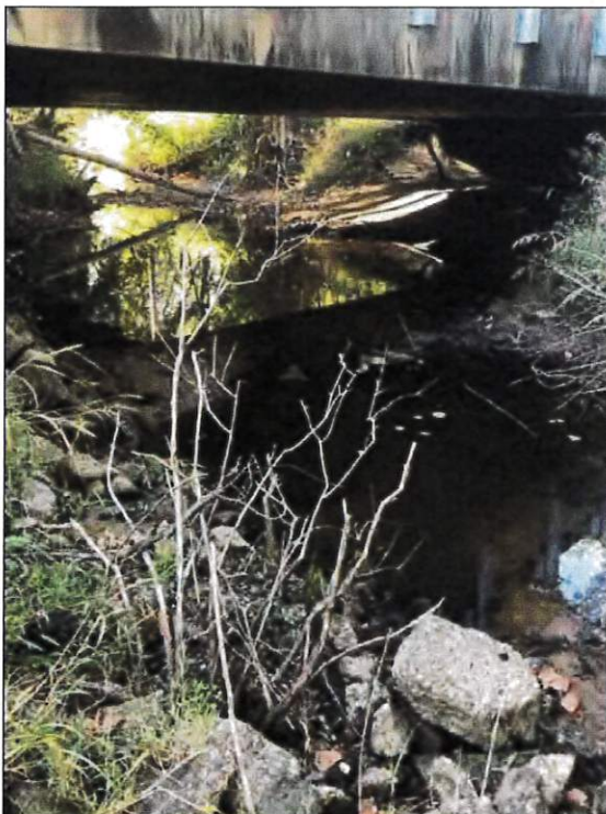
Picture 3—White Creek downstream and project structure 058-03-05882 B; south view; 9-23-22.
