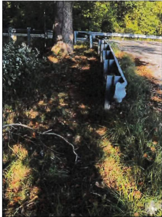
Picture 46—CR 700S roadside; northwest view; 9-23-22.
