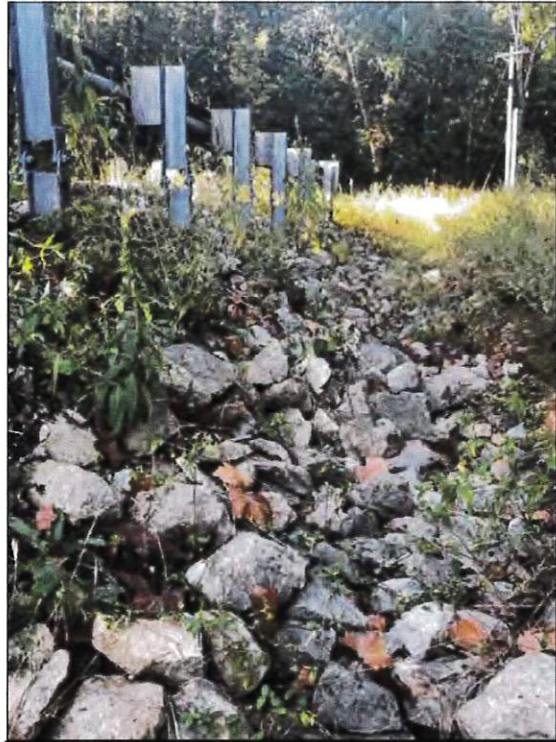
Picture 42—Riprap area; southwest view; 9-23-22.
