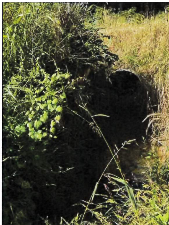
Picture 76—UNT2 to White Creek corrugated metal pipe inlet; west view; 9-23-22.
