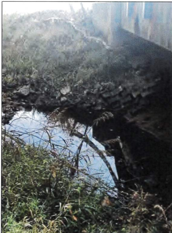
Picture 7—White Creek and project structure 058-03-05882 B; east view; 9-23-22.
