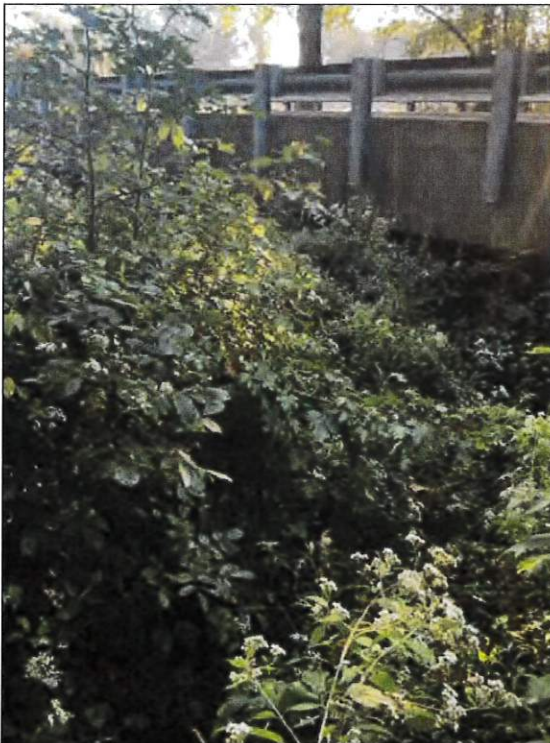
Picture 23—Project structure 058-03-05882 B from UNT1 to White Creek; east view; 9-23-22.
