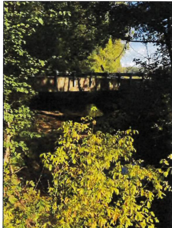
Picture 8—White Creek upstream and project structure 058-03-05882 B; north view; 9-23-22.
