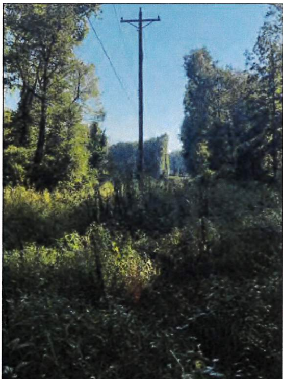
Picture 52—Powerline corridor east view; 9-23-22.
