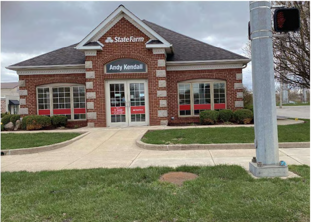
8 Looking south at c. 2002 commercial building at 333 W. Main Street
