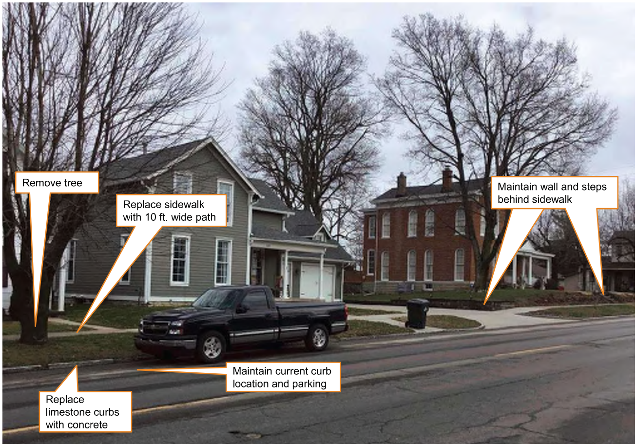
23 Looking northeast across SR 46 towards Wilder Street at “Contributing” and “Notable” houses in the Greensburg Eastside Residential Historic District.
