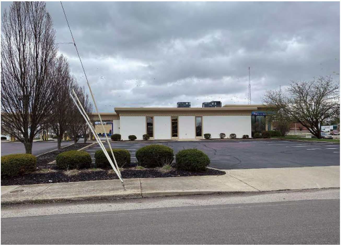
5 Looking east at the c. 1973 "Contributing" bank (RQAW #8) within the original APE.
