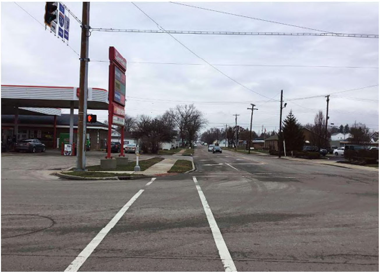
3 Looking north from the Main Street (SR 46) and US 421 (Ireland Street) intersection.
