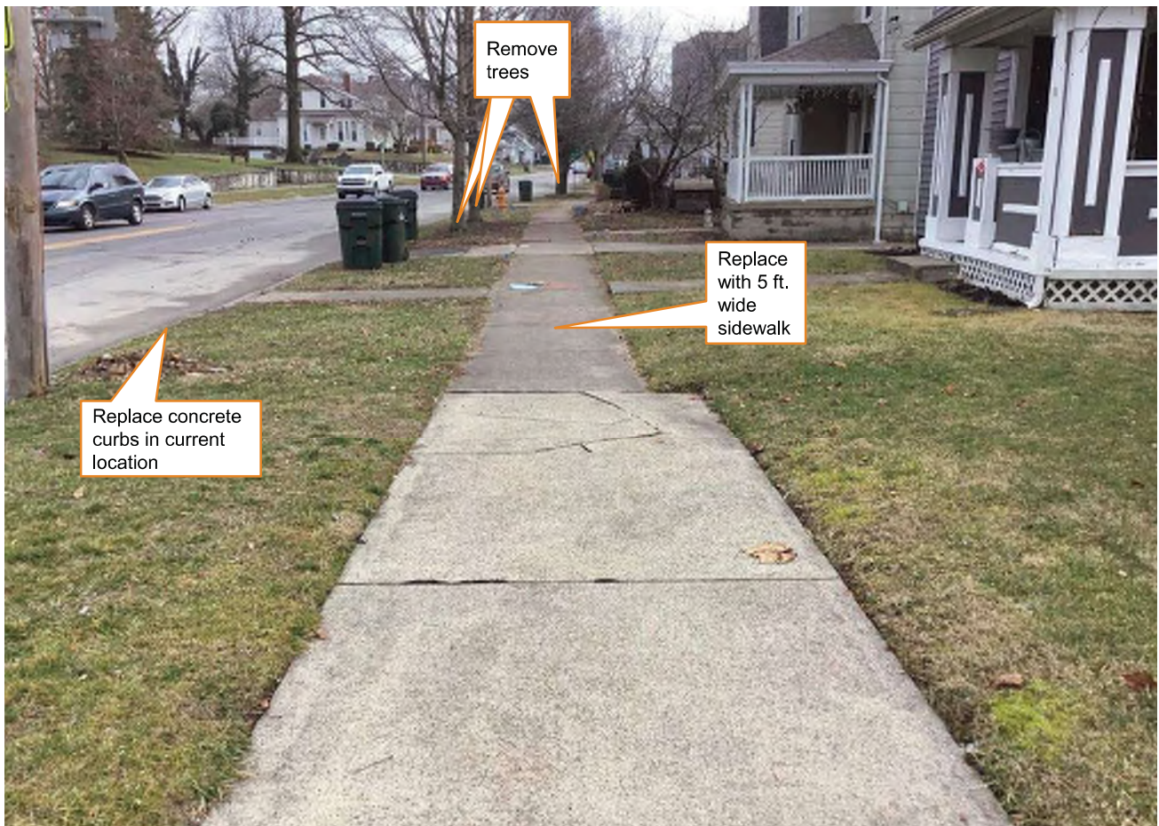
8 Looking east along the south side of SR 46 in the Greensburg Eastside Residential Historic District.
