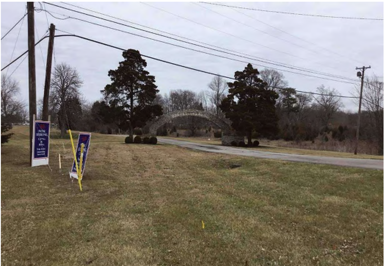
108. Looking northeast at the “Contributing” c. 1940 cobblestone veneer arch (RQAW # 16) at Arbor Grove Village, previously the Odd Fellows Home.
