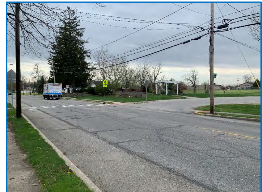
Photo 8 – View of the intersection of SR 22 and Jefferson Street, facing southwest. Memorial Park is in the background (04-22-20).
