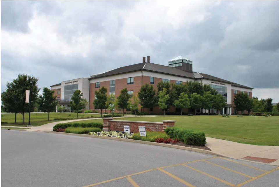
Photograph 15. View of large modern buildings on the campus of Taylor University, looking southwest.
