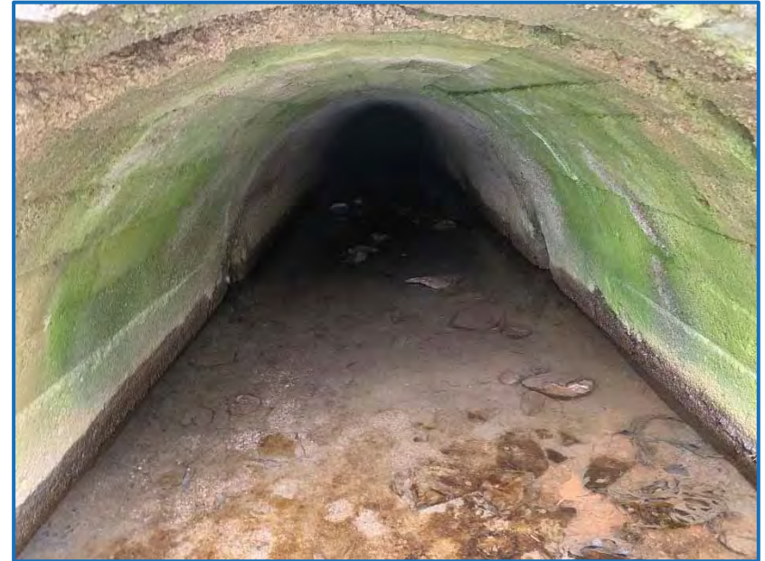
Photo 6 – View facing west inside of INDOT Structure No. CV 022-027-49.42 (4-23-2020).
