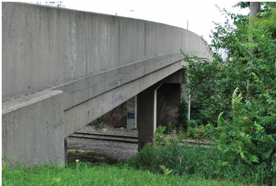
Photograph 6. SR 22 bridge over the CERA Railroad (Structure No. 22-27-02130A), looking southeast.
