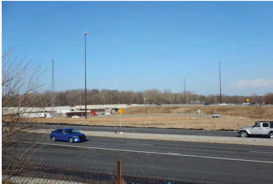
Photograph 7. View of the project area along the I-465 EB off-ramp to US 31/East Street NB, looking northeast. The US 31/East Street NB on-ramps to I-465 are higher in elevation than the area proposed for improvements.
