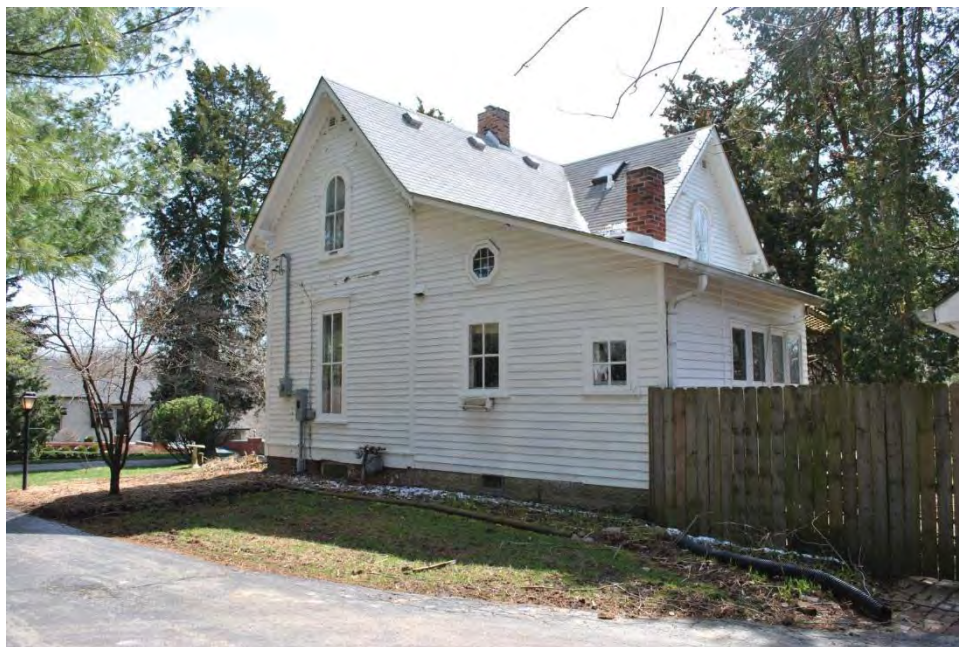
Photograph 2. View of the north side elevation of 4398 Asbury Street (IHSSI No. 097-392-85266), showing the later addition, looking southeast.
