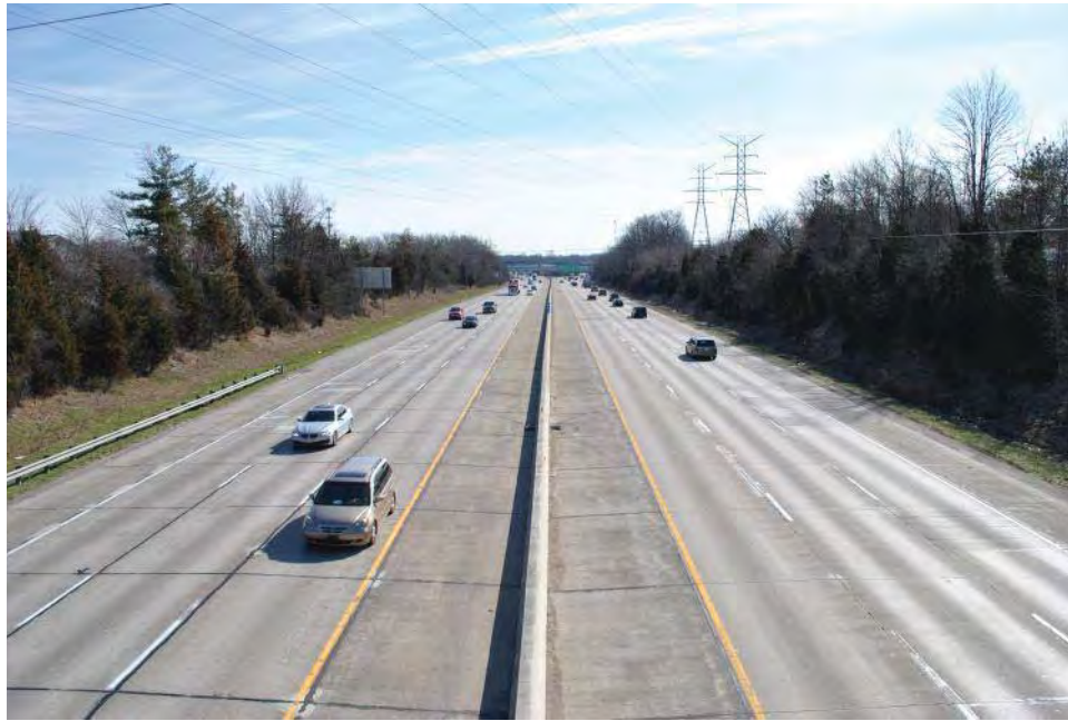
Photograph 11. View of the project area along I-465 from the Keystone Avenue bridge, looking east-northeast. The adjacent land use is predominantly mid-twentieth century single-family residences south of the interstate and modern multi-family residences north of the interstate.
