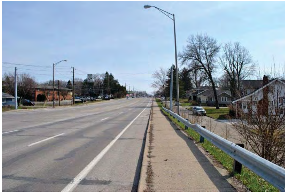
Photograph 9. View of the southern approach to the Madison Avenue bridge, looking south-southeast. The adjacent buildings are early and mid-twentieth century residences.
