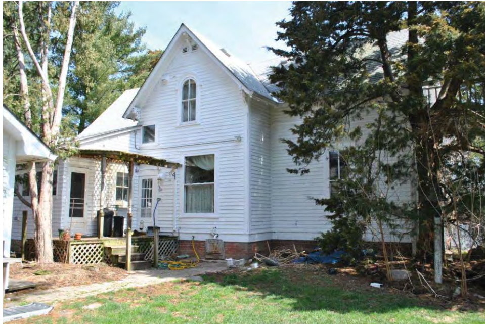
Photograph 3. View of the rear (west) elevation of 4398 Asbury Street (IHSSI No. 097-392-85266), looking northeast.
