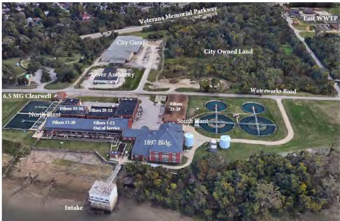
Figure 3 – View of Evansville's existing water treatment plant looking east with the City garage, the proposed site of the new plant, in the upper left. This pre 2019 photo does not show the Waterworks Road relocation across the wooded City owned land.
